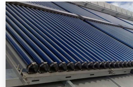
Example of Solar Thermal unit
