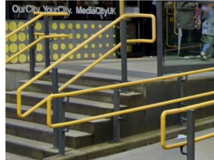
H01 - Steel Handrail
