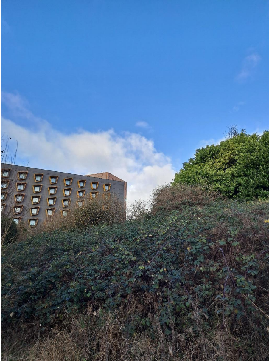
Figure 3: Dense Scrub North of the Site
