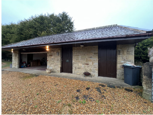
View of the existing detached garage
