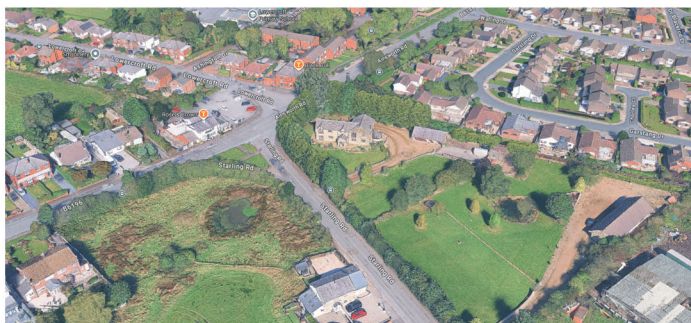
Aerial view of the site and surroundings.
