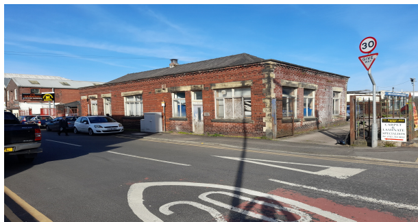
View of building from Stewart Street/Tottington Road junction.
