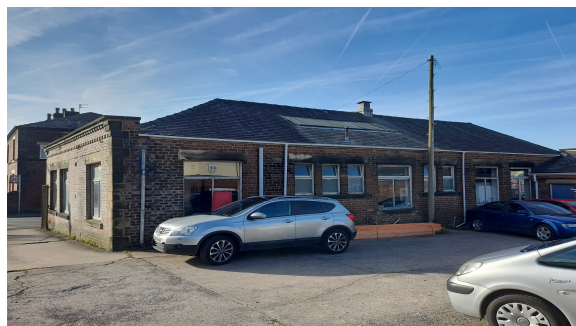
View of rear elevation
