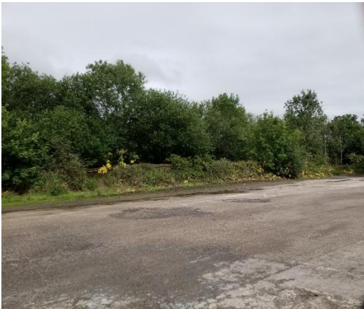
Image 4.24: Area of hardstanding within northern area of Scheme footprint
