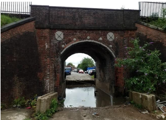
Image 4.19: Underpass beneath railway line
