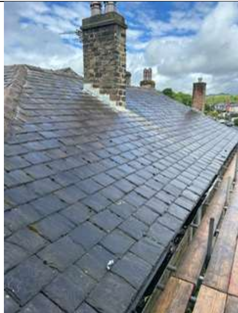
North facing view across roof slope D.
