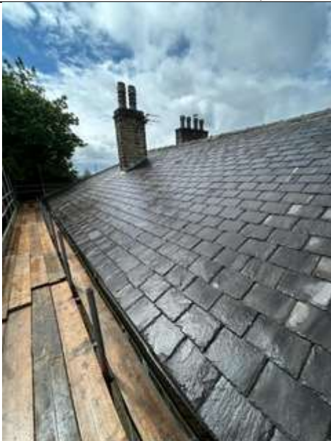
South facing view across roof slope D.
