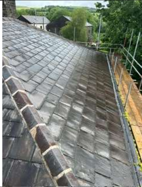
View across roof slope F.
