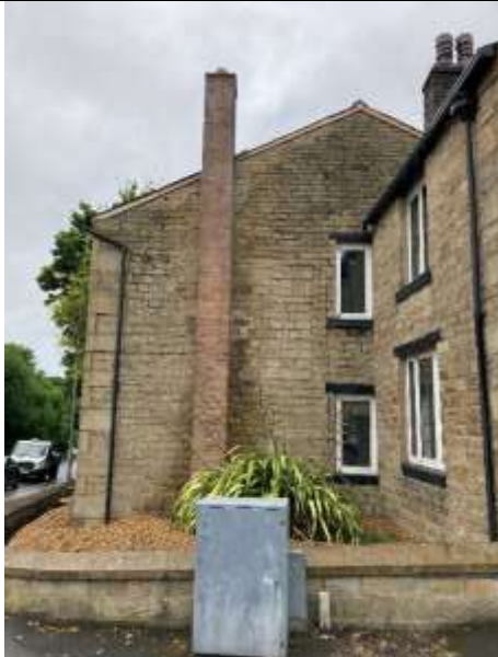
North gable with central brick chimney stack.
