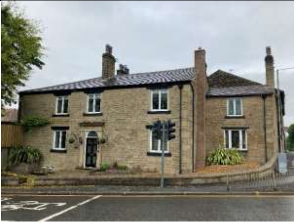
East elevation to Walmersley Road, including traditional slated roof surfaces and painted timber fascia boards to eaves.
