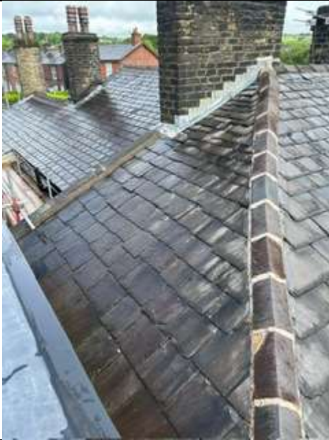
View across roof slopes E, C and A indicating Welsh slates, clay ridge and hip tiles, stone coping to verge and leadwork to stone chimney stacks.
