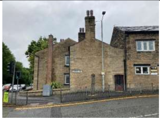
North elevation to Springside Road, with mortar bedded verges and chimney stacks.
