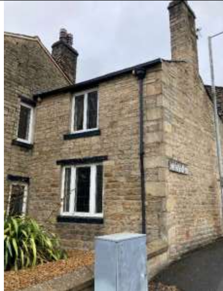
East elevation to north extension.
