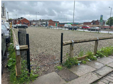
Photograph of the new pedestrian access for the car park
