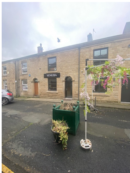
View of front elevation from opposite side of Square Street
