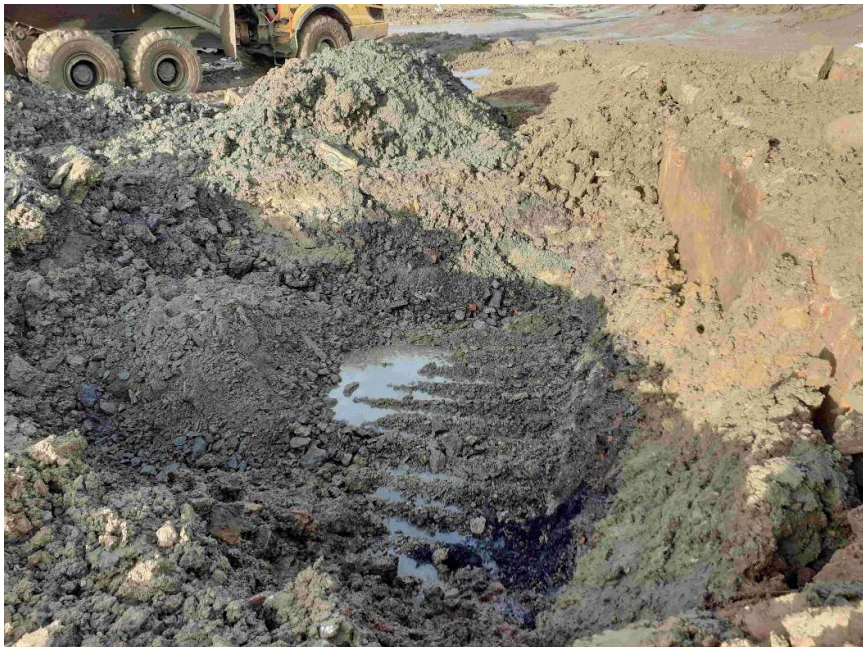
General view west over HS10-Cell 2 – excavation continued to competent Rough Rock Strata where ingress groundwater commenced
