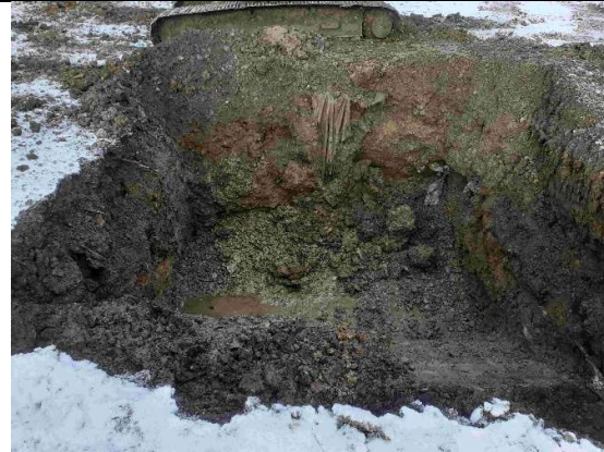
Initial dig in south side
