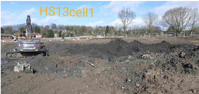
General view after excavation
