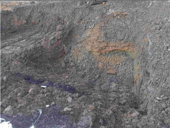
Second dig in north side (south backfilled with clean overburden)
