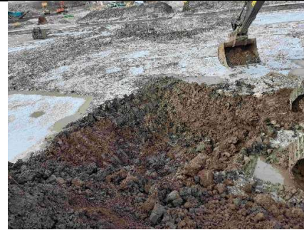
Commencement Excavation in south – temporary removal clean overburden
