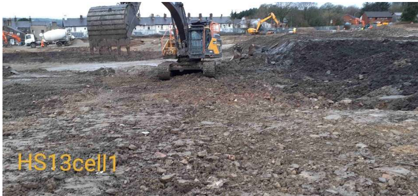
General view before excavation
