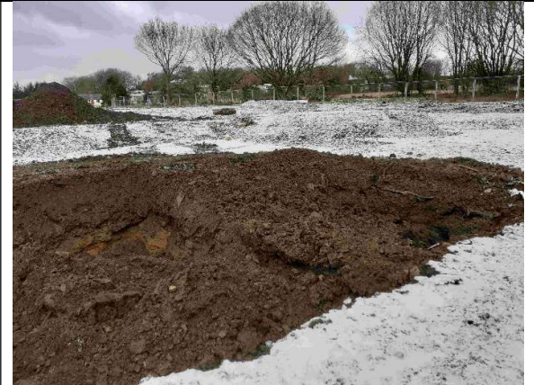
Extent of excavation
