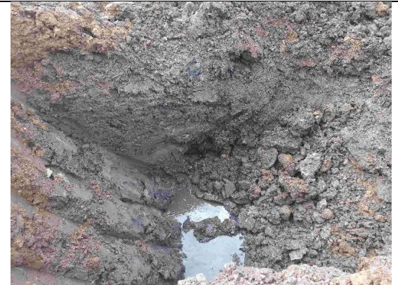
Base of excavation at 2.5-3.0m
