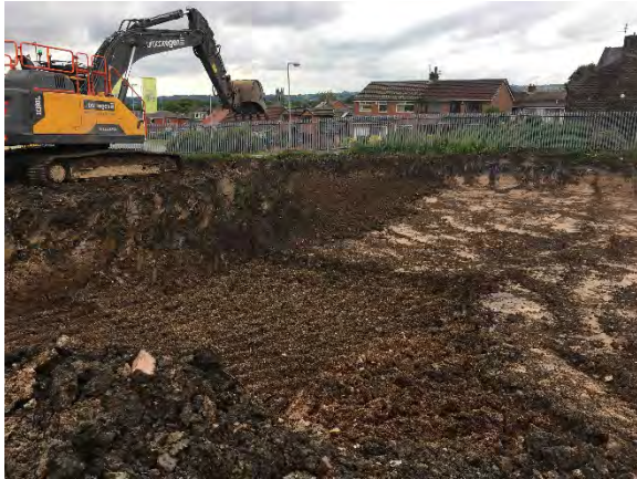
06.08.20 – Regrade of site levels in west (3/3)
