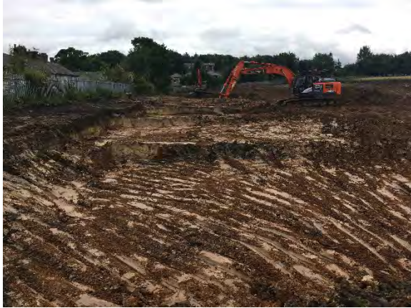
06.08.20 – Regrade of site levels in west (1/3)
