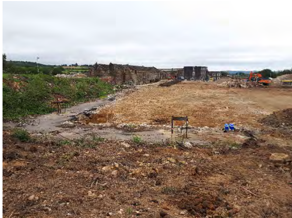
16.07.20 – View south from north of site: breakout of 'Building 2' slab visible in far distance.
