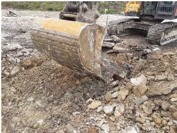
02.07.20 – Excavation of 'HS12' hotspot.
