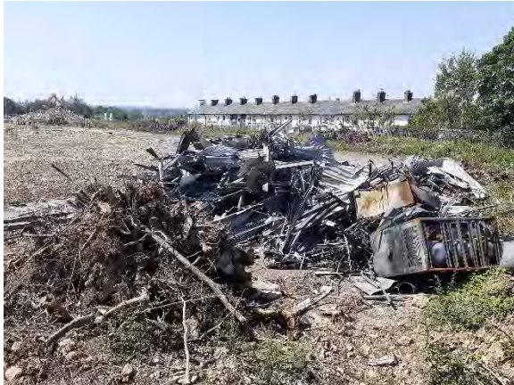
25.06.20 – Remnants of demolished 'Building 3' and small vegetation stockpile in north of site.
