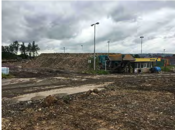
31.07.20 – Stockpile of crushed aggregate in wider Phase 1 area to south; feedstock recovered during Phase 1a earthworks (i.e. building slabs).
