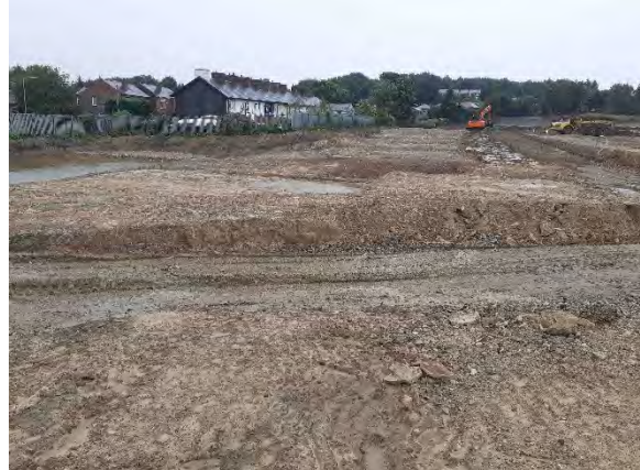
02.09.20 – Site recovered aggregate placed in footprints of future dwellings for use as development platforms in west.
