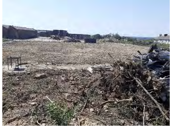
25.06.20 – View south from north of site: slab of 'Building 3' broken out and transferred to stockpile in wider Phase 1 area prior to inspection.
