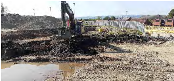
21.09.20 – Regrade of site levels in south (1/2).
