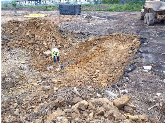
16.07.20 – Excavation of 'HS15' hotspot complete.
