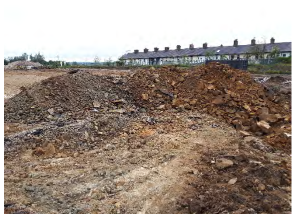
16.07.20 – 'HS15' hotspot excavation arisings.
