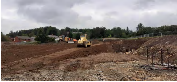
17.08.20 – Regrade of site levels in north (visible in far distance) and compaction of relocated soils.
