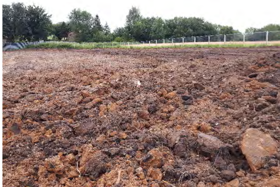
16.07.20 – Excavation and replacement of made ground soils complete in north (1/2).
