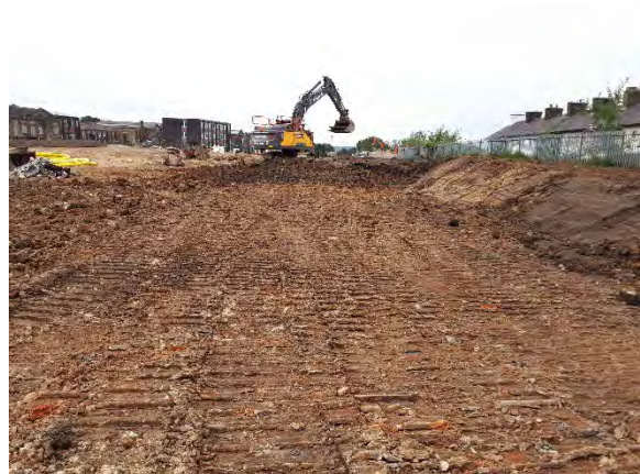
22.07.20 – Excavation and replacement of made ground soils along western boundary.
