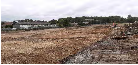
10.09.20 – Regrade of site levels in centre-northeast (visible in far distance).
