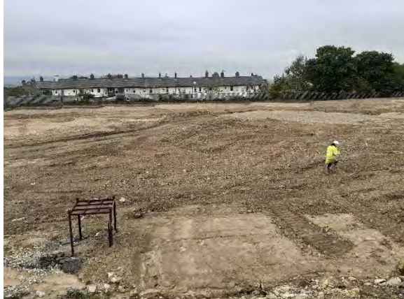
28.09.20 – Remediation works complete in central areas: view west from centre of eastern boundary.
