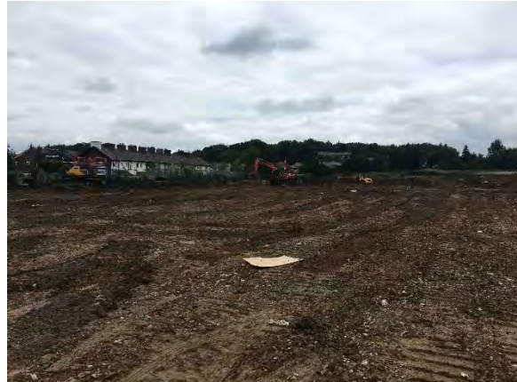
06.08.20 – Excavation and replacement of made ground soils complete in central areas of site.
