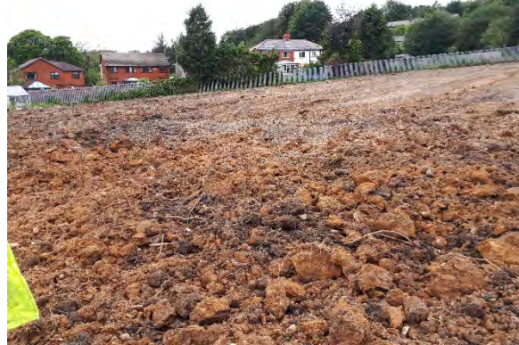
16.07.20 – Excavation and replacement of made ground soils complete in north (2/2).
