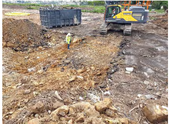
16.07.20 – Excavation of 'HS15' hotspot (2/2).
