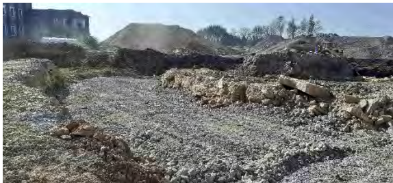
21.09.20 – Site recovered aggregate placed as road base along roadways in east.
