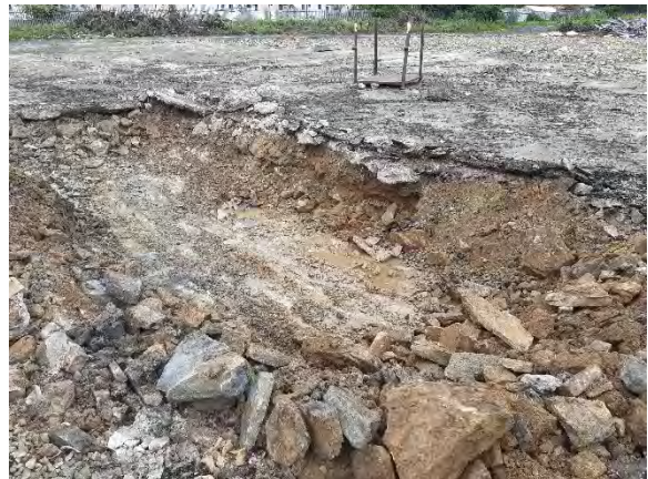
02.07.20 – Excavation of 'HS12' hotspot complete (1/2 - view west)
