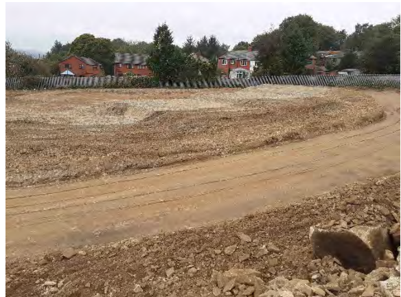
28.09.20 – Remediation works complete in north: view west from northeast of site
