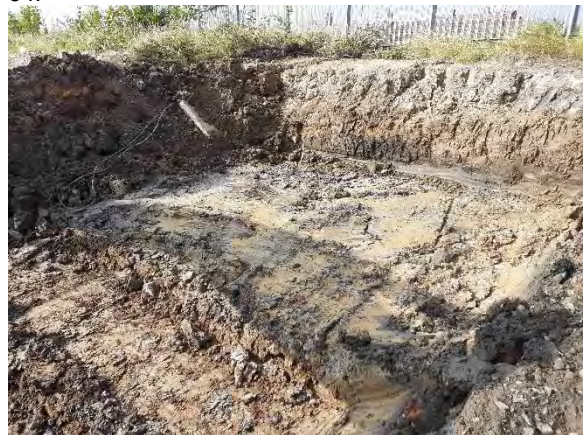
16.09.20 – Regrade of site levels in southwest (3/3).
