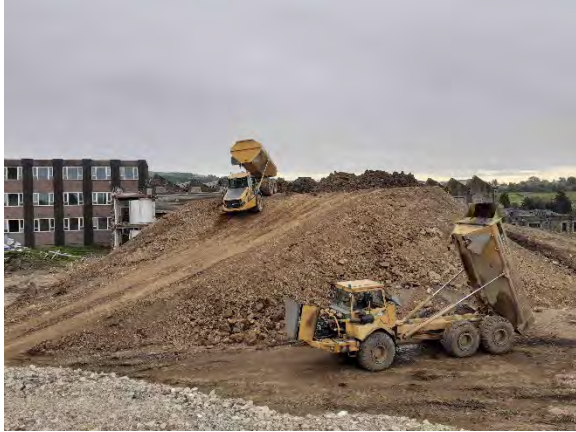
28.09.20 – Removal of excess soils from southeast to stockpile in wider Phase 1 area to south (2/2).
