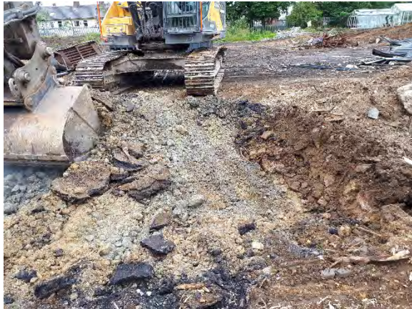
16.07.20 – Excavation of 'HS15' hotspot (1/2).
