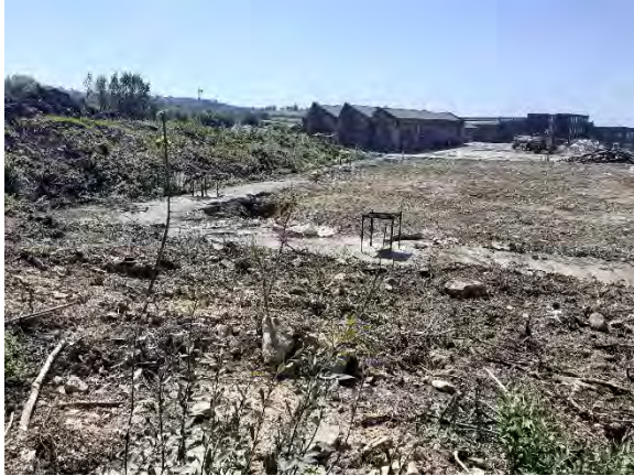
25.06.20 – View south-southeast from north of site: slab of 'Building 3' broken out and transferred to stockpile in wider Phase 1 area prior to inspection.
