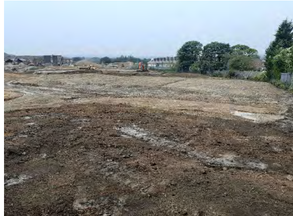
02.09.20 – Site recovered aggregate placed in footprints of future dwellings for use as development platforms in north.
