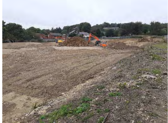
28.09.20 – Remediation works complete in central areas: view northwest from centre of eastern boundary (civil engineering works ongoing).
