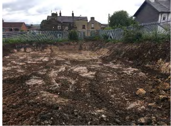
06.08.20 – Regrade of site levels in west (2/3)
