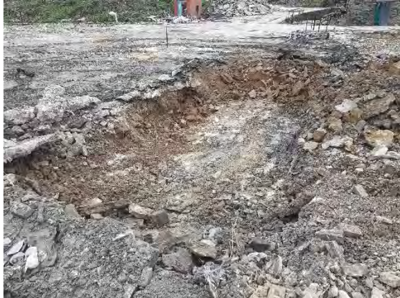
02.07.20 – Excavation of 'HS12' hotspot complete (2/2 - view east).
