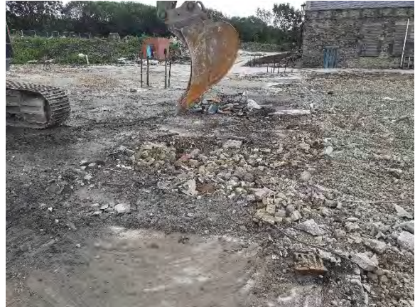
02.07.20 – Location of 'HS12' hotspot prior to excavation works.
