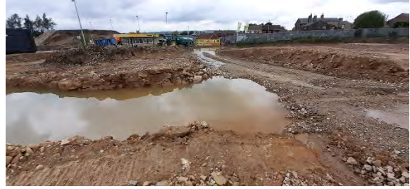
27.08.20 – Pumping of flooded areas in south of site using tractor and bowser (1/2 - view west).
