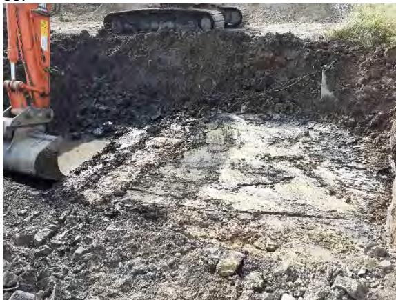
16.09.20 – Regrade of site levels in southwest (2/3).
