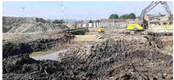
21.09.20 – Regrade of site levels in south (2/2).
