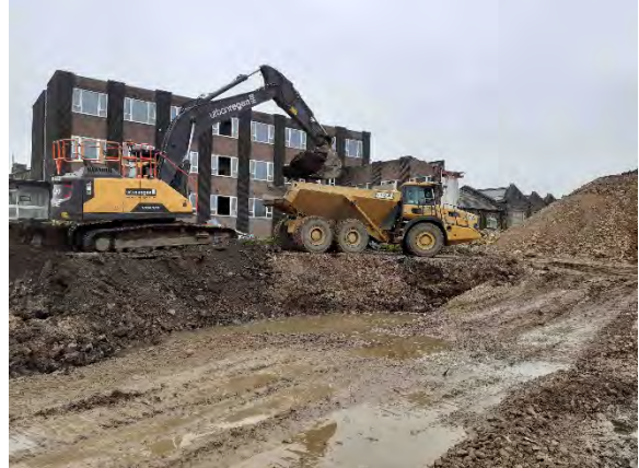
28.09.20 – Removal of excess soils from southeast to stockpile in wider Phase 1 area to south (1/2).
