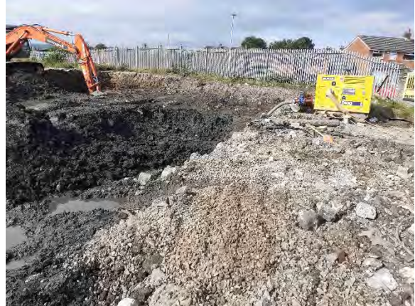
16.09.20 – Regrade of site levels in southwest (1/3).
