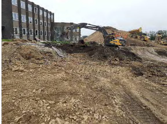
28.09.20 – Regrade of site levels in southeast (1/2).
