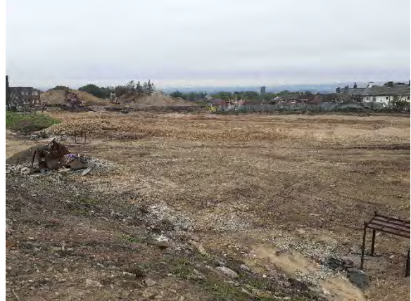
28.09.20 – Remediation works complete in central areas: view southwest from centre of eastern boundary.
