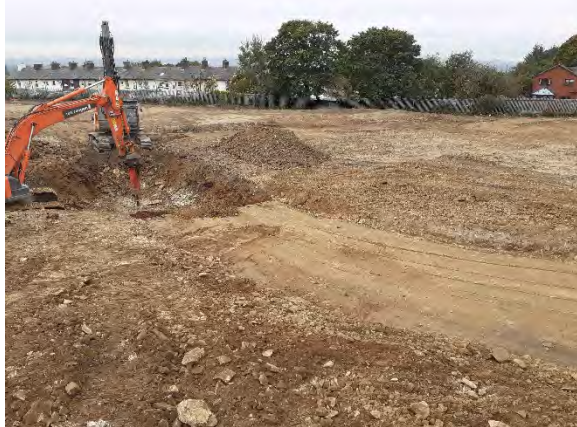
28.09.20 – Remediation works complete in central areas: view southwest from northeast of site (civil engineering works ongoing).
