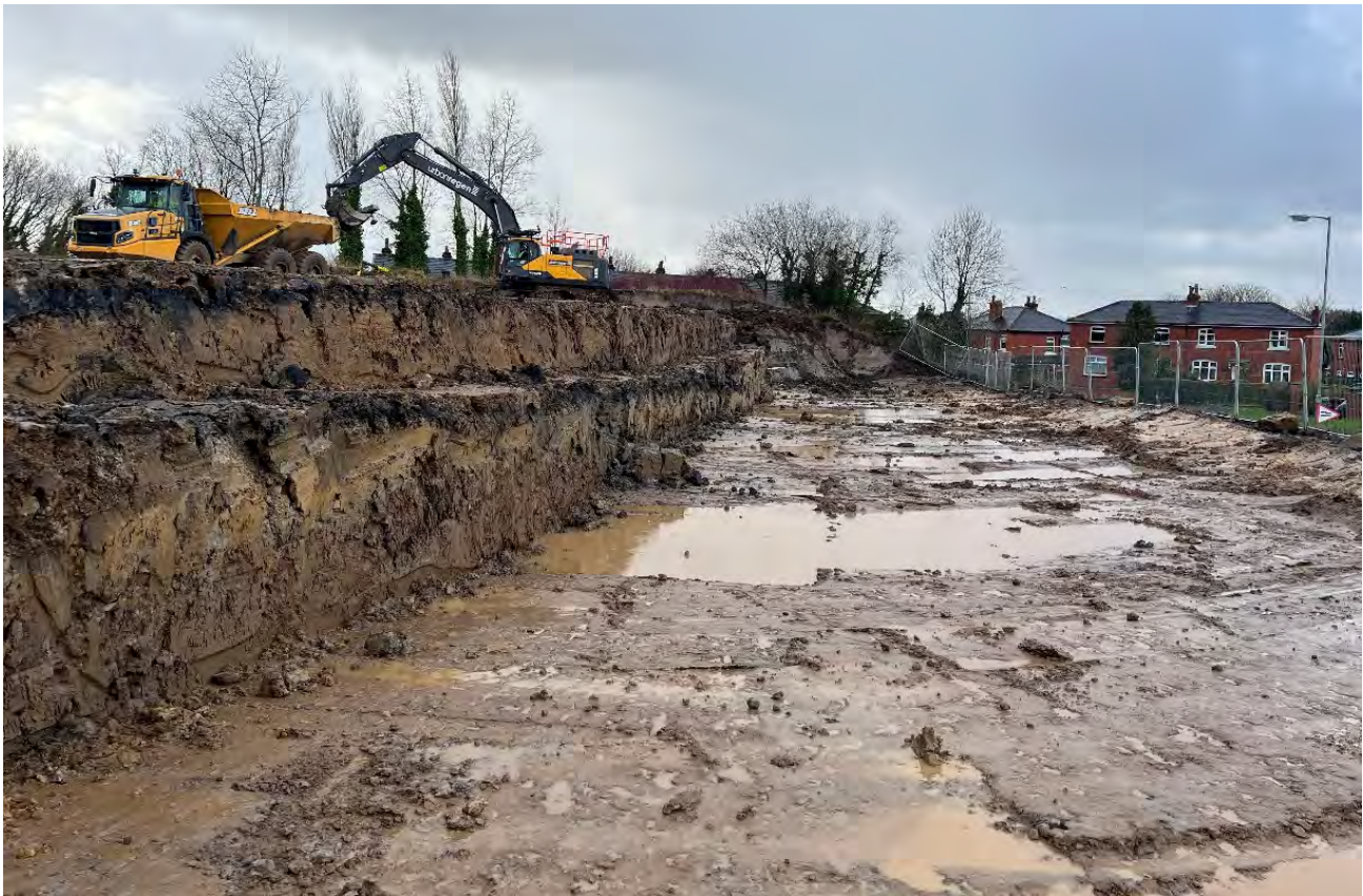
Photograph 7 – Progress of reduced level dig.
