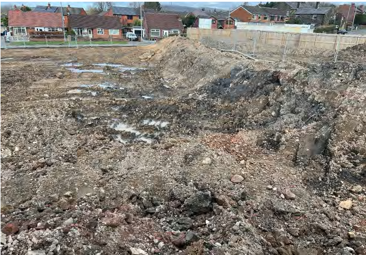
Photograph 13 – Northern extent of reduced level dig including area of hydrocarbon contamination.
