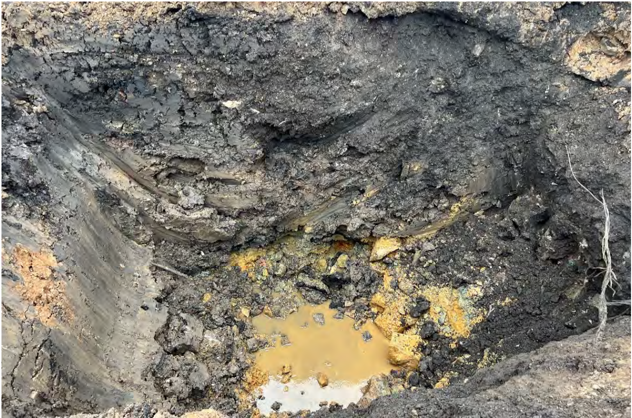
Photograph 26 – Area of deep Made Ground in northern extent of site (to be excavated to formation level)
