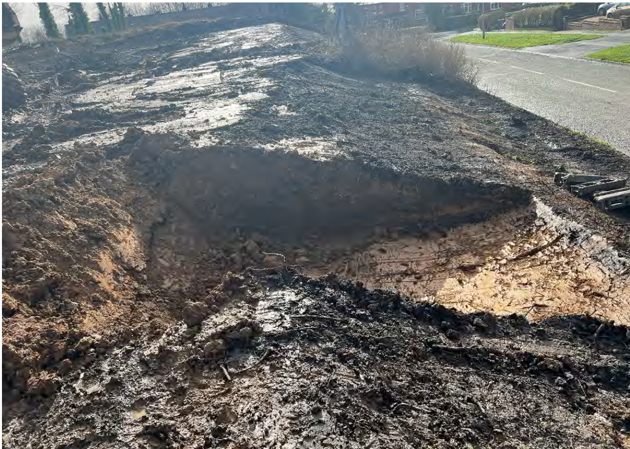
Photograph 5 – Excavation into reworked clay at western extent.
