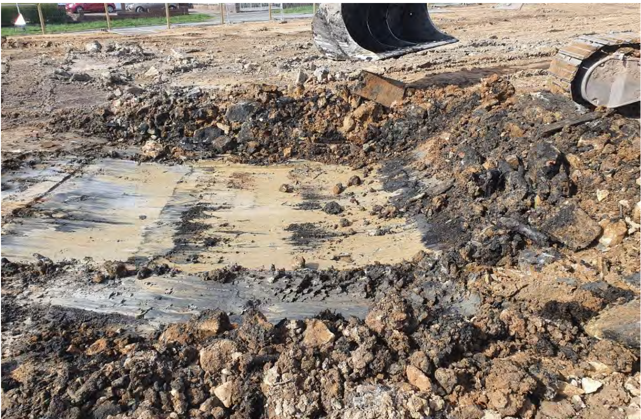
Photograph 21 – Natural (possibly reworked) clay beneath containing some bands of silt (black material)
