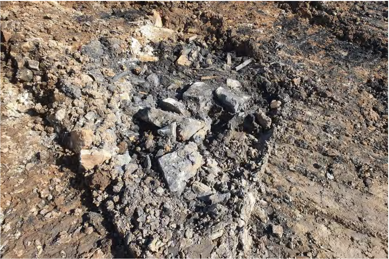
Photograph 22 – Made Ground present at proposed formation level.
