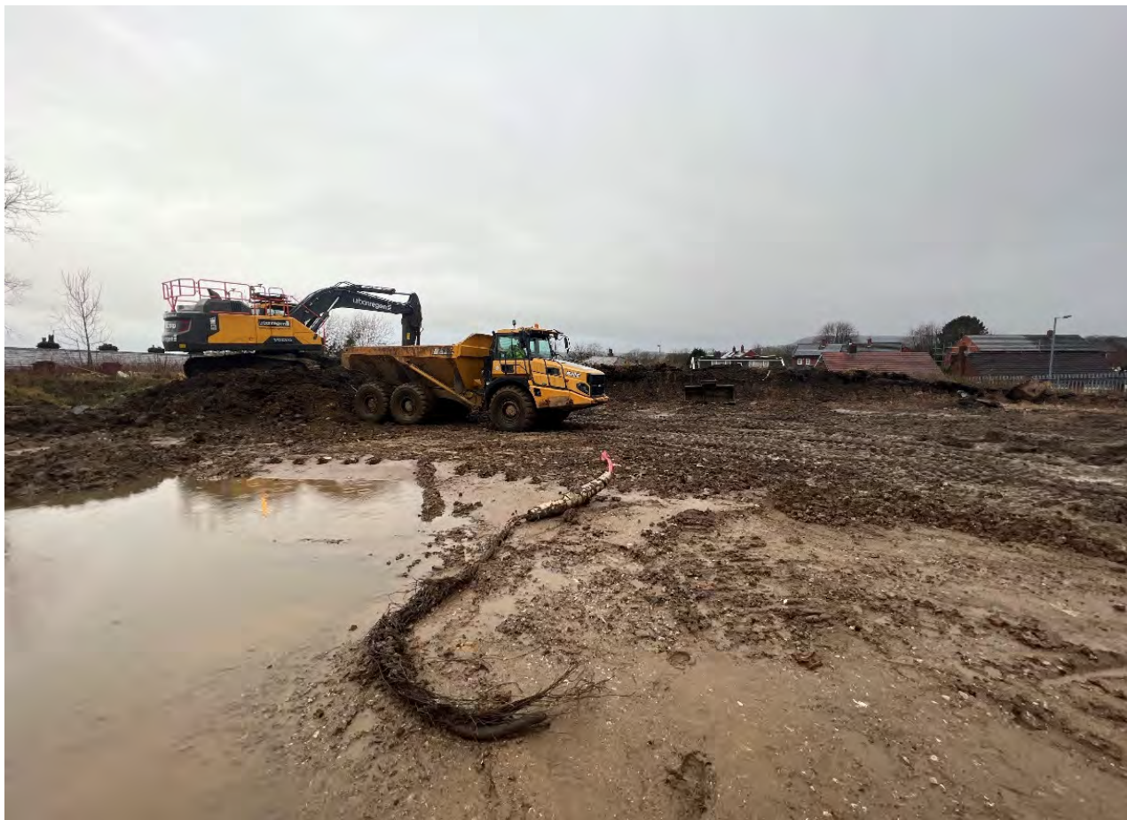
Photograph 3 – Stockpile/vegetation clearance at former car park area.
