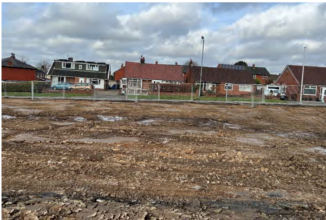
Photograph 15 – Western site boundary with soils at near proposed formation level, some small areas of Made Ground still present at surface level.
