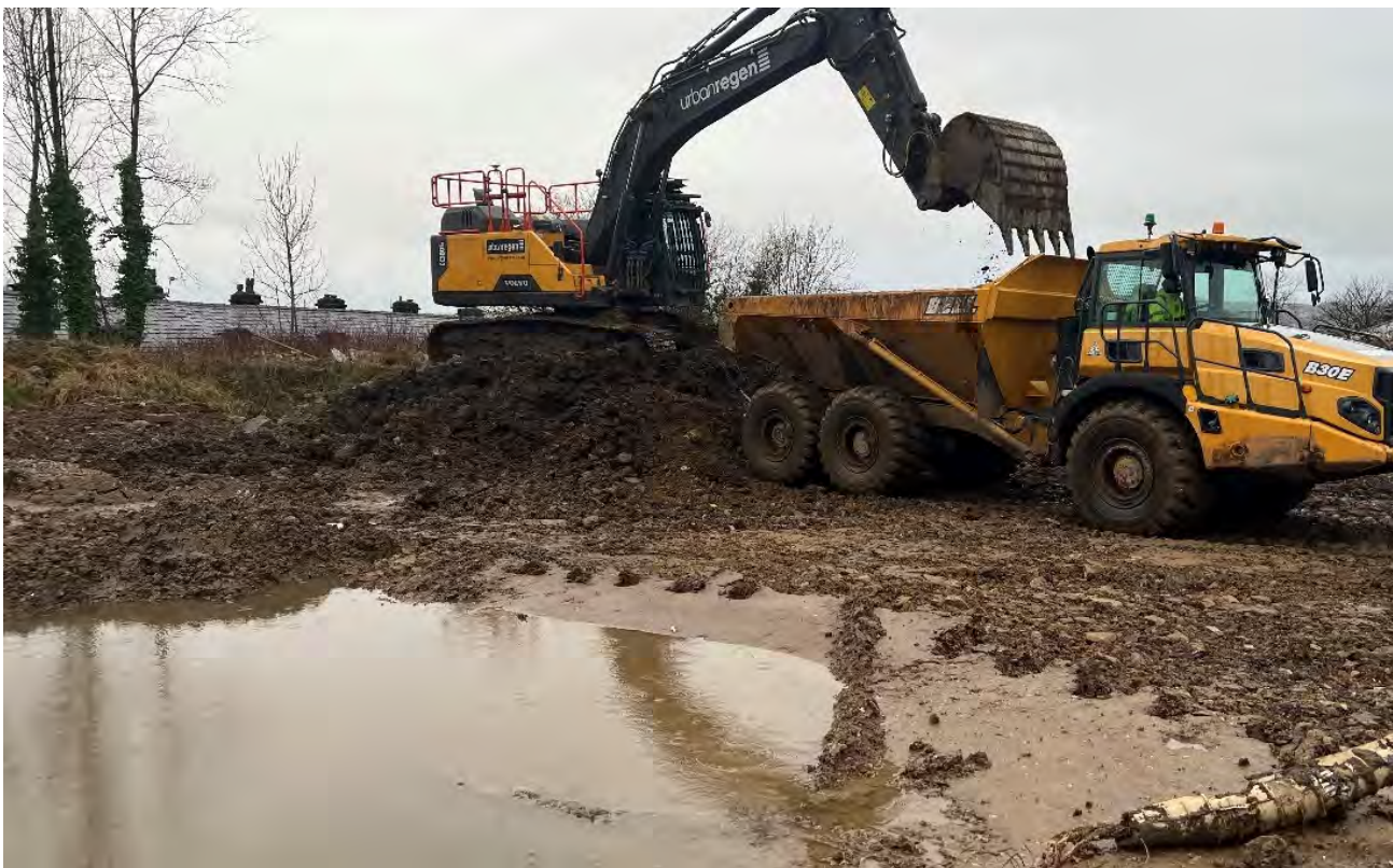
Photograph 2 – Stockpile/vegetation clearance at former car park area.
