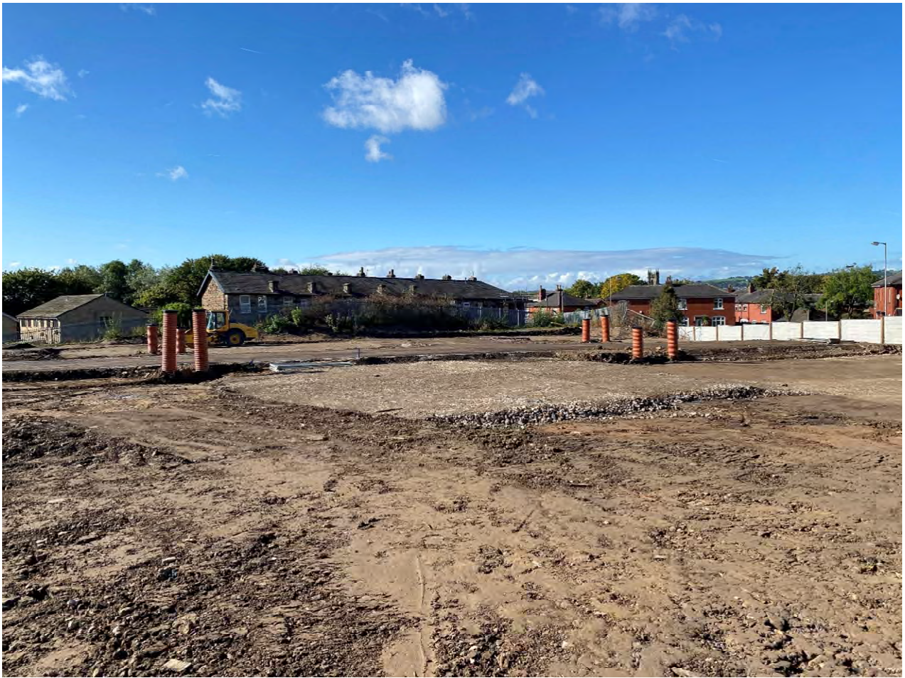
Photograph 36 – Roadway at centre of site and imported 6F2 material (piling mat) beneath.
