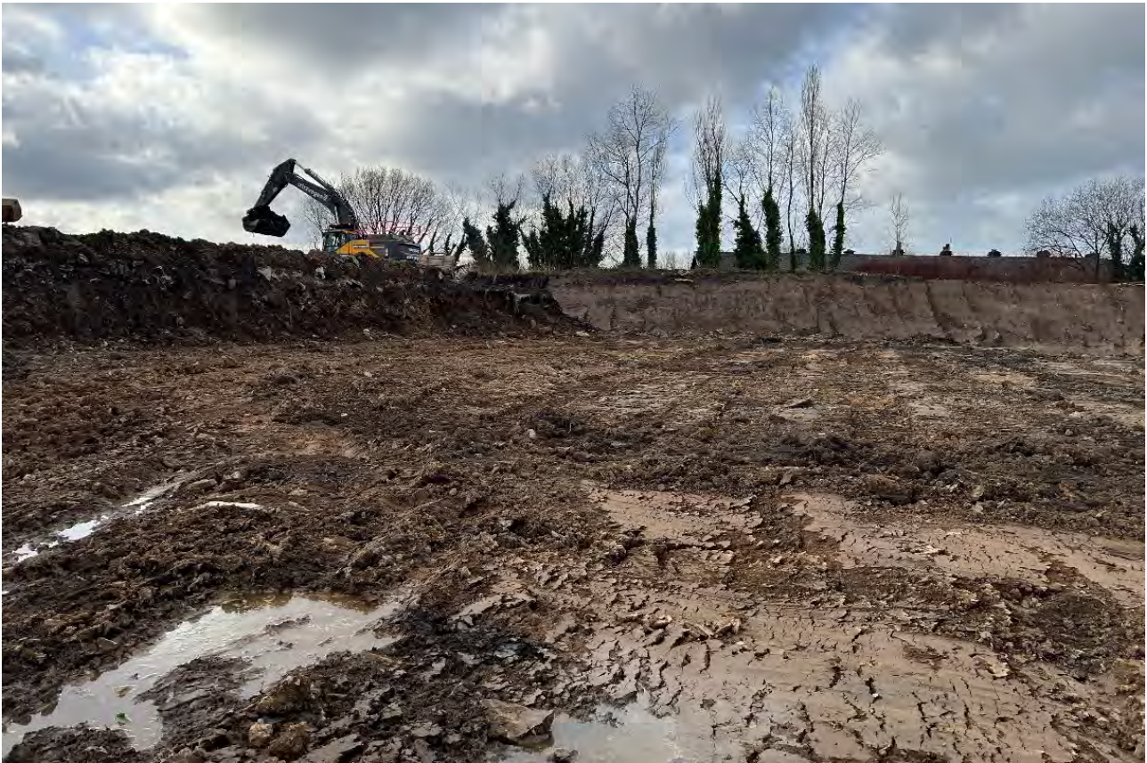
Photograph 14 – Natural clay present at formation level (possibly reworked).
