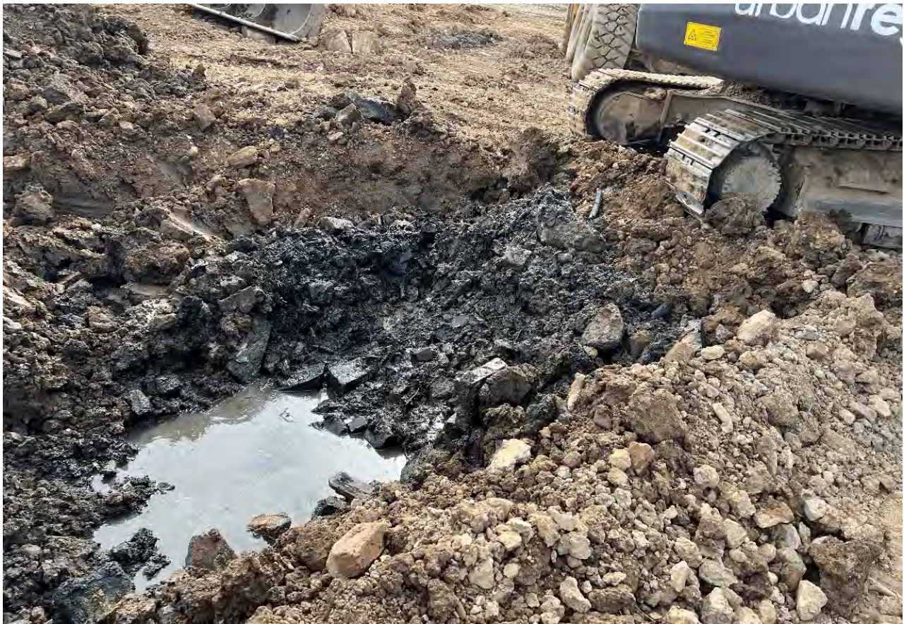
Photograph 35 – Deeper Made Ground removed from ground along the northern boundary.
