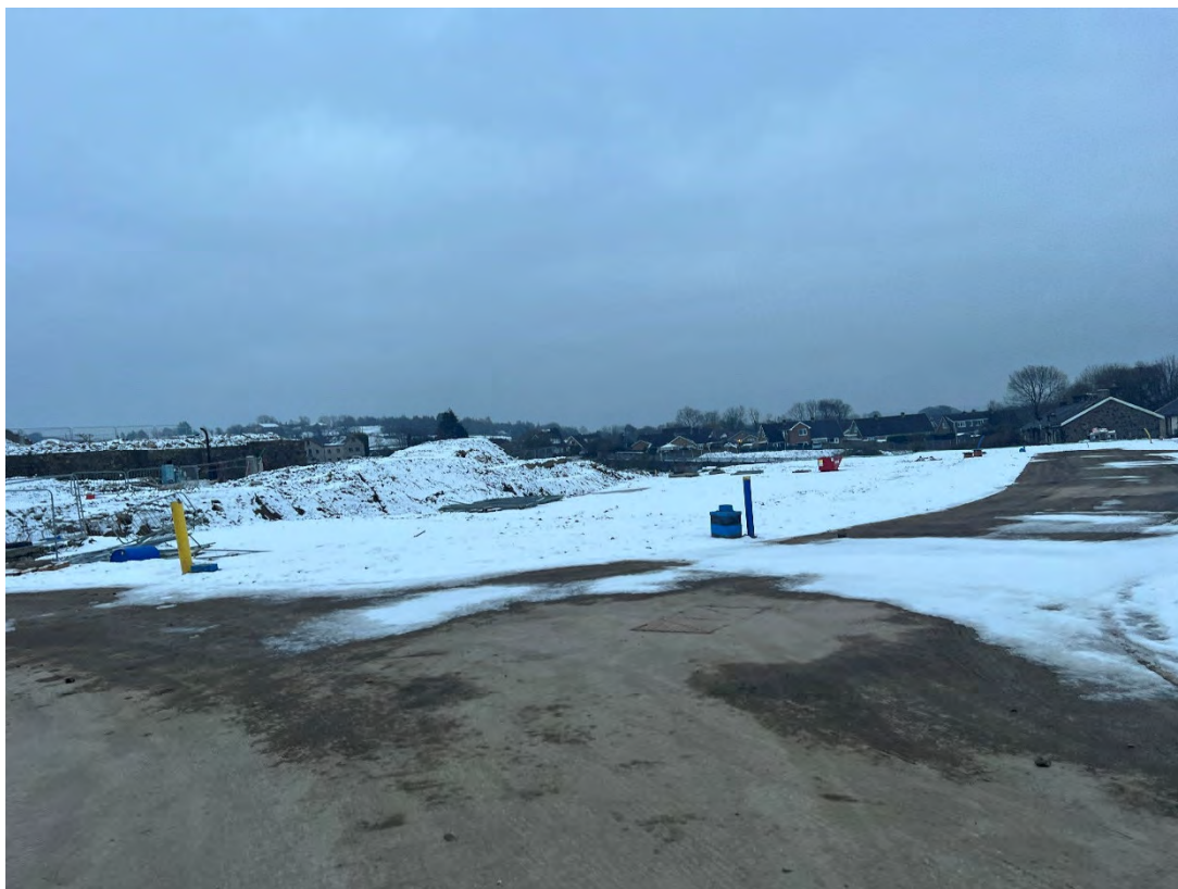
Photograph 38 – Eastern section of Phase 1B.
