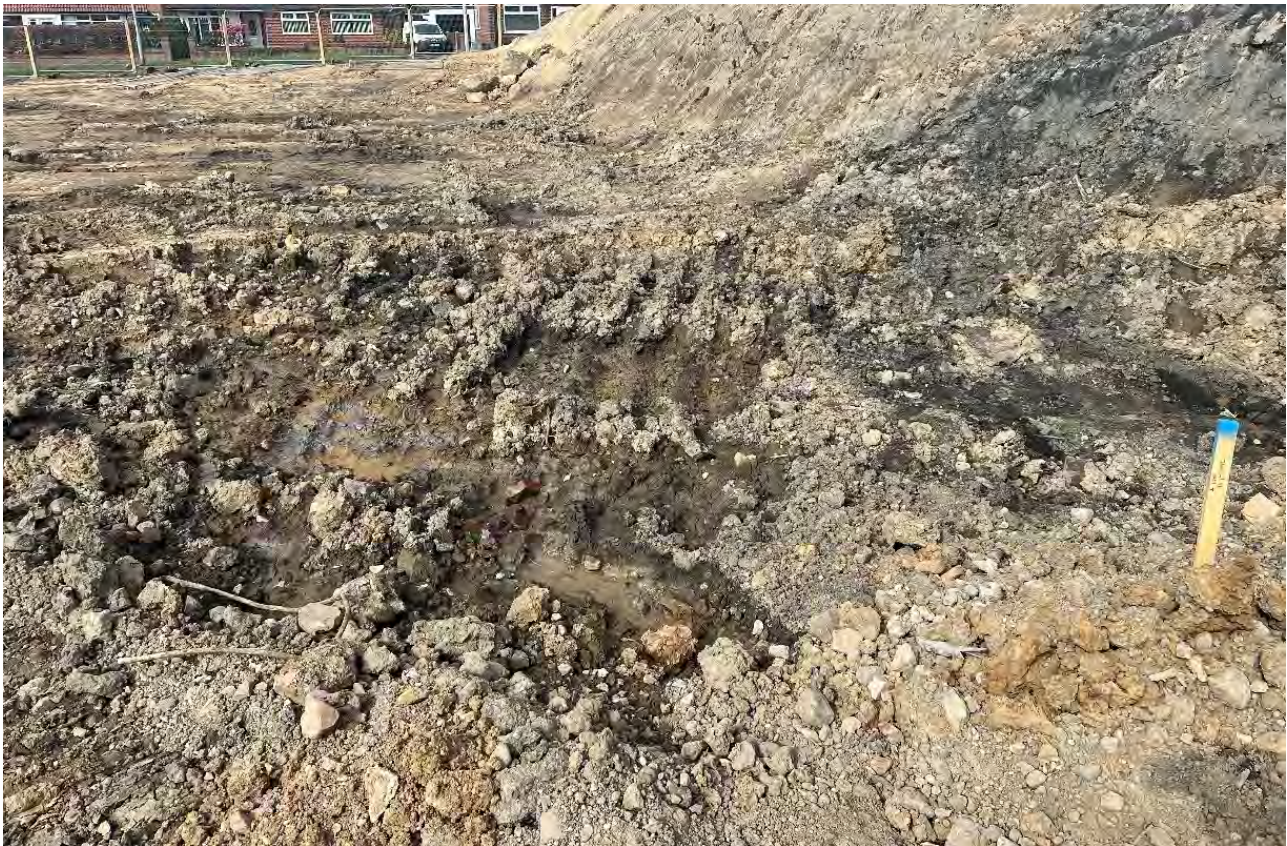
Photograph 19 – Pocket of deeper Made Ground.
