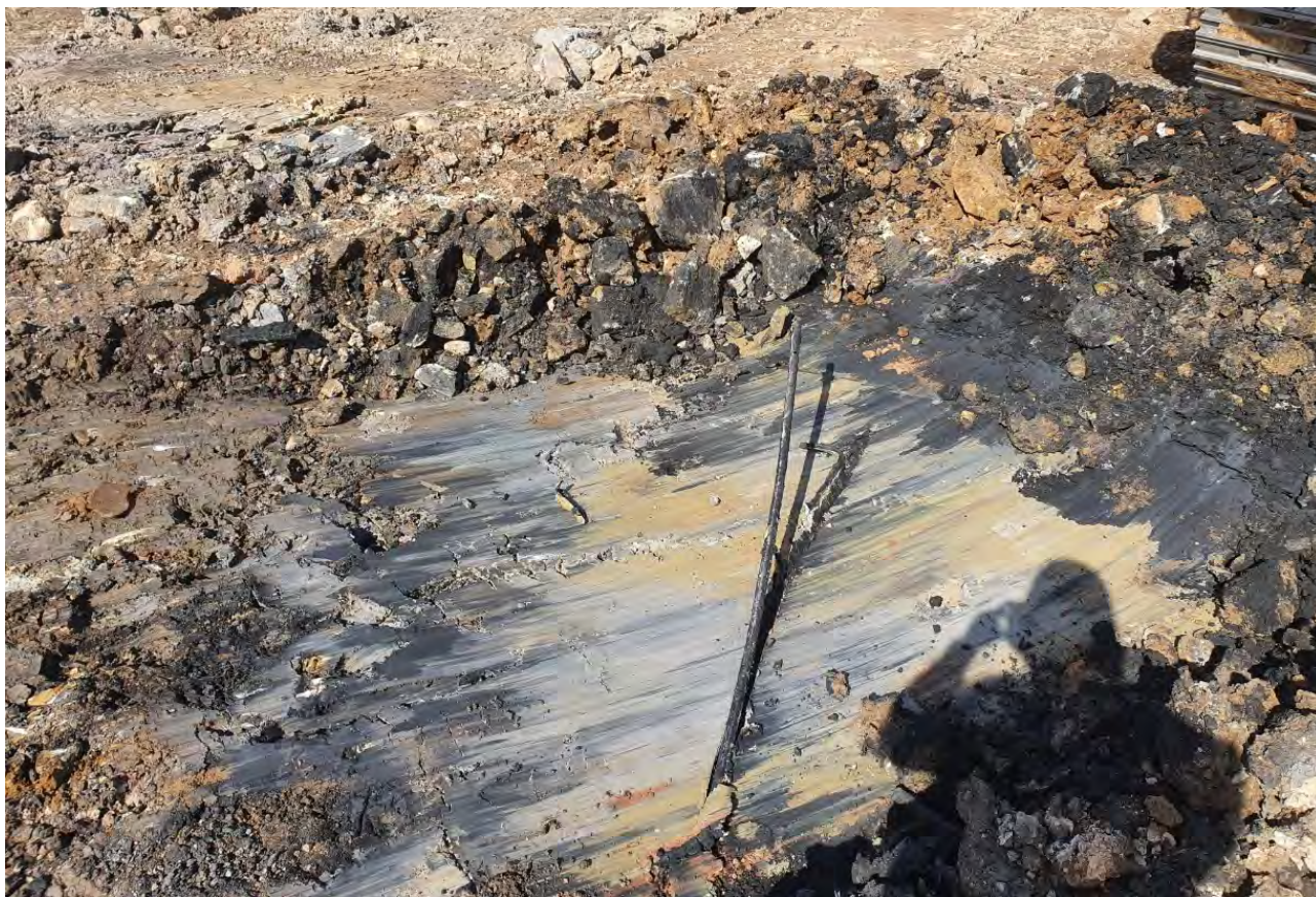
Photograph 23 – Reworked clay and some areas of silt indicated at formation level.
