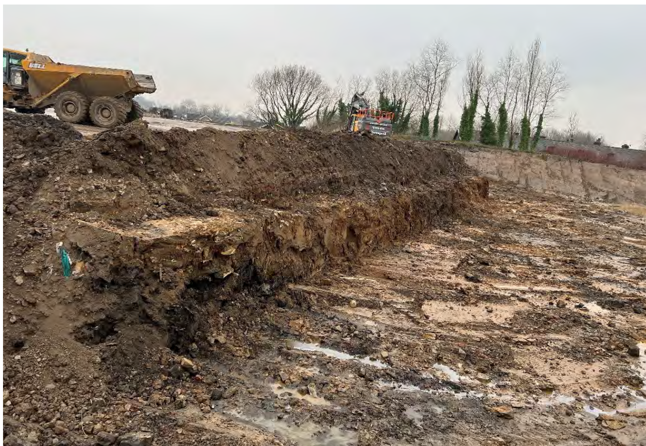
Photograph 12 – Reduced level dig progress.
