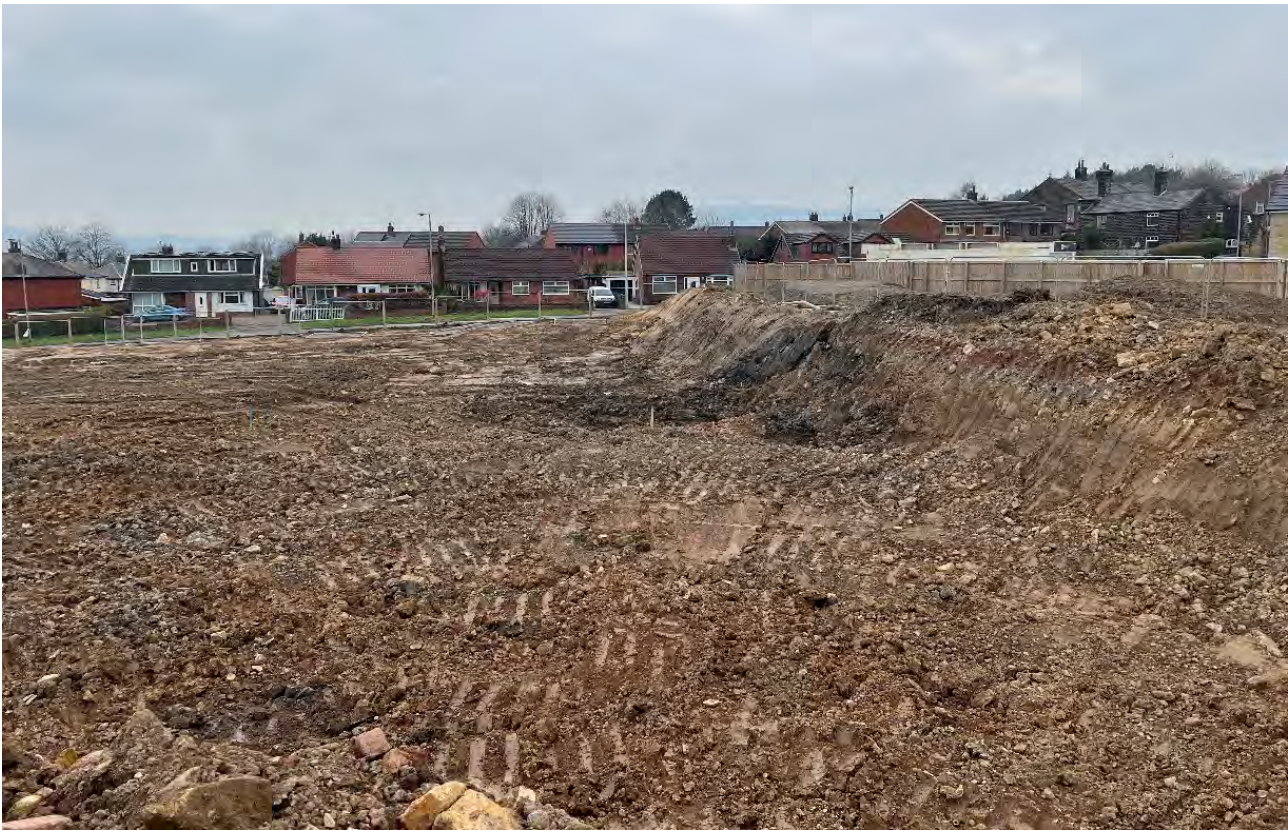
Photograph 16 – Northern extent of reduced level dig.
