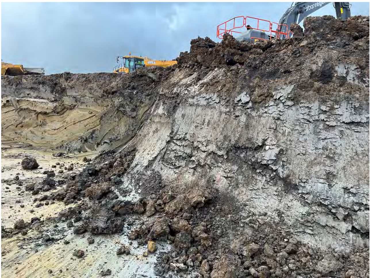
Photograph 8 – Cross profile from existing level to formation.
