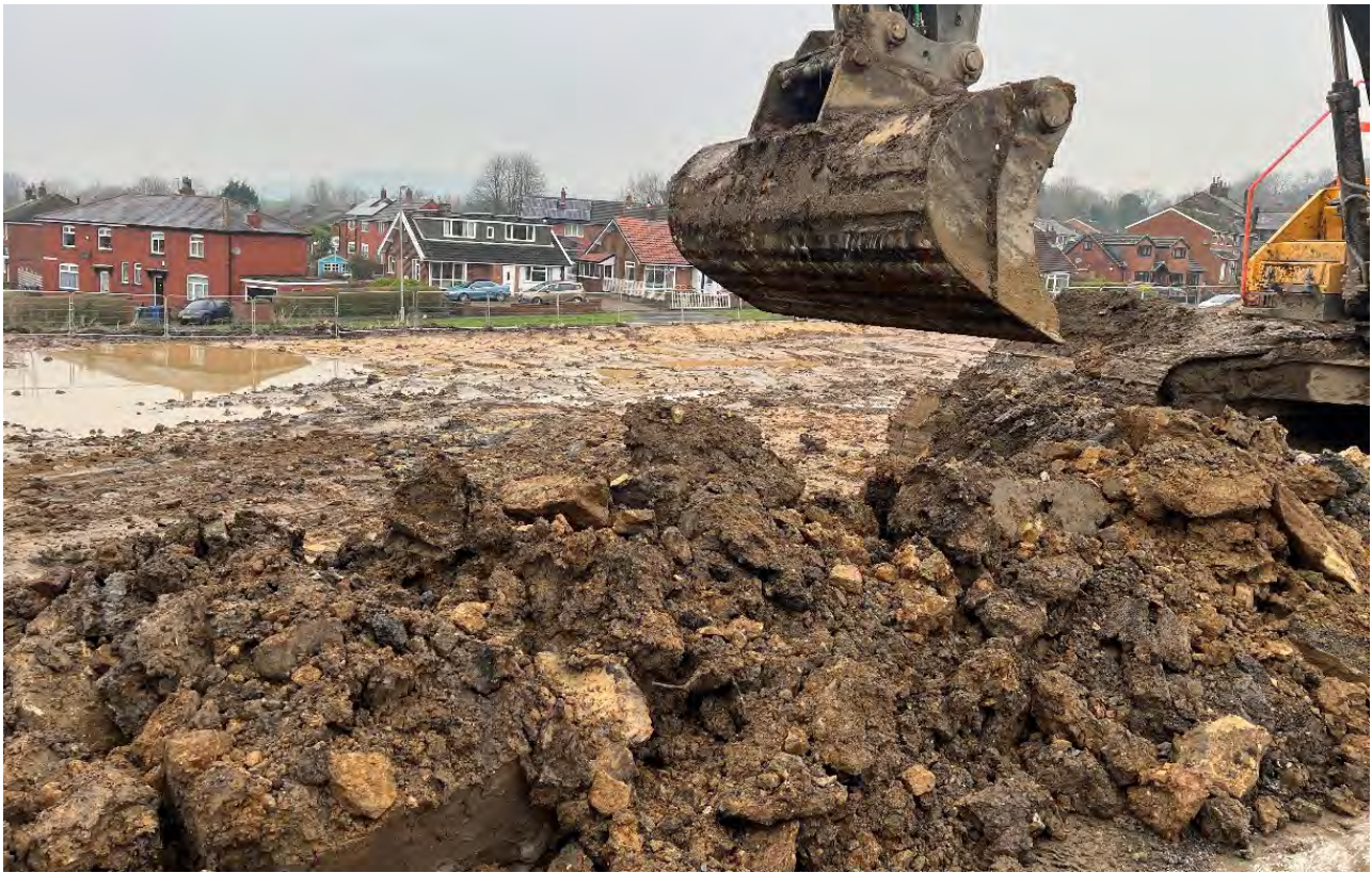
Photograph 10 – Excavation of reworked clay and reduced level dig progress west.
