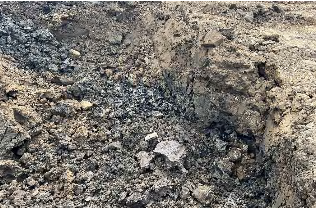
Photograph 34 – Small silt band chased out towards centre of site.
