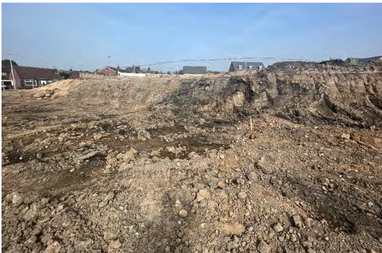
Photograph 20 – Pocket of deeper Made ground & northern area (background) still to be excavated.
