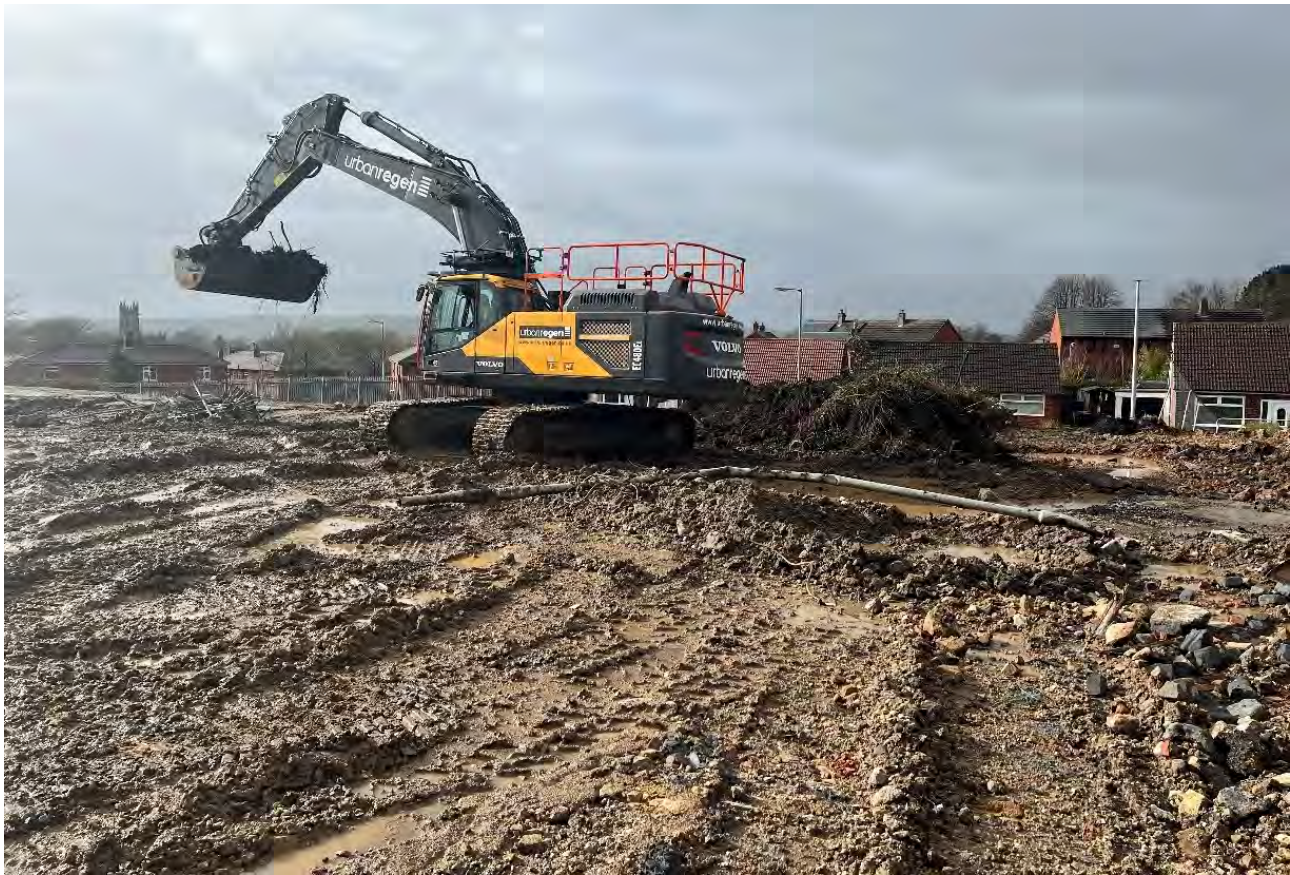
Photograph 4 – Excavation of overlying vegetation at western site boundary.
