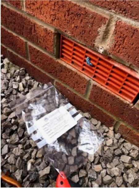
Plot 48 sub-floor void monitoring.
