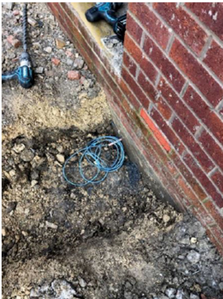
Installation of diffusion tube attached to metal rod into void space. Rope secured for recovery
