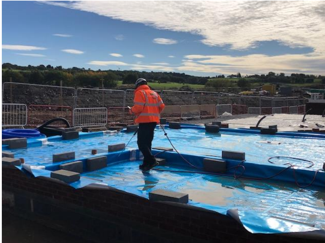
Barratt Bury Photograph 2: VISQUEEN GAS BARRIER Membrane:
