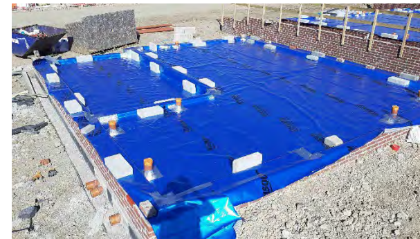
Plot 184: Membrane extends across plot footprints with all areas available for inspection.
