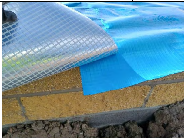
Plot 174: Membrane joins heat welded and >150mm
