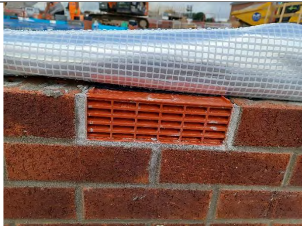
Plot 188: Airbricks installed were clear and free from any obstructions.
