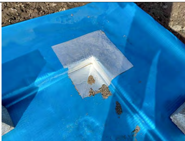
Plot 173: Good detail on cornering using self-adhesive membrane patches.
