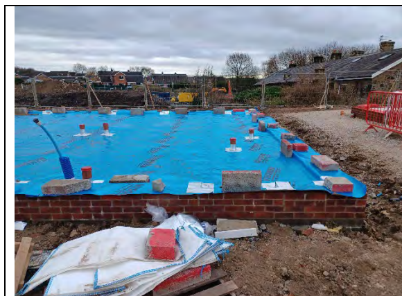
Plot 177: Membrane extends across plot footprint with all areas available for inspection. Standing water indicative of watertight seal achieved
