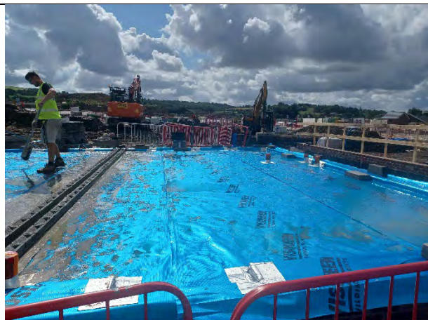
Plot 163: Membrane extends across plot footprint with all areas available for inspection. Standing water indicative of watertight seal achieved.
