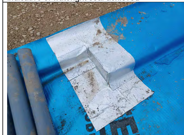
Plot 156: Good detail on cornering using proprietary double and single sided tape, detailing strip to reduce stress points.
