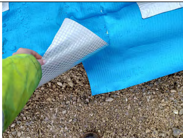
Plot 164: Membrane overlapping external wall. Heated sealed joints between membrane sheets
