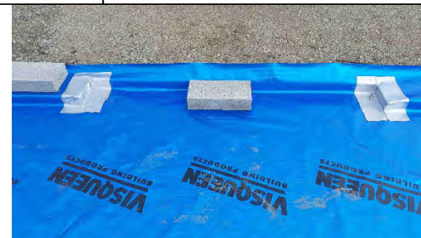
Plot 160: Good detail on cornering using self-adhesive membrane patches.
