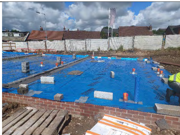
Plot 161: Membrane extends across plot footprint with all areas available for inspection. Standing water indicative of watertight seal achieved
