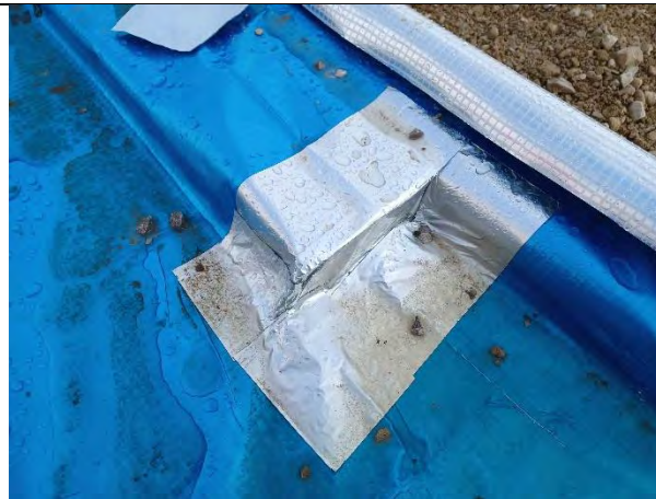
Plot 188: Good detail on cornering using self-adhesive membrane patches.
