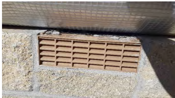
Plot 182: Airbricks installed were clear and free from any obstructions.
