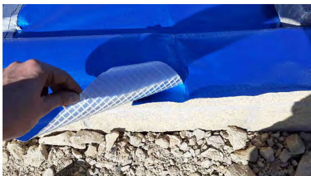
Plot 181: Laps sealed using heat sealed joints
