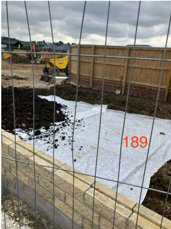
Developer photo showing placement of terram in garden of Plot 189.
