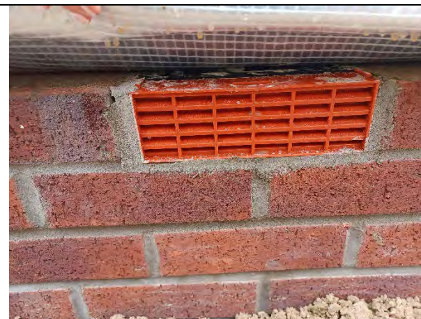
Plot 165: Airbricks installed were clear and free from any obstructions.
