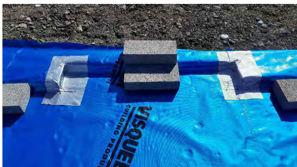
Plot 185: Good detail on cornering using self-adhesive membrane patches.
