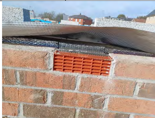
Plot 170: Airbricks installed were clear and free from any obstructions.
