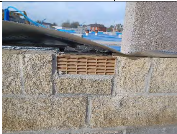
Plot 174: Airbricks installed were clear and free from any obstructions.
