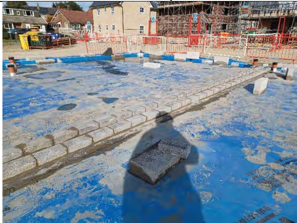
Plot 170: Membrane spans beneath internal wall
