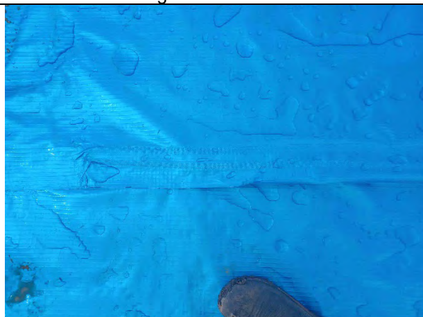
Plot 163: Membrane sealed using heat seal joints; all in good condition.
