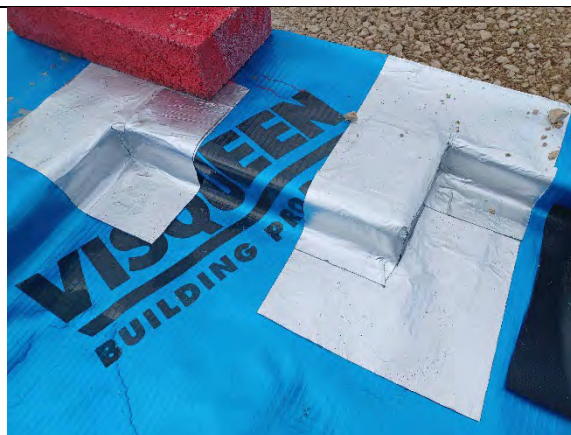
Plot 157: Good detail on cornering using proprietary double and single sided tape detailing strip to reduce stress points.
