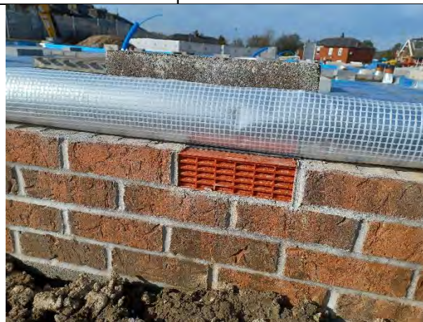
Plot 172: Airbricks installed were clear and free from any obstructions.
