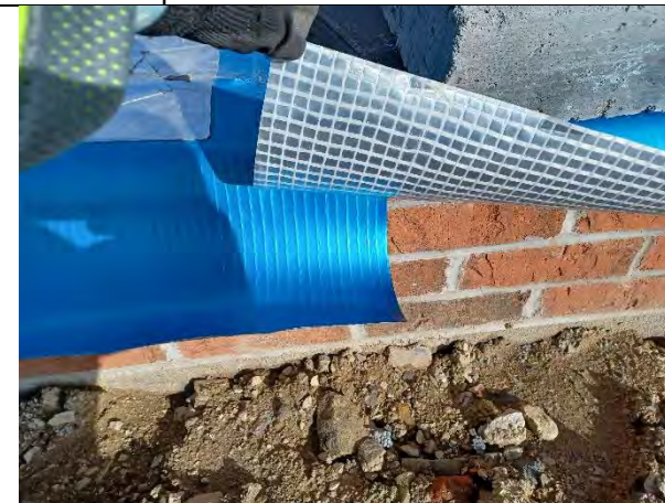
Plot 171: Membrane joins heat welded
