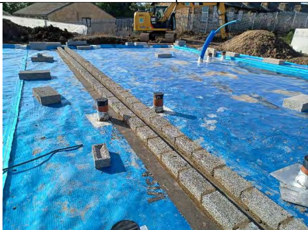
Plot 171: Membrane spans beneath internal wall
