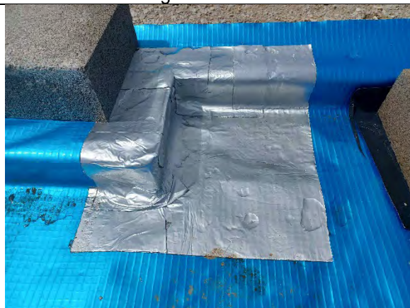
Plot 155: Good corner detailing with no stress points secured using double and single sided tape.
