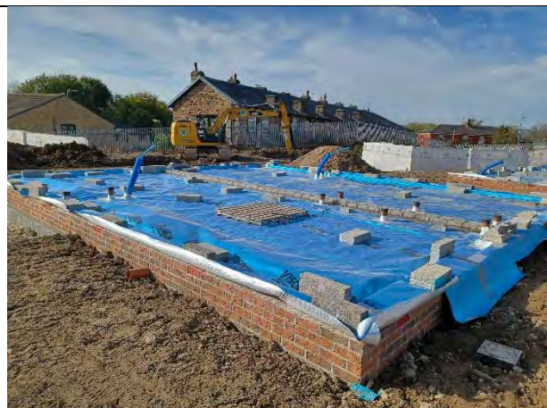
Plot 172: Membrane extends across plot footprints with all areas available for inspection.
