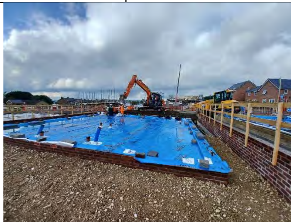
Plot 188: Membrane extends across plot footprints with all areas available for inspection.
