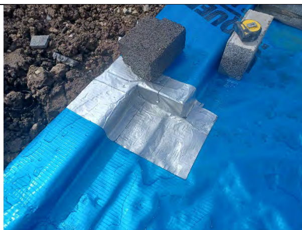
Plot 165: Good detail on cornering using proprietary double and single sided tape, detailing strip to reduce stress points.
