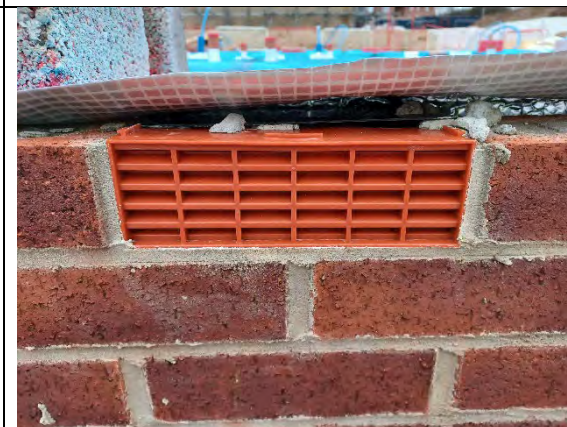
Plot 179: Airbricks installed were clear and free from any obstructions.
