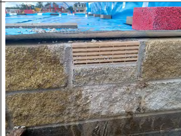
Plot 157: Airbricks installed were clear and free from any obstructions.
