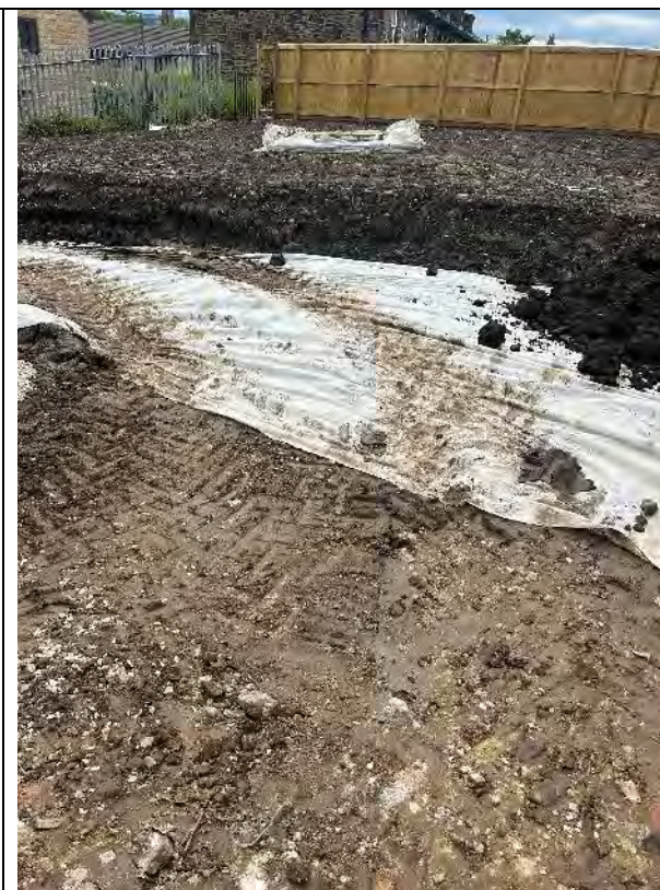
Geotextile membrane placed in Plot 173
