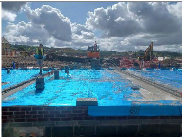
Plot 162: Membrane extends across plot footprint with all areas available for inspection. Standing water indicative of watertight seal achieved
