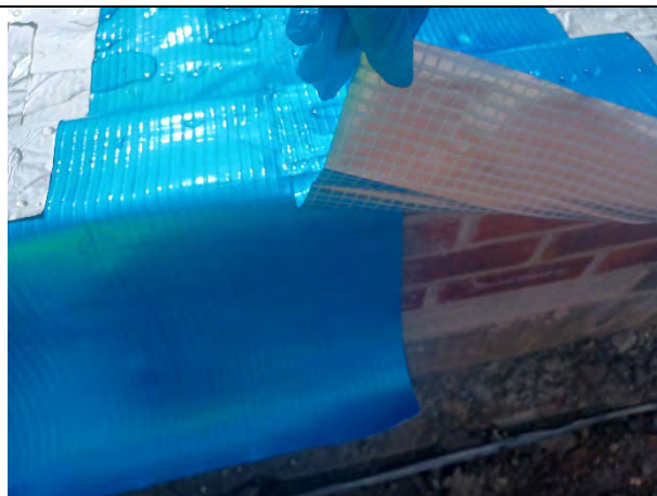
Plot 161: Membrane overlapping external wall.
