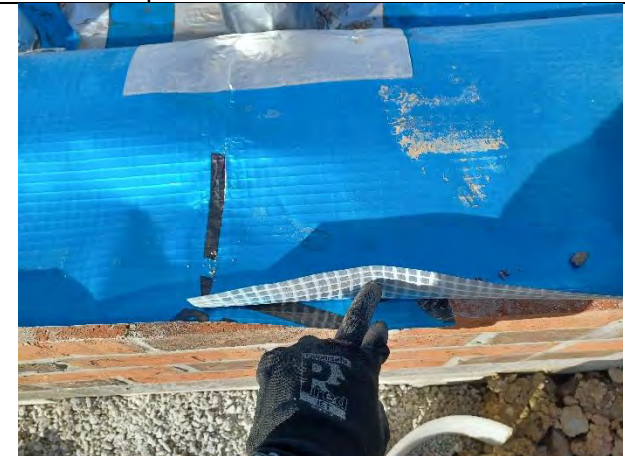
Plot 170: Membrane joins heat welded and >150mm
