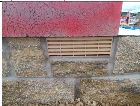
Plot 158 - Airbricks installed were clear and free from any obstructions.
