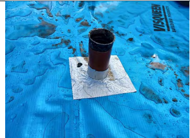
Plot 189: Service entries sealed with self-adhesive membrane patches.
