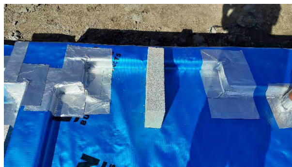
Plot 184: Good detail on cornering using self-adhesive membrane patches.
