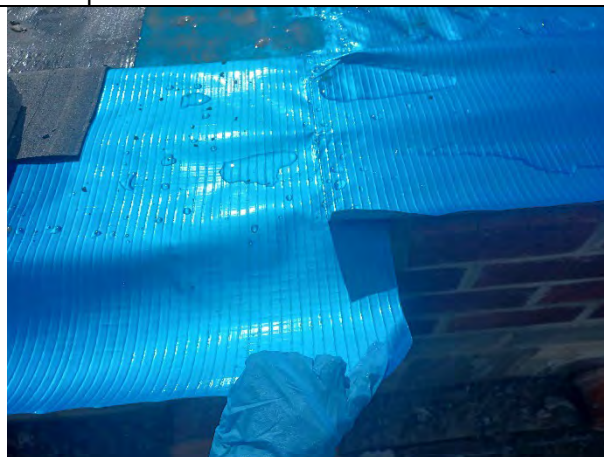
Plot 162: Membrane overlapping external wall.
