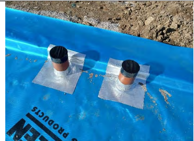
Plot 174: Service entries sealed with self-adhesive membrane patches.
