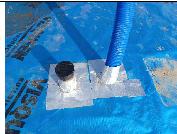
Plot 171: Service entries sealed with self-adhesive membrane patches.
