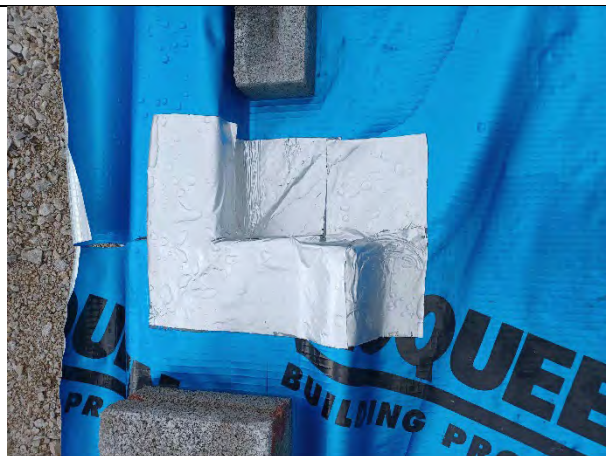
Plot 161: Good detail on cornering using double and single sided tape.
