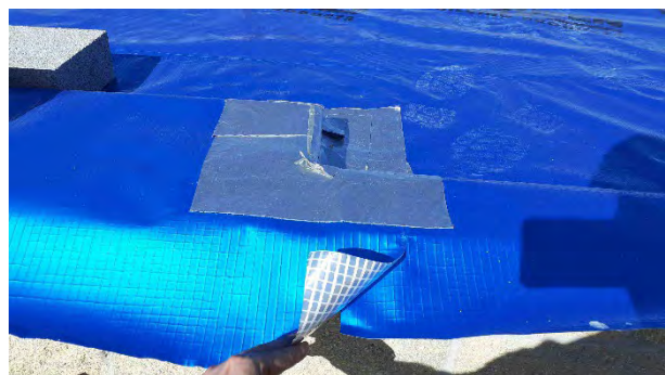
Plot 182: Laps sealed using heat sealed joints
