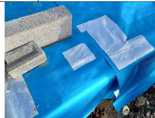
Plot 172: Patch repair made during inspection
