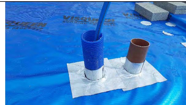
Plot 159: Service entries sealed with self-adhesive membrane patches.
