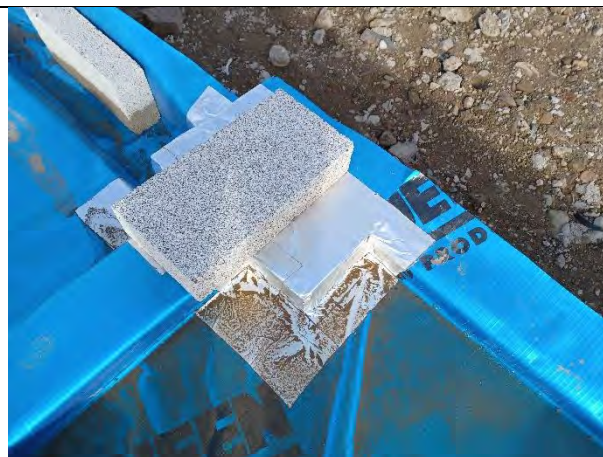
Plot 168: Good detail on cornering using self-adhesive membrane patches.
