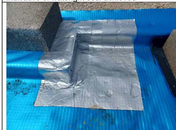
Plot 177: Good corner detailing with no stress points secured using double and single sided tape.
