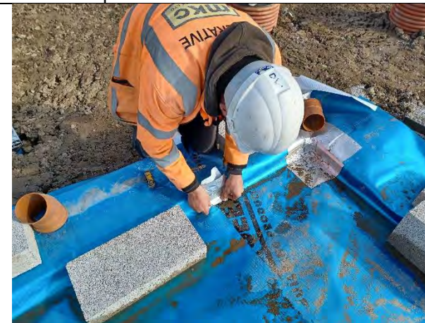
Plot 169: Patch repair made during inspection
