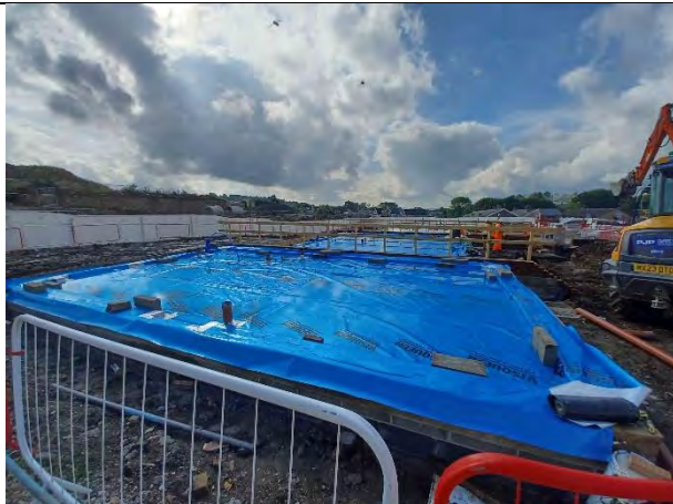
Plot 189: Membrane extends across plot footprints with all areas available for inspection.
