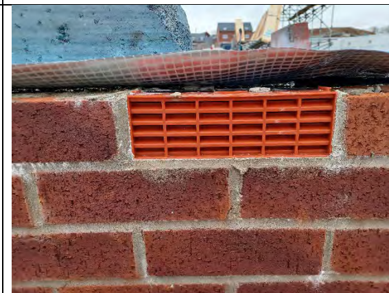
Plot 177: Airbricks installed were clear and free from any obstructions.
