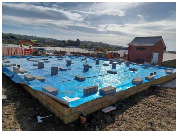
Plot 173: Membrane extends across plot footprints with all areas available for inspection.
