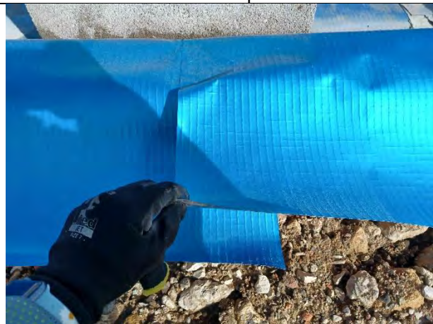
Plot 169: Membrane joins heat welded and >150mm
