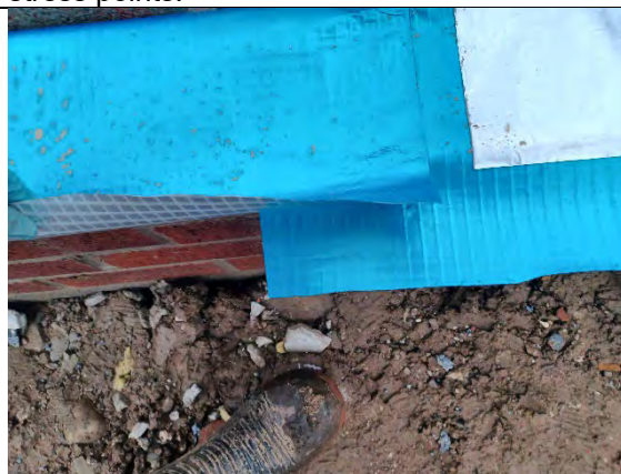
Plot 179: Membrane external wall, overlapping the membrane at the joints.
