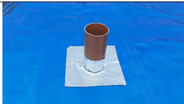
Plot 159: Service entry sealed with self-adhesive membrane patches.
