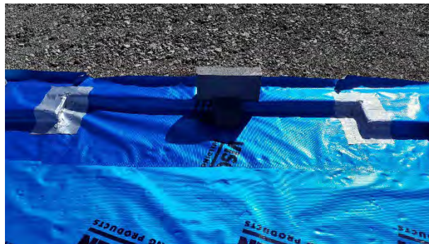
Plot 182: Good detail on cornering using self-adhesive membrane patches.
