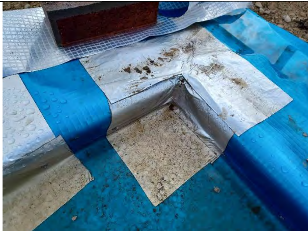
Plot 187: Good detail on cornering using self-adhesive membrane patches.
