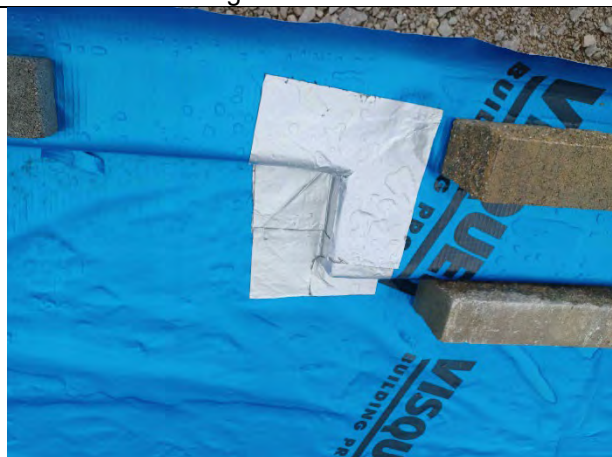
Plot 166: Good corner detailing with no stress points. DPC taped to membrane across cavity wall
