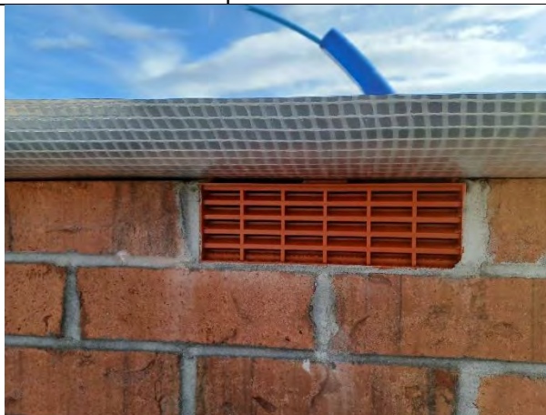
Plot 171: Airbricks installed were clear and free from any obstructions.
