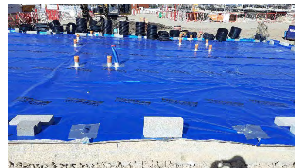
Plot 182: Membrane extends across plot footprints with all areas available for inspection.
