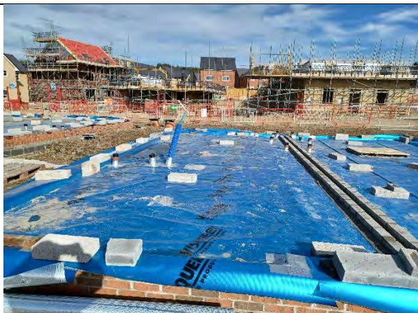
Plot 171: Membrane extends across plot footprints with all areas available for inspection.
