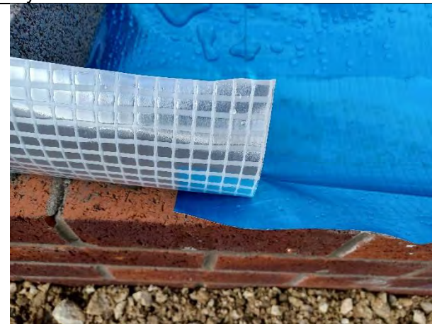
Plot 188: Laps sealed using heat sealed joints >150mm
