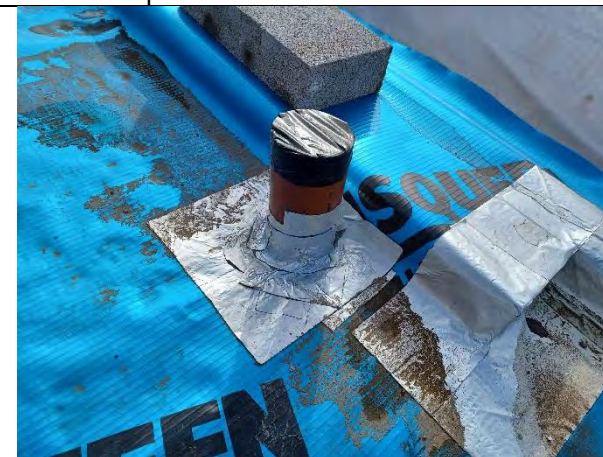
Plot 168: Patch repair made during inspection
