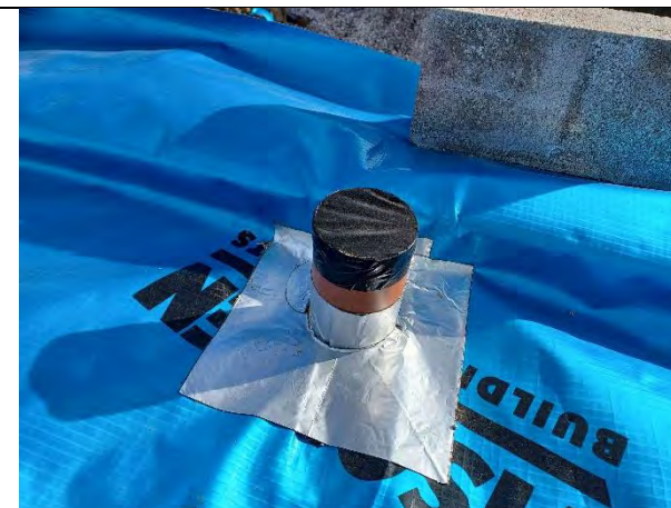
Plot 172: Service entries sealed with self-adhesive membrane patches.
