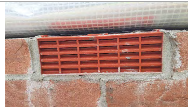
Plot 160: Airbricks installed were clear and free from any obstructions.
