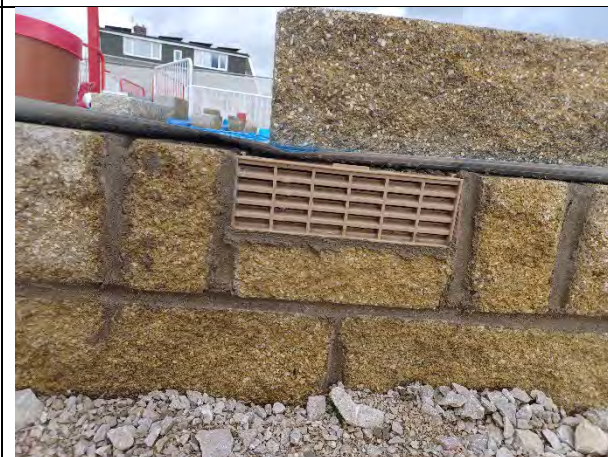
Plot 166: Airbricks installed were clear and free from any obstructions.
