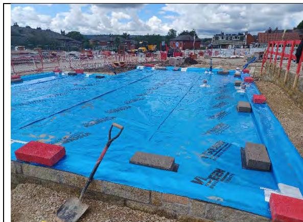
Plot 157: Membrane extends across plot footprint with all areas available for inspection. Standing water indicative of watertight seal achieved.
