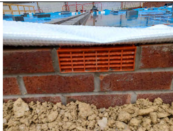
Plot 164: Airbricks installed were clear and free from any obstructions.
