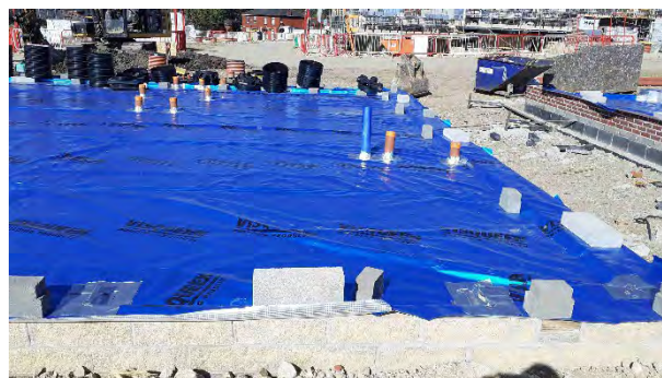
Plot 183: Membrane extends across plot footprints with all areas available for inspection.
