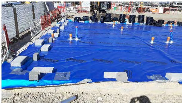
Plot 181: Membrane extends across plot footprints with all areas available for inspection.
