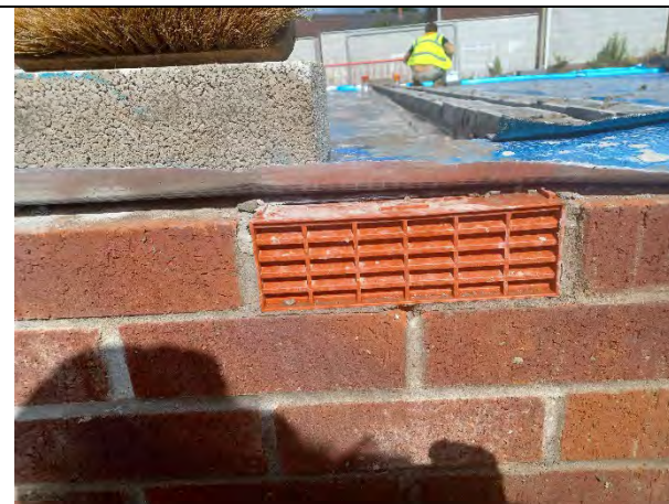
Plot 163: Airbricks installed were clear and free from any obstructions.
