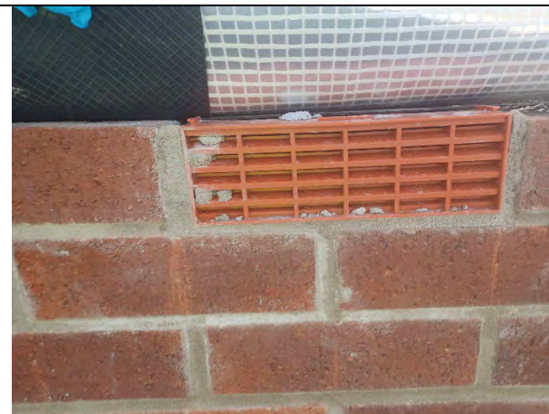
Plot 162: Airbricks installed were clear and free from any obstructions.
