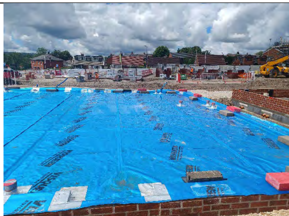
Plot 155: Membrane extends across plot footprint with all areas available for inspection. Standing water indicative of watertight seal achieved
