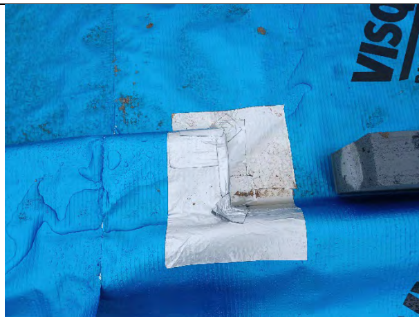
Plot 164: Good detail on cornering using double and single sided tape.
