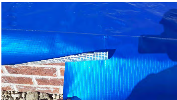
Plot 184: Laps sealed using heat sealed joints
