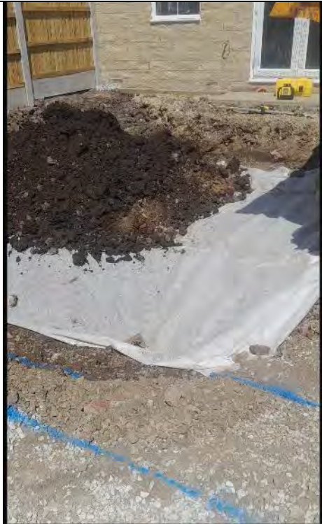
Geotextile membrane placed in Plot 174
