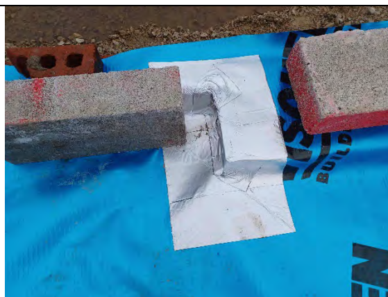
Plot 179: Good detail on cornering using proprietary double and single sided tape detailing strip to reduce stress points.
