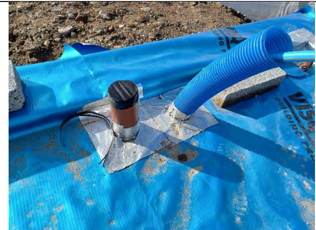
Plot 170: Service entries sealed with self-adhesive membrane patches.
