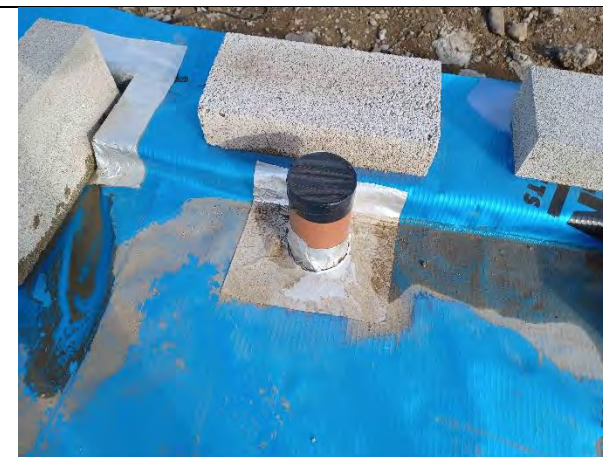
Plot 168: Service entries sealed with self-adhesive membrane patches.
