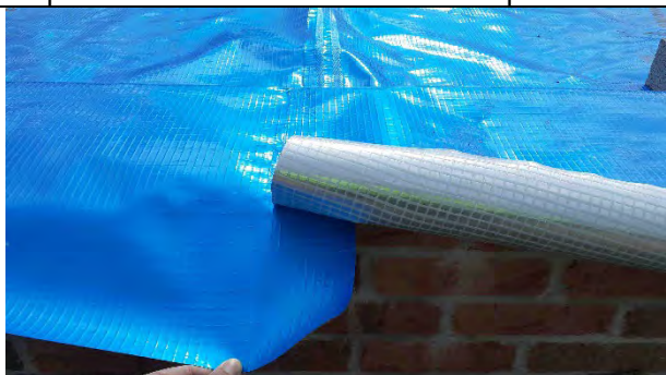
Plot 159: Laps sealed using heat sealed joints
