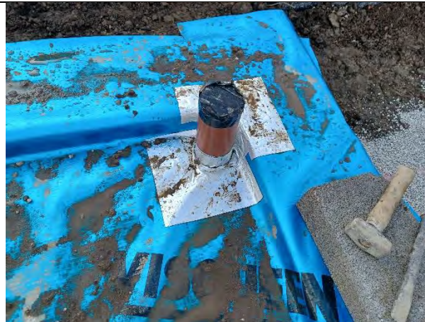
Plot 187: Service entries sealed with self-adhesive membrane patches.
