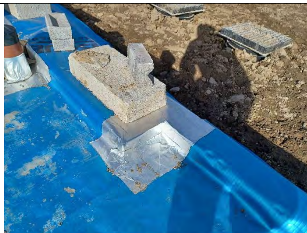
Plot 172: Good detail on cornering using self-adhesive membrane patches.
