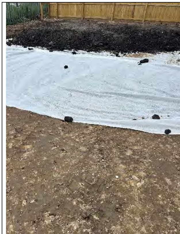
Geotextile membrane placed in Plot 171
