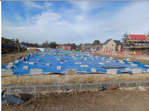
Plot 174: Membrane extends across plot footprints with all areas available for inspection.
