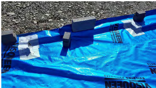
Plot 183: Good detail on cornering using self-adhesive membrane patches.
