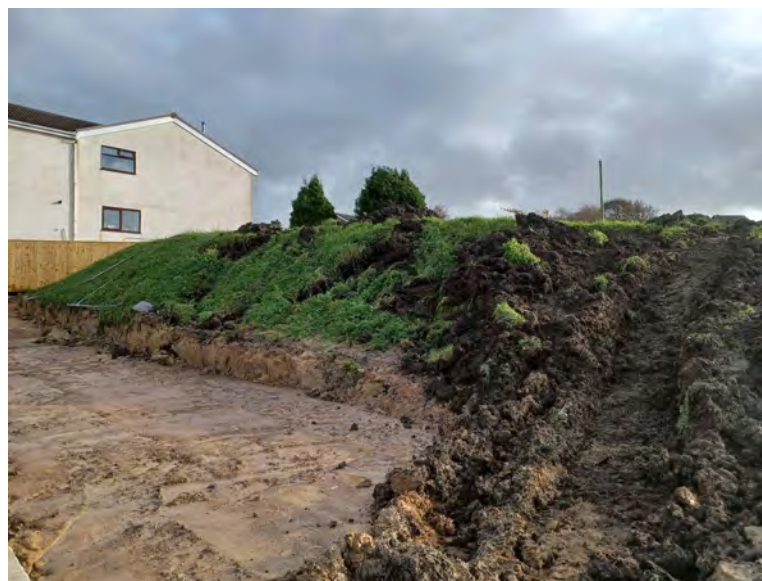
Photograph (Topsoil Stockpile A)
