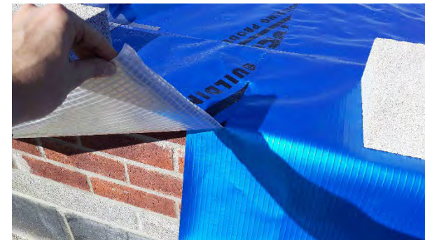
Plot 185: Laps sealed using heat sealed joints
