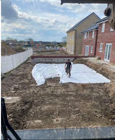
Photographs provided for developer, Barratt Homes, of membrane installation over Plots 185-186.
