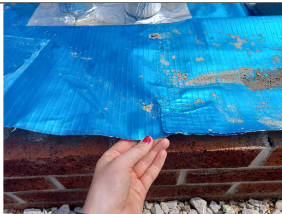
Plot 155: Membrane external wall, overlapping the membrane at the joints.
