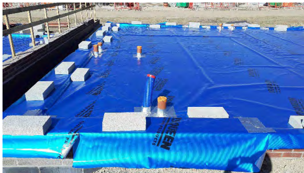
Plot 185: Membrane extends across plot footprints with all areas available for inspection.
