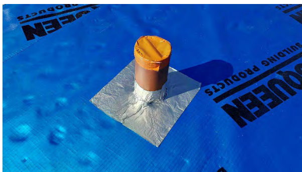
Plot 185: Service entries sealed with self-adhesive membrane patches.
