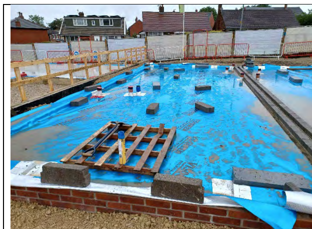
Plot 165: Membrane extends across plot footprint with all areas available for inspection. Standing water indicative of watertight seal achieved
