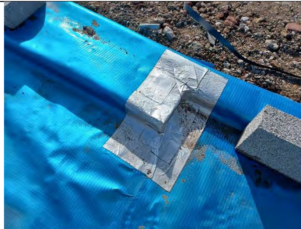
Plot 170: Good detail on cornering using self-adhesive membrane patches.
