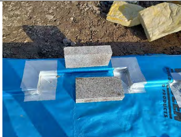
Plot 174: Good detail on cornering using self-adhesive membrane patches.
