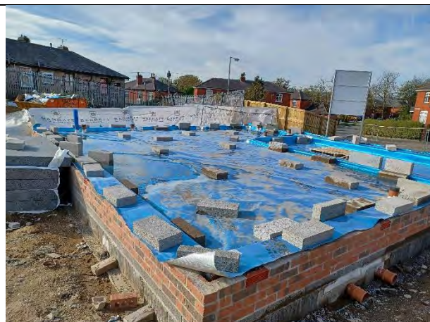
Plot 168: Membrane extends across plot footprint with all areas available for inspection.
