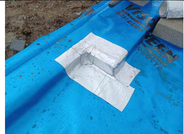
Plot 189: Patch repair made during inspection
