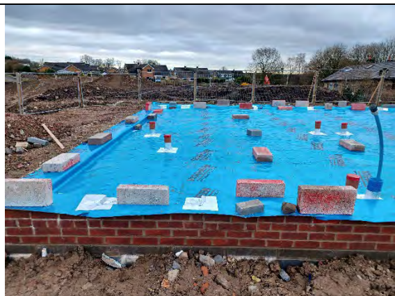
Plot 180 - Membrane extends across plot footprint with all areas available for inspection. Standing water indicative of watertight seal achieved.
