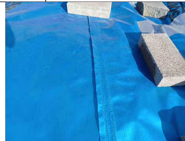
Plot 173: Heat welded joins between membrane sheets
