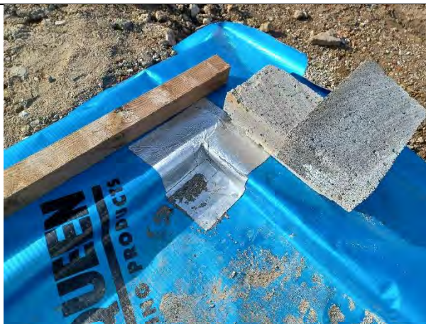
Plot 171: Good detail on cornering using self-adhesive membrane patches.
