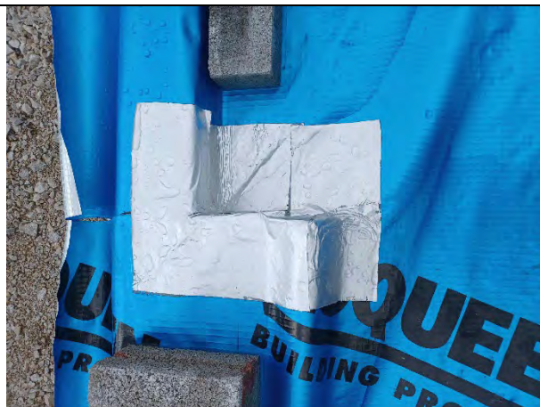
Plot 166: Good detail on cornering using proprietary detailing strip to reduce stress points; DPC taped to gas membrane extending to external wall
