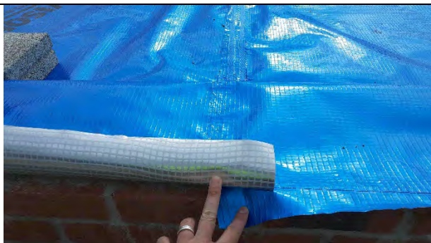
Plot 160: Laps sealed using heat sealed joints.
