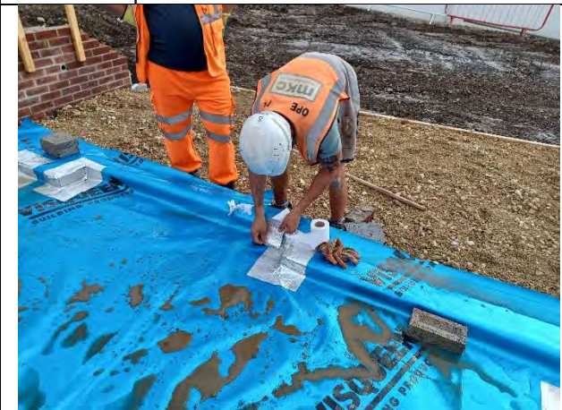
Plot 188: Patch repair made during inspection
