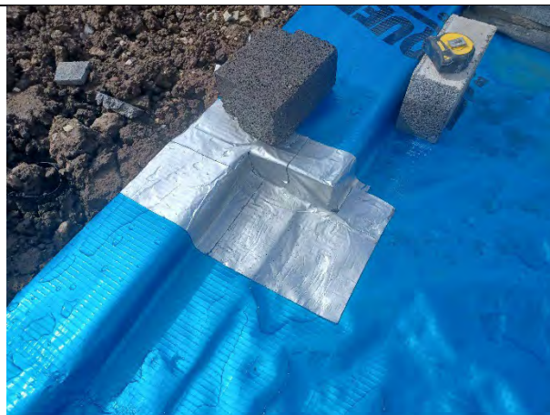
Plot 163: Good detail on cornering using proprietary double and single sided tape detailing strip to reduce stress points.
