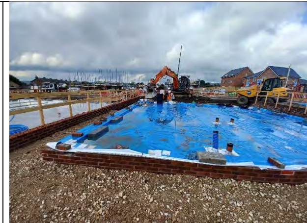
Plot 187: Membrane extends across plot footprints with all areas available for inspection.
