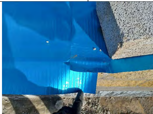
Plot 173: Membrane joins heat welded
