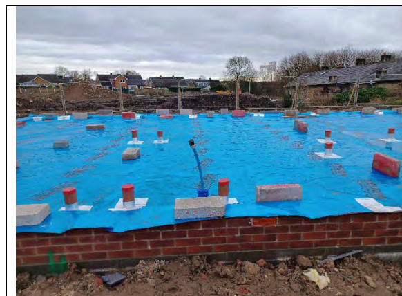
Plot 179: Membrane extends across plot footprint with all areas available for inspection. Standing water indicative of watertight seal achieved.
