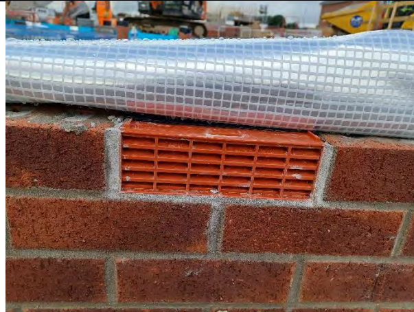
Plot 189: Airbricks installed were clear and free from any obstructions.
