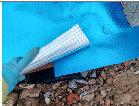
Plot 177: Membrane external wall, overlapping the membrane at the joints.
