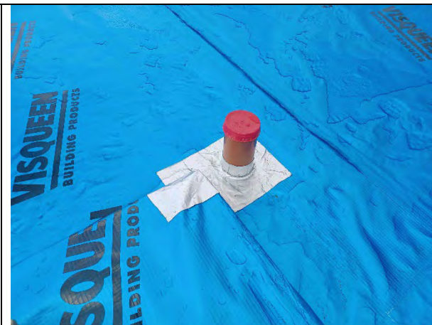
Plot 166: Service entry sealed with top hat, double and single sided tape and a jubilee clip
