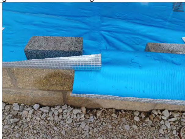
Plot 166: Membrane overlapping external wall.
