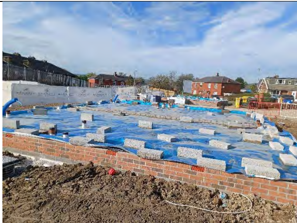
Plot 170: Membrane extends across plot footprints with all areas available for inspection.
