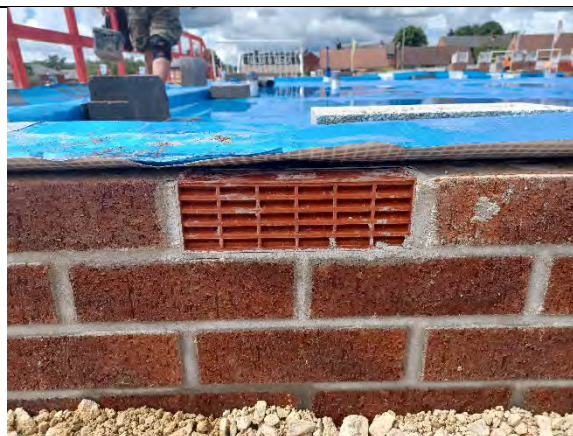
Plot 156: Airbricks installed were clear and free from any obstructions.
