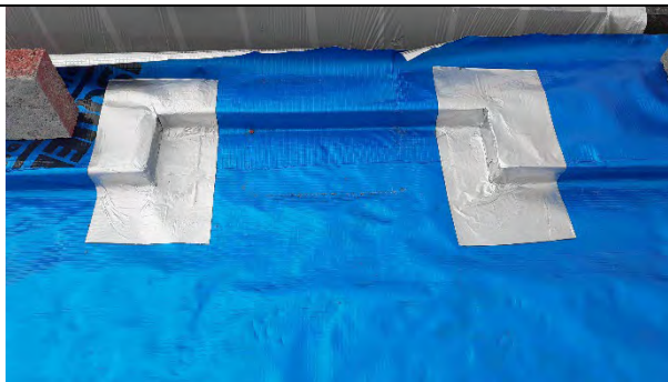
Plot 159: Good detail on cornering using self-adhesive membrane patches.
