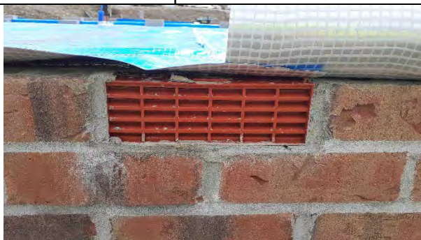
Plot 159: Airbricks installed were clear and free from any obstructions.
