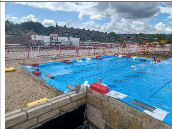
Plot 158 - Membrane extends over plots 157-158.
