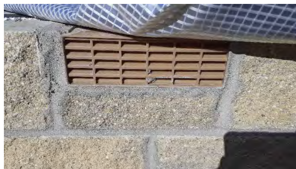
Plot 181: Airbricks installed were clear and free from any obstructions.
