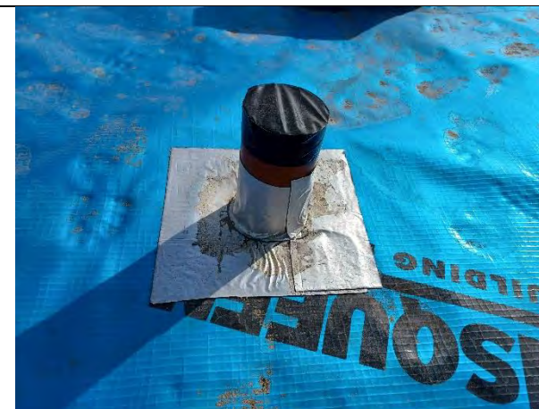
Plot 169: Service entries sealed with self-adhesive membrane patches.
