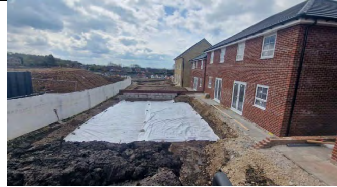
Photographs provided for developer, Barratt Homes, of membrane installation over Plots 185-186.
