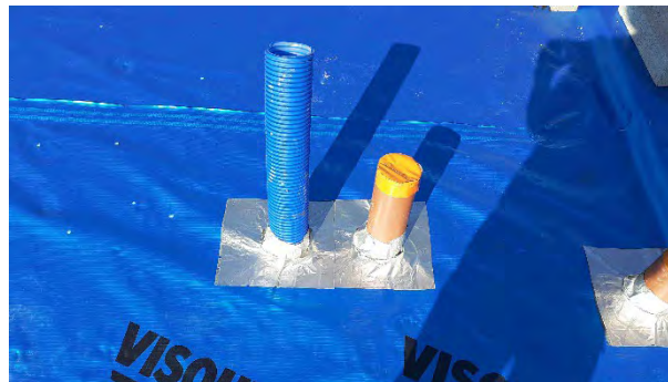
Plot 183: Service entries sealed with self-adhesive membrane patches.
