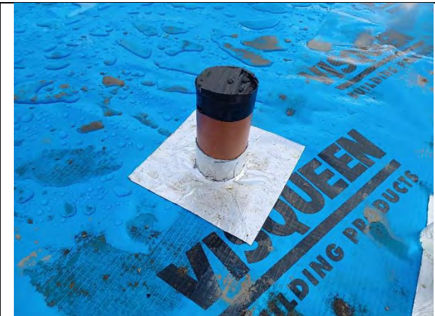
Plot 188: Service entries sealed with self-adhesive membrane patches.
