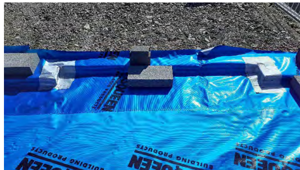
Plot 181: Good detail on cornering using self-adhesive membrane patches.
