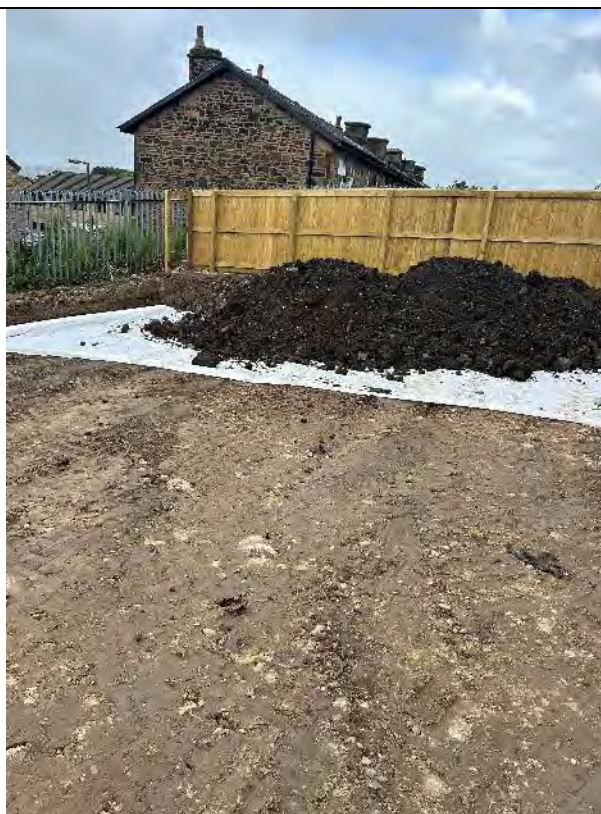
Geotextile membrane placed in Plot 172
