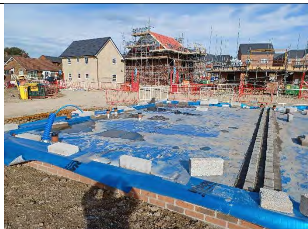
Plot 169: Membrane extends across plot footprints with all areas available for inspection.
