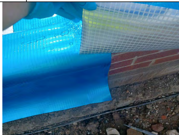
Plot 163: Membrane overlapping external wall.
