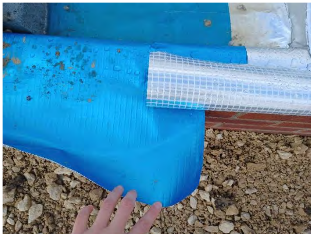
Plot 187: Laps sealed using heat sealed joints
