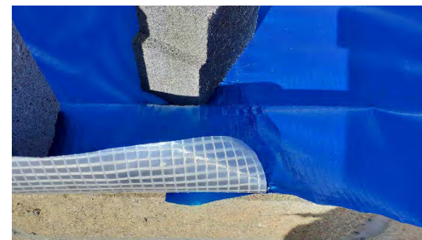
Plot 183: Laps sealed using heat sealed joints
