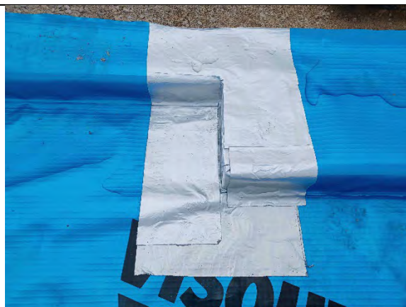
Plot 158 - Good detail on cornering using proprietary double and single sided tape detailing strip to reduce stress points.
