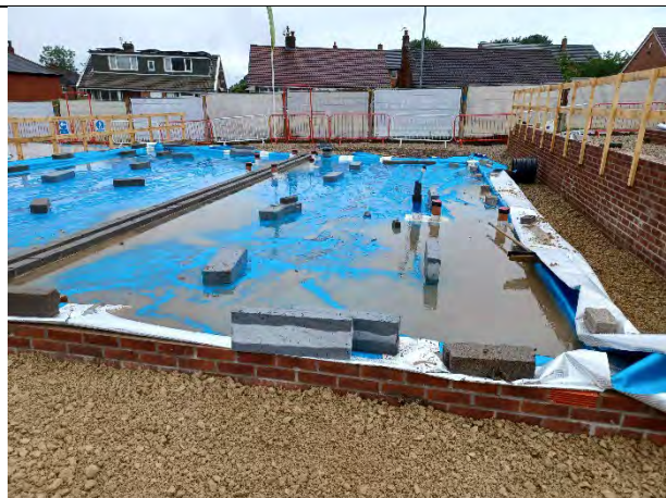
Plot 164: Membrane extends across plot footprint with all areas available for inspection. Standing water indicative of watertight seal achieved
