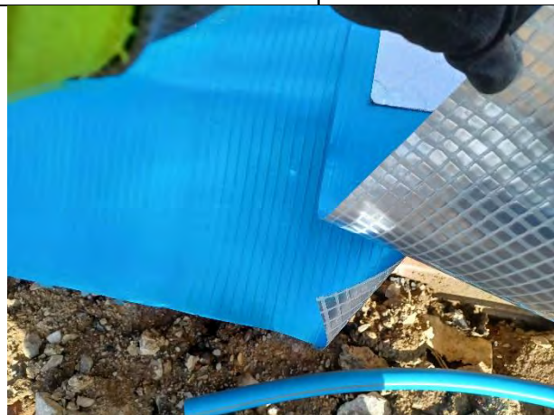
Plot 172: Membrane joins heat welded and >150mm
