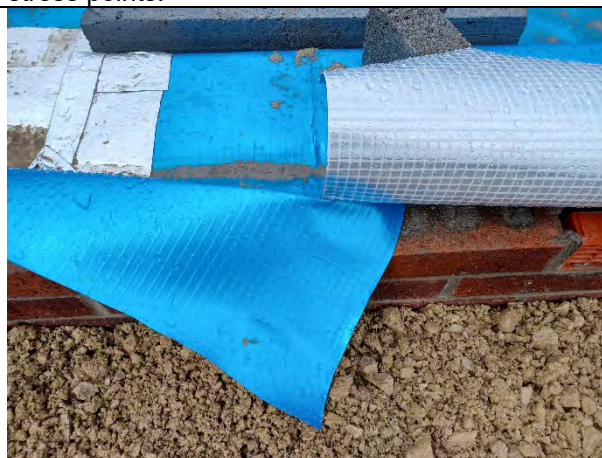
Plot 165: Membrane overlapping external wall.
