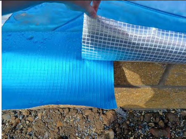
Plot 189: Laps sealed using heat sealed joints
