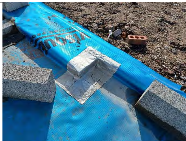
Plot 169: Good detail on cornering using self-adhesive membrane patches.
