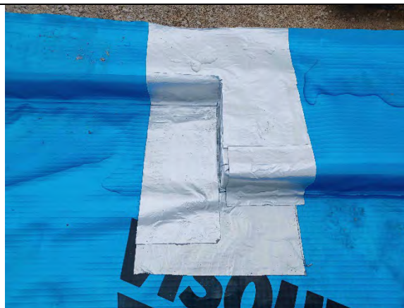
Plot 180 - Good detail on cornering using proprietary double and single sided tape detailing strip to reduce stress points.
