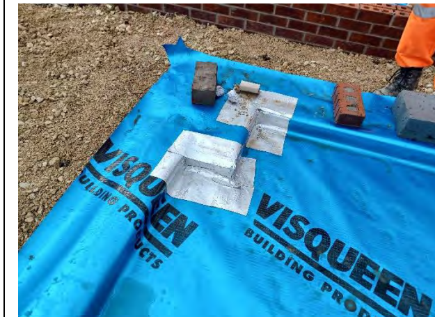
Plot 187: Patch repair made during inspection
