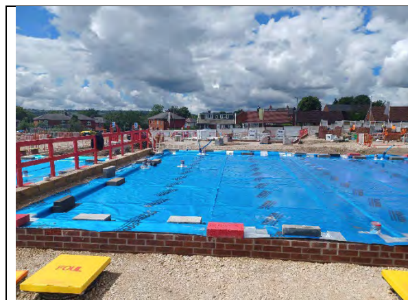
Plot 156: Membrane extends across plot footprint with all areas available for inspection. Standing water indicative of watertight seal achieved
