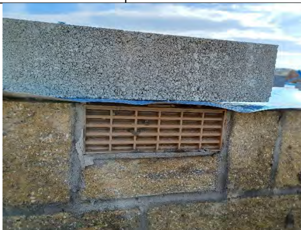
Plot 173: Airbricks installed were clear and free from any obstructions.
