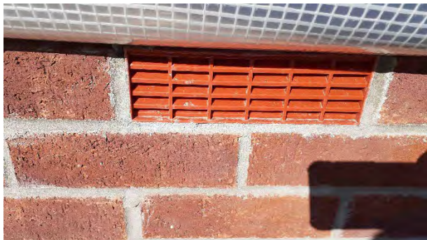
Plot 184: Airbricks installed were clear and free from any obstructions.
