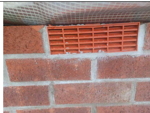
Plot 161: Airbricks installed were clear and free from any obstructions.
