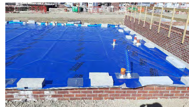
Plot 186: Membrane extends across plot footprints with all areas available for inspection.
