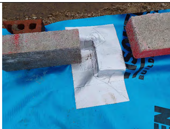
Plot 177: Good detail on cornering using double and single sided tape.
