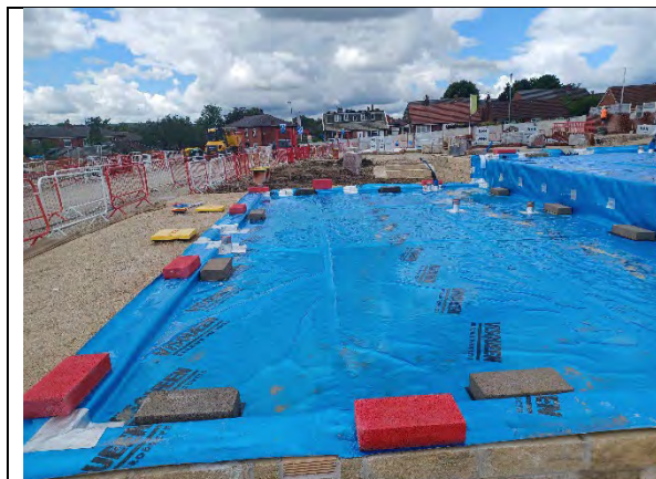
Plot 158 - Membrane extends across plot footprint with all areas available for inspection. Standing water indicative of watertight seal achieved.
