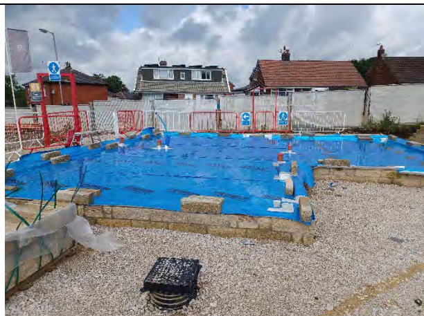
Plot 166: Membrane extends across plot footprint with all areas available for inspection. Standing water indicative of watertight seal achieved
