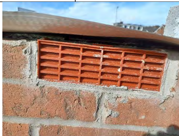
Plot 168: Airbricks installed were clear and free from any obstructions.
