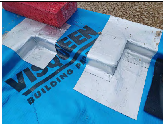
Plot 155: Good detail on cornering using double and single sided tape.
