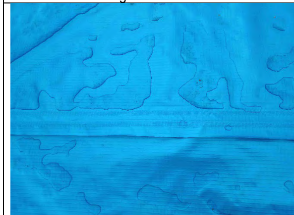
Plot 157: Membrane sealed using heat seal joints; all in good condition.
