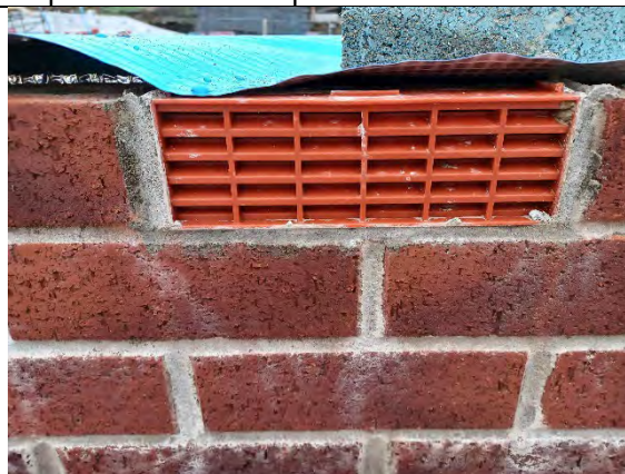
Plot 180 - Airbricks installed were clear and free from any obstructions.
