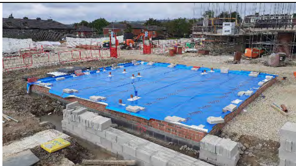
Plots 159 & 160: Membrane extends across plot footprints with all areas available for inspection.
