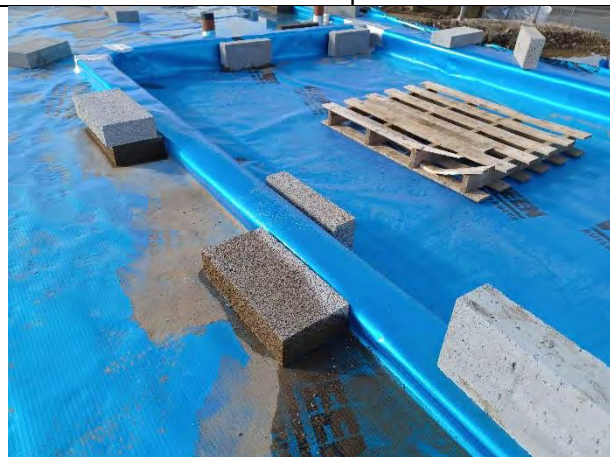
Plot 168: Membrane neatly spans internal wall
