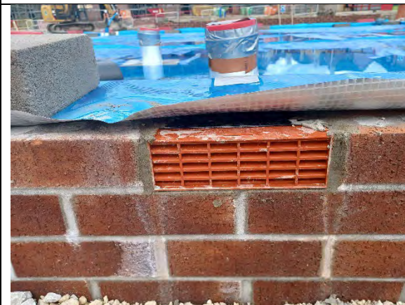
Plot 155: Airbricks installed were clear and free from any obstructions.
