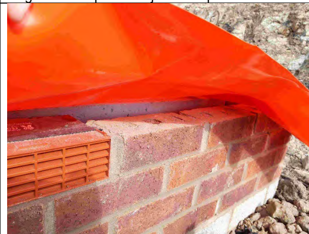
Plot 5: Membrane extends across outer wall
