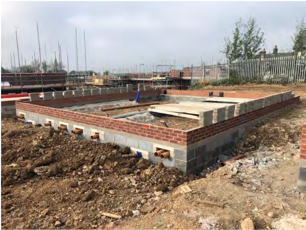
Barratt Bury Photograph 3: Example beam and block construction:
