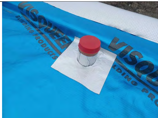
Plot 149: Service entry sealed using proprietary detailing strip
