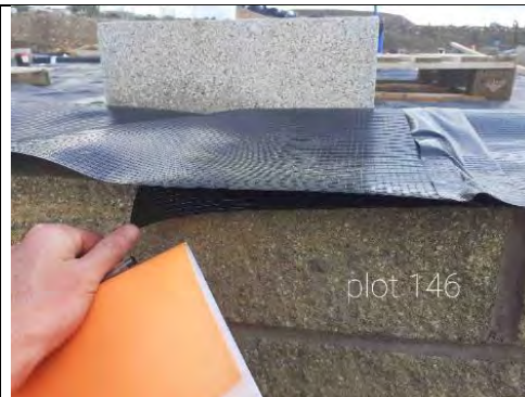
Plot 146: Overlap in membrane sheets to gas resistant DPC >150mm
