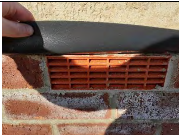
Plot 10: Airbricks installed were clear and free from any obstructions.
