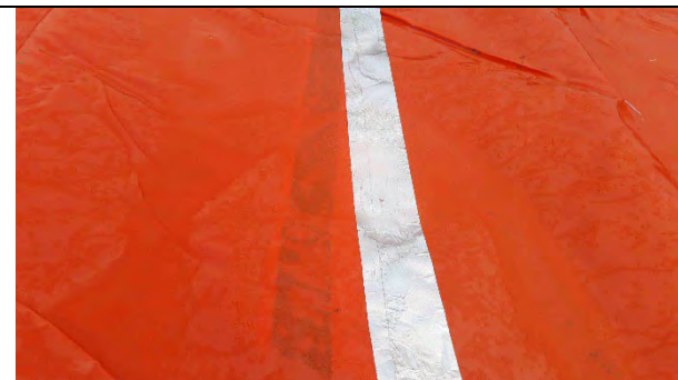
Plot 19: Overlap in membrane sheets >150mm and sealed with double and single sided tape
