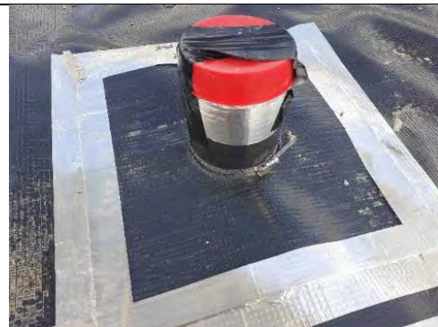
Plot 146: Service entry sealed with top hat, double and single sided tape and a jubilee clip.
