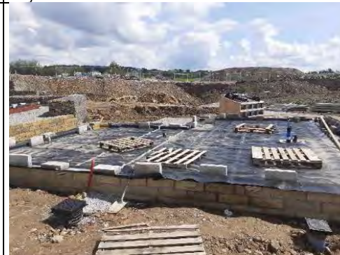
Plot 146: Membrane fully exposed and in good condition.
