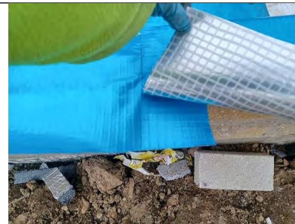
Plot 151: Overlap in membrane sheets >150mm and sealed with heat gun.
