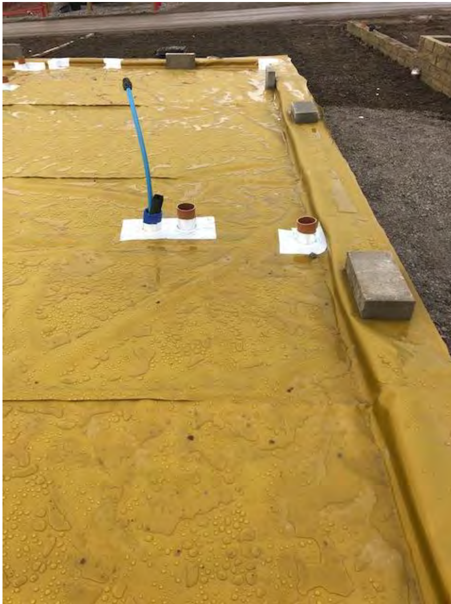
Photo 3: Barratts Bury: Corner and Penetration detailing:
