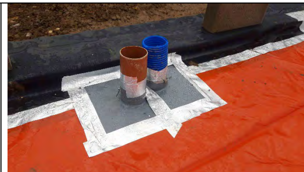
Plot 19: Service entries sealed with top hat, double and single sided tape and a jubilee clip
