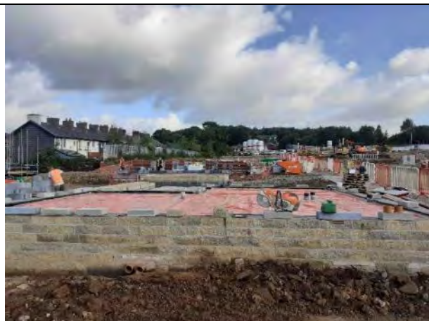
Plot 9: Membrane fully exposed and in good condition.
