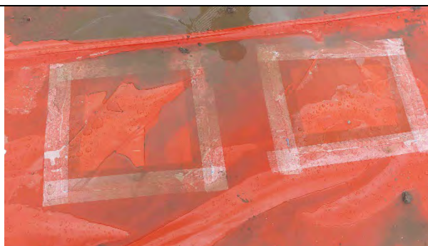
Plot 4: 2 patches to repair tears combination of membrane patch and double and single sided tape used.
