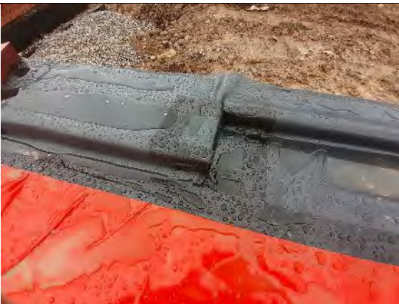
Plot 14: Good detail on cornering using proprietary detailing strip to reduce stress points.
