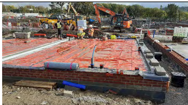
Plot 16: Membrane fully exposed and in good condition.
