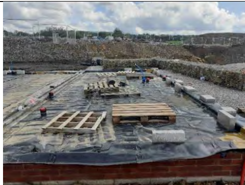
Plot 145: Membrane fully exposed except across cavity wall, Airbricks visible to front elevation
