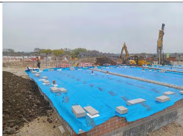
Plot 147: Membrane fully exposed and in good condition.
