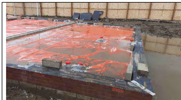
Plot 3: Membrane fully exposed except across cavity wall, despite some traffic marks and standing water is generally in good condition. Airbricks visible to front elevation
