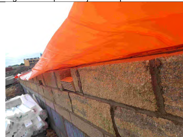
Plot 5: Membrane extends across outer wall
