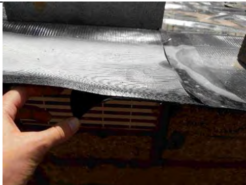
Plot 143: Overlap in membrane sheets to Gas resistant DPC >150mm and sealed with double and single sided tape.
