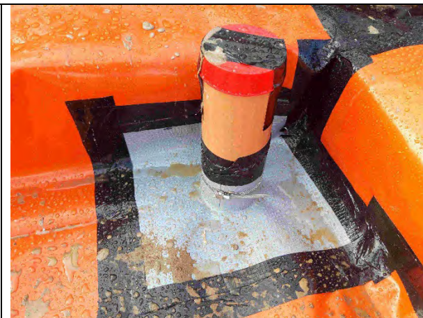
Plot 12: Service entry sealed with top hat, double and single sided tape and a jubilee clip
