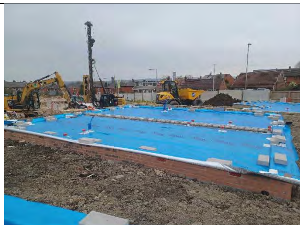
Plot 149: Membrane fully exposed and in good condition.
