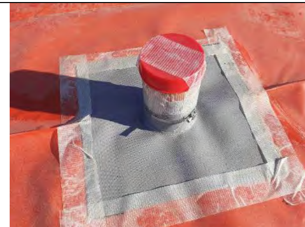
Plot 10: Service entry sealed with top hat, double and single sided tape and a jubilee clip
