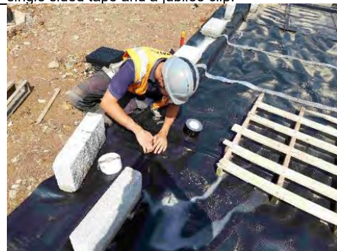
Plot 146: Single sided tape used to repair minor gaps in the geomembrane.
