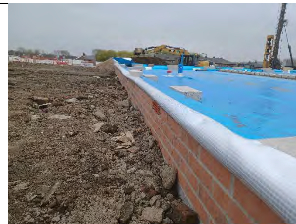
Plot 149: Membrane extends across outer cavity wall
