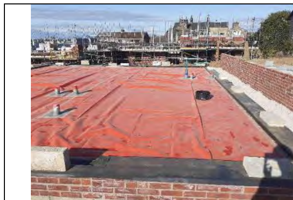
Plot 11: Membrane fully exposed and in good condition.
