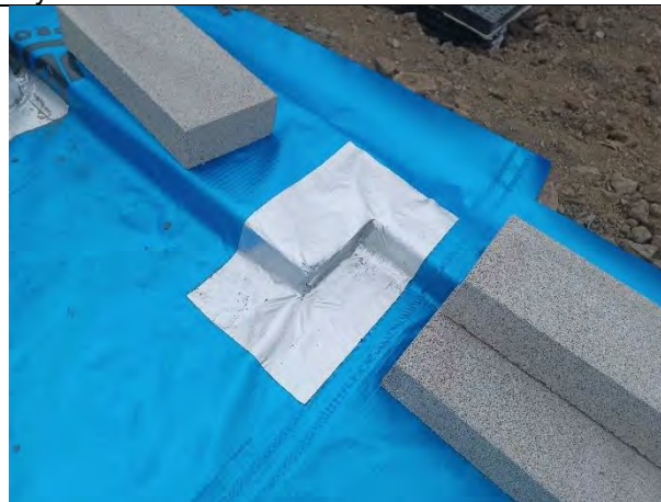
Plot 150: Good detail on cornering using proprietary detailing strip to reduce stress points.
