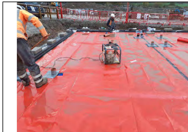
Plot 21: Membrane extends across plot footprint with all areas available for inspection. Standing water indicative of watertight seal achieved
