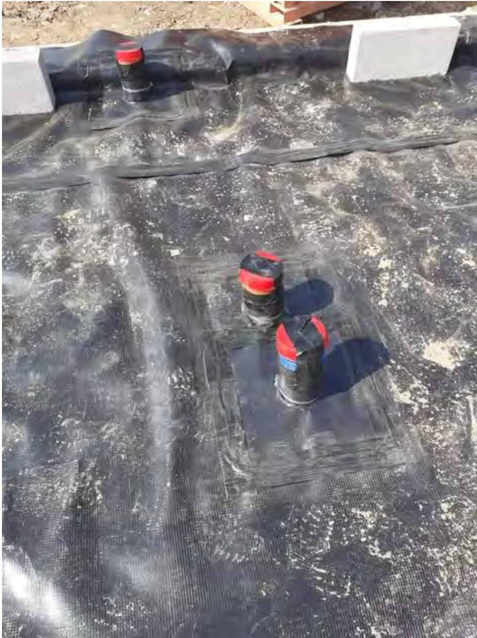
Barratt Bury: Site visit evidence:
