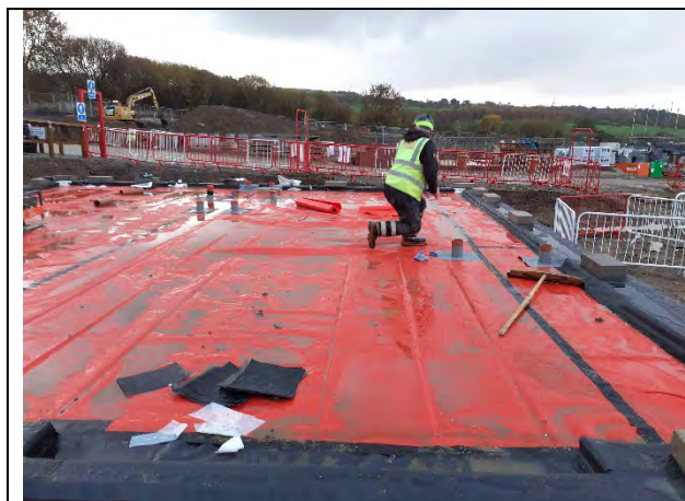
Plot 20: Membrane in good condition. Final taping of tap-hats taking place during inspection. Works complete during inspection
