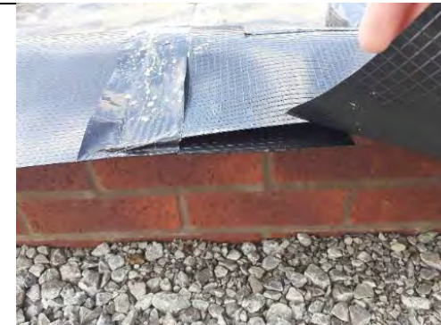
Plot 145: Overlap in membrane sheets to Gas resistant DPC >150mm and sealed with double and single sided tape.
