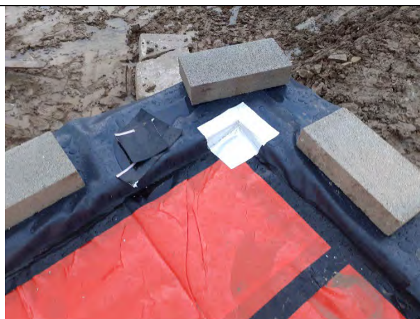
Plot 20: Good detail on cornering using proprietary detailing strip to reduce stress points; DPC taped to gas membrane extending to external wall.
