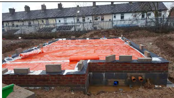
Plot 19: Membrane fully exposed and in good condition.
