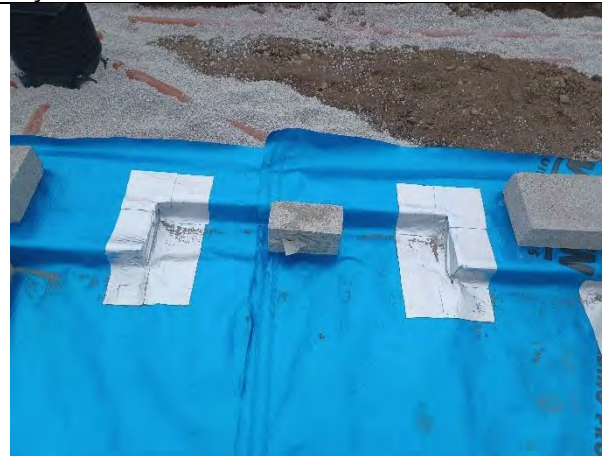
Plot 148: Good detail on cornering using proprietary detailing strip to reduce stress points.
