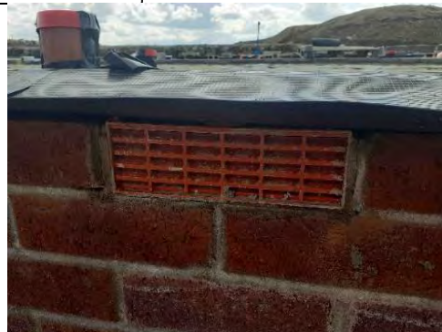
Plot 144: Airbricks installed were clear and free from any obstructions. Membrane extends across outer wall
