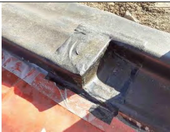
Plot 11: Good detail on cornering using proprietary detailing strip to reduce stress points.
