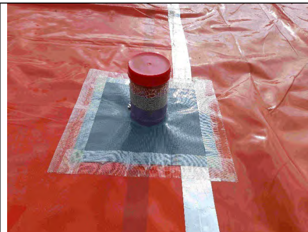
Plot 5: Service entry sealed with top hat, double and single sided tape and a jubilee clip.
