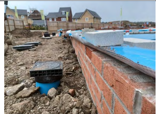
Plot 150: Membrane extends across outer cavity wall
