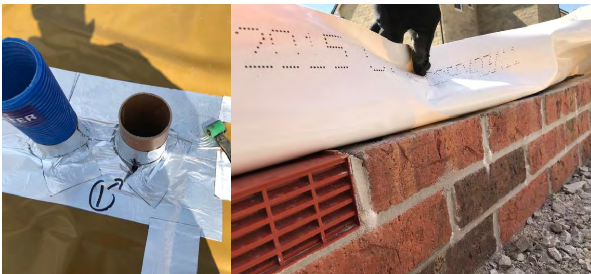
Pipe Penetrations - before repair
