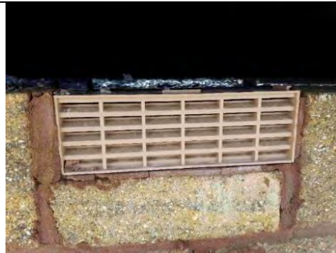
Plot 143: Airbricks installed were clear and free from any obstructions.
