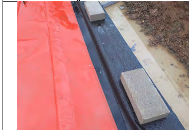
Plot 21: Good corner detailing with no stress points. DPC taped to membrane across cavity wall
