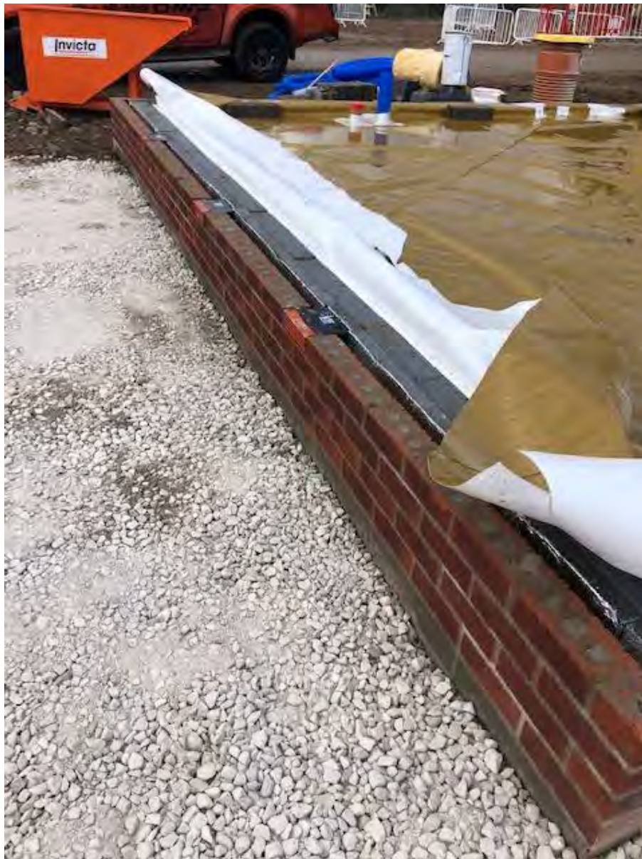
Barratt Bury Photograph 3: Showing line of edge air bricks, flow tested on the day.
