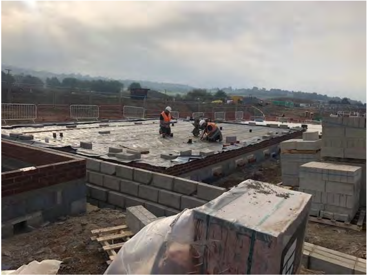
Barratt Bury Photograph 1: The plots as laid and being repaired.
