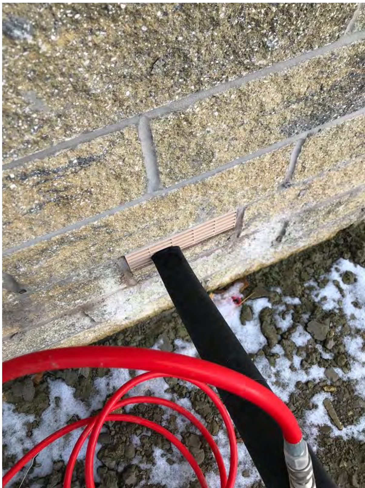
Figure 3 trace gas injection into sub-floor void.
