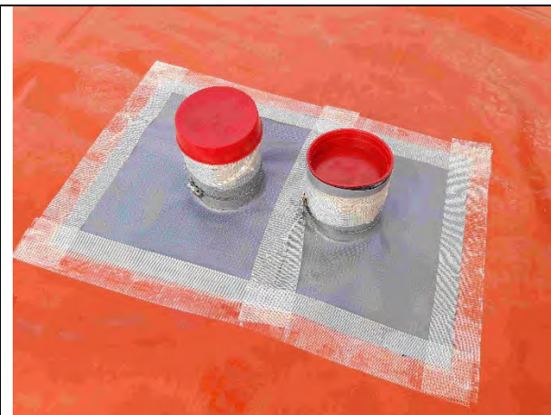
Plot 1: Service entry sealed with top hat, double and single sided tape and a jubilee clip
