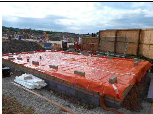
Plot 5: Membrane fully exposed and in good condition.
