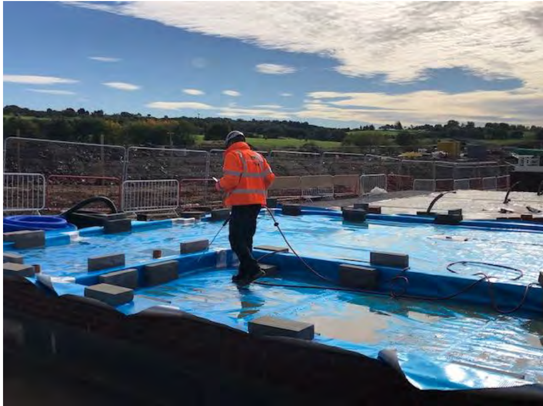
Barratt Bury Photograph 2: VISQUEEN GAS BARRIER Membrane:
