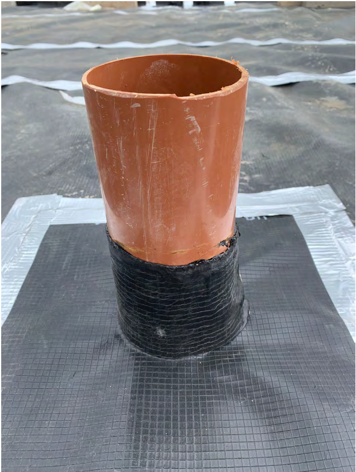
Barratt Bury Photograph 3: Example Penetration detail:
