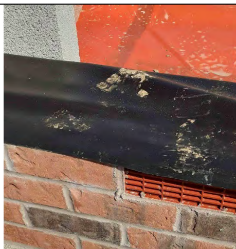
Plot 7: Airbricks installed were clear and free from any obstructions.
