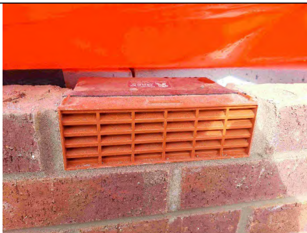
Plot 1: Airbricks installed were clear and free from any obstructions.
