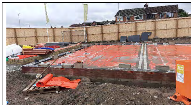
Plot 4: Membrane fully exposed except across cavity wall, despite some traffic marks and standing water is generally in good condition. Airbricks visible to front elevation
