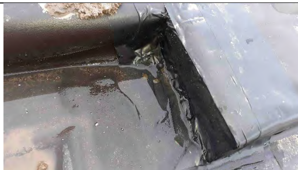
Plot 2: Good detail on cornering using proprietary detailing strip to reduce stress points.
