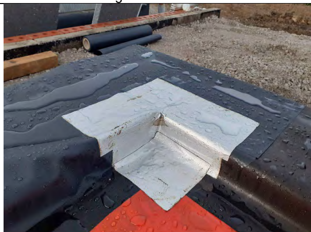
Plot 18: Good corner detailing with no stress points. DPC taped to membrane across cavity wall
