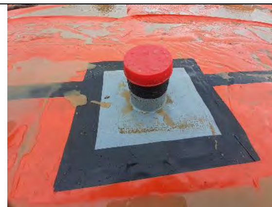
Plot 14: Service entry sealed with top hat, double and single sided tape and a jubilee clip under presence of JR,
