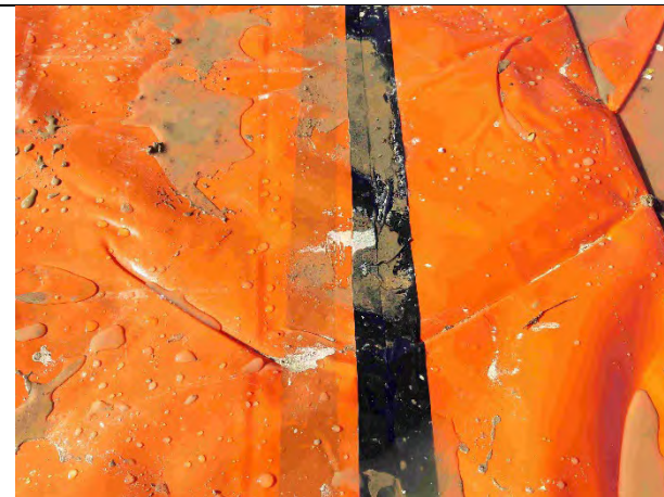
Plot 15: Overlap in membrane sheets >150mm and sealed with double and single sided tape
