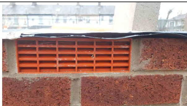
Plot 19: Airbricks installed were clear and free from any obstructions.
