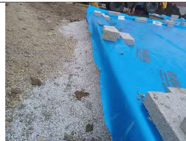
Plot 151: Membrane extends across outer cavity wall
