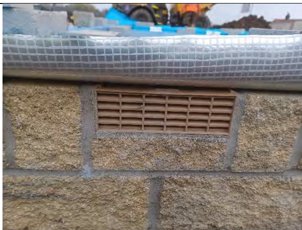
Plot 151: Airbricks installed were clear and free from any obstructions.
