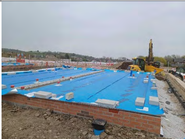
Plot 150: Membrane fully exposed and in good condition.
