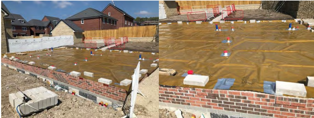
Pipe Penetrations - before repair
