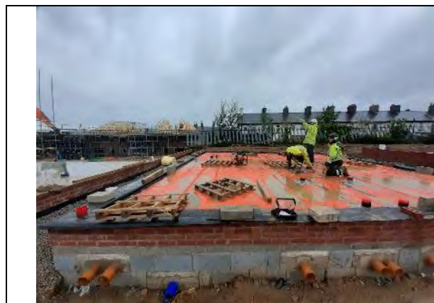
Plot 14: Membrane fully exposed and in good condition. Groundstaff sealing top hats whilst JR present, due to wet conditions.
