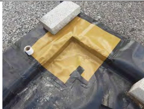
Plot 145: Corner detail, no holes visible in joints
