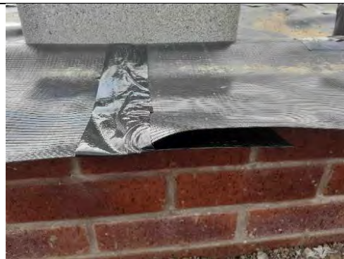
Plot 144: Membrane fully exposed except across cavity wall, Airbricks visible to front elevation
