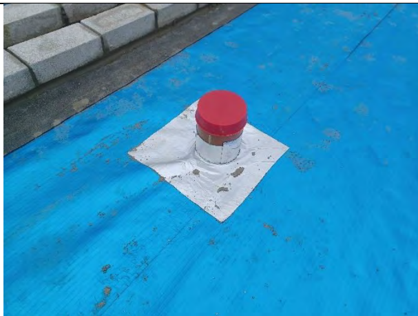
Plot 150: Service entry sealed using proprietary detailing strip
