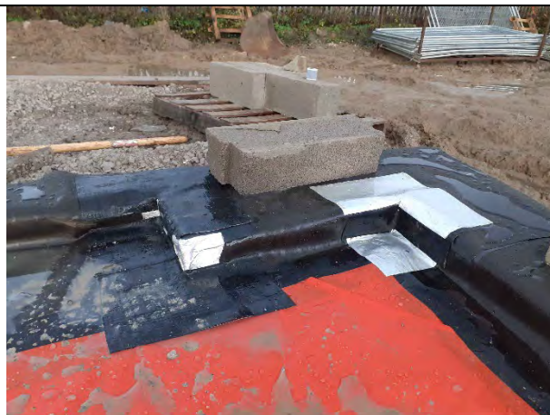
Plot 18: Good detail on cornering using proprietary detailing strip to reduce stress points; DPC taped to gas membrane extending to external wall
