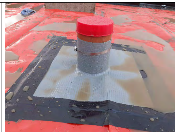
Plot 20: Service entry sealed with top hat, double and single sided tape and a jubilee clip
