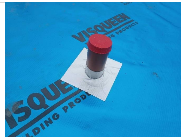
Plot 147: Service entry sealed using proprietary detailing strip
