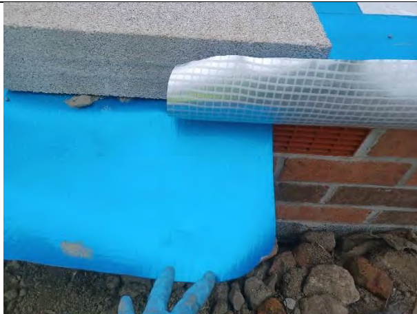
Plot 148: Overlap in membrane sheets >150mm and sealed with heat gun.
