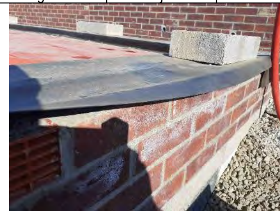
Plot 11: DPC taped to membrane and extends across outer cavity wall
