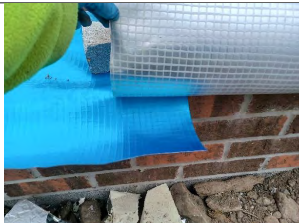
Plot 147: Overlap in membrane sheets >150mm and sealed with heat gun
