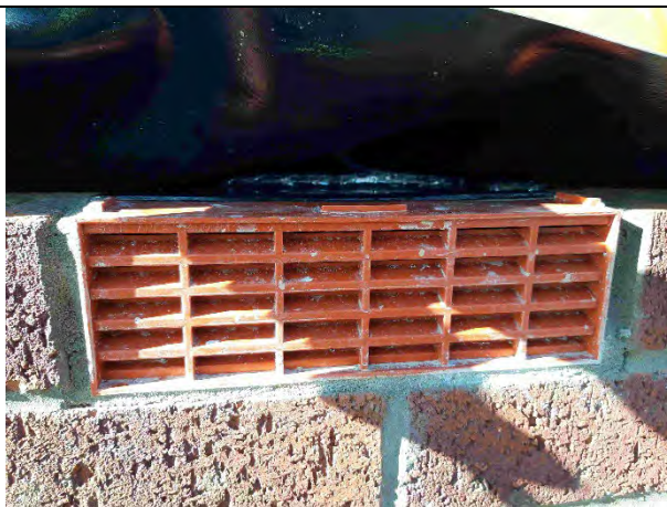
Plot 15: Airbricks installed were clear and free from any obstructions.
