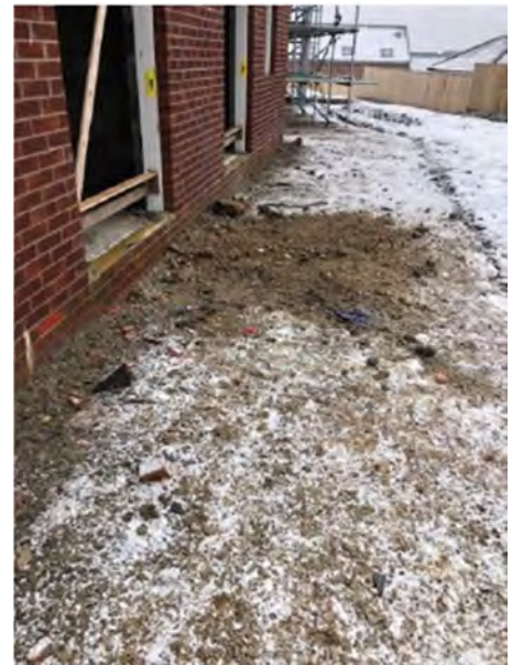
Monitoring location temporarily backfilled to avoid destruction during site works
