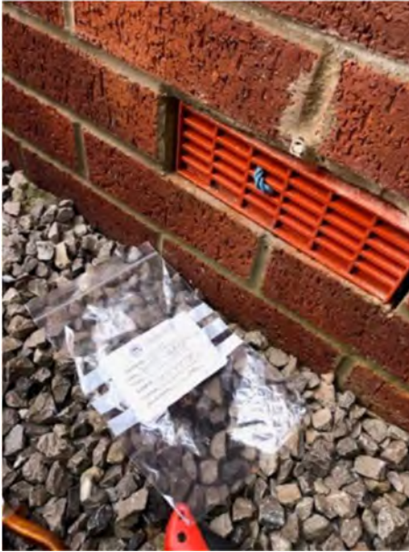
Plot 48 sub-floor void monitoring.
