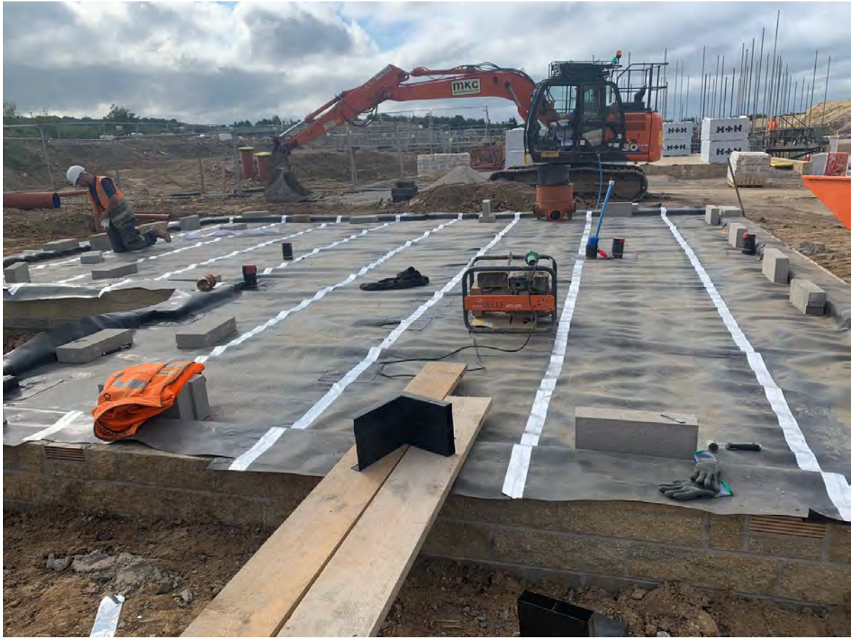
Barratt Bury Photograph 2: General area view (taped seams with silver foil tape):
