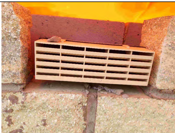
Plot 5: Airbricks installed were clear and free from any obstructions.
