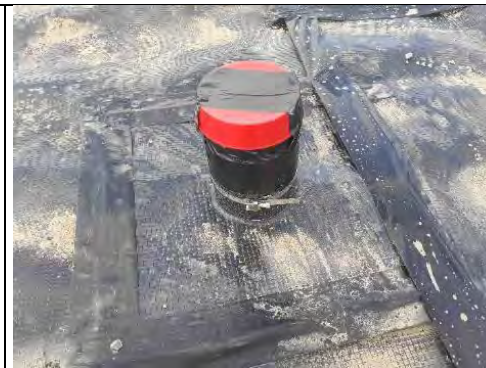
Plot 144: Service entry sealed with top hat, double and single sided tape and a jubilee clip.
