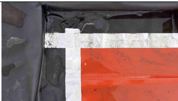
Plot 2: Overlap in membrane sheets to Gas resistant DPC >150mm and sealed with double and single sided tape.
