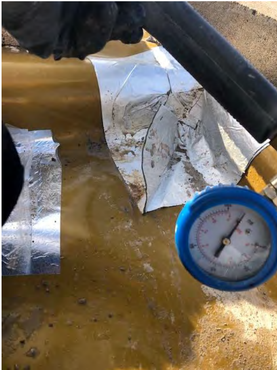
Photo 3: Barratts Bury: Corner and Penetration detailing: 31.1.22
