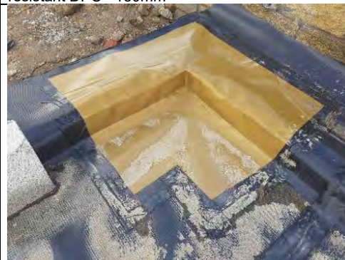
Plot 146: Corner detail, no holes visible in joints
