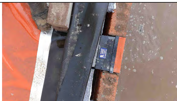
Plot 2: Airbricks installed were clear and free from any obstructions. Membrane extends across outer wall
