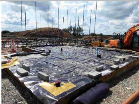
Plot 143: Membrane fully exposed and in good condition.
