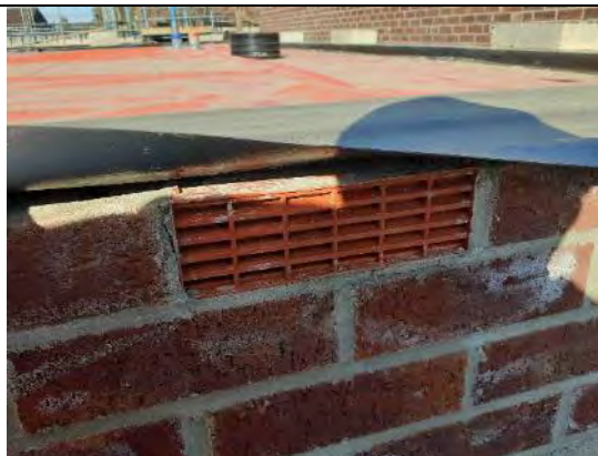
Plot 11: Airbricks installed were clear and free from any obstructions.
