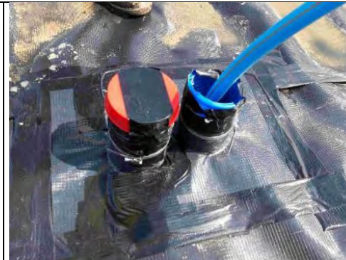
Plot 143: Service entry sealed with top hat, double and single sided tape and a jubilee clip
