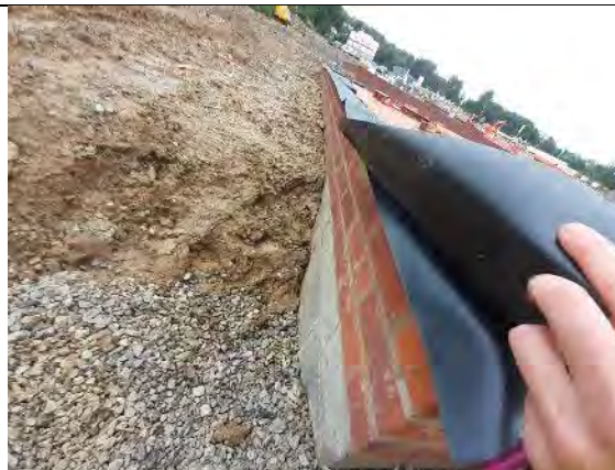
Plot 14: DPC taped to membrane and extends across outer cavity wall
