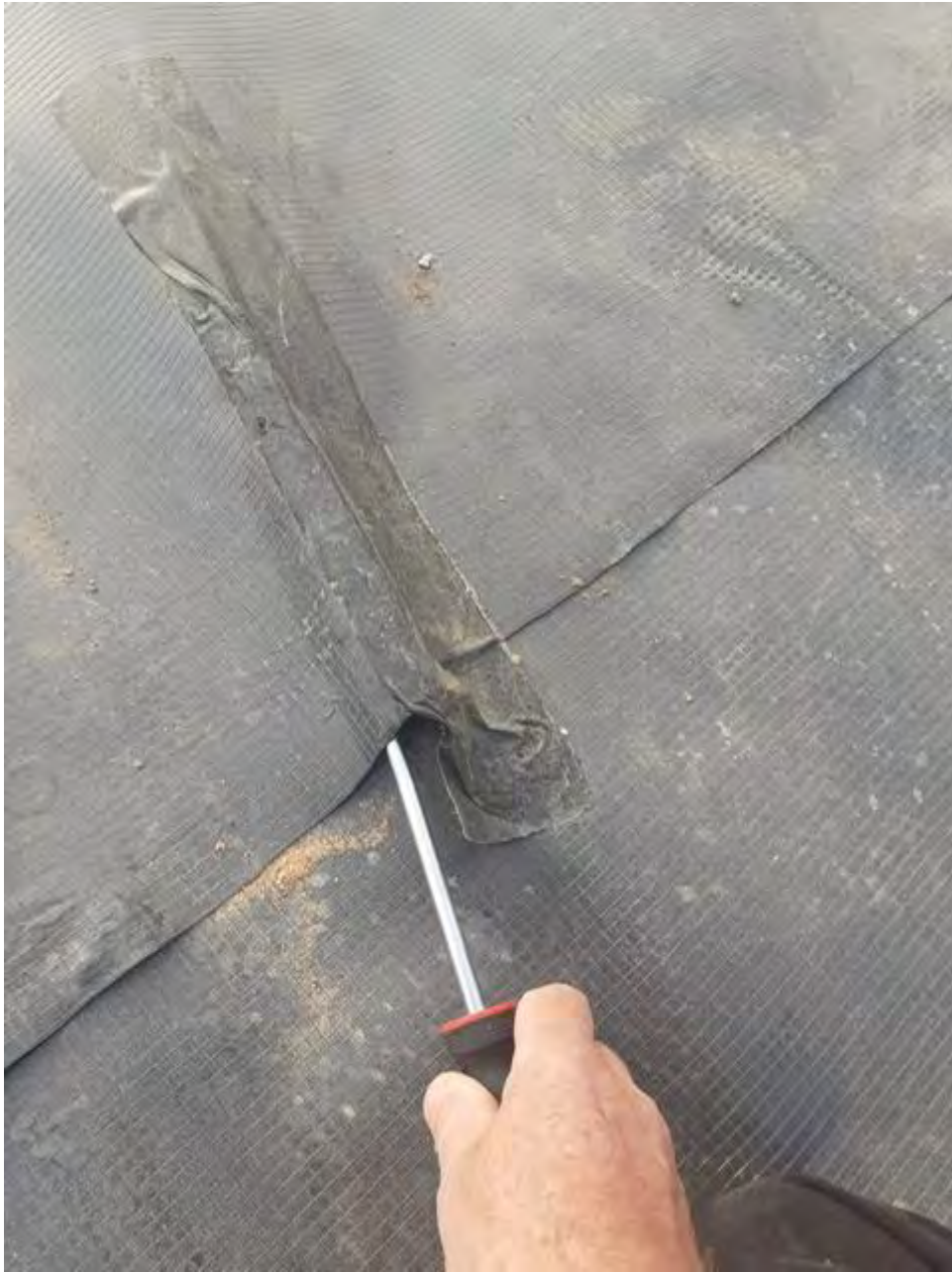
Barratt Bury Photograph 1: Repair made to seam.
