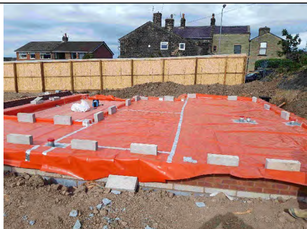
Plot 1: Membrane fully exposed and in good condition.
