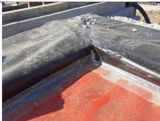
Plot 10: Good detail on cornering using proprietary detailing strip to reduce stress points.
