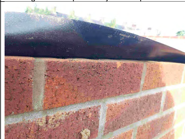
Plot 12: Membrane extends across outer wall
