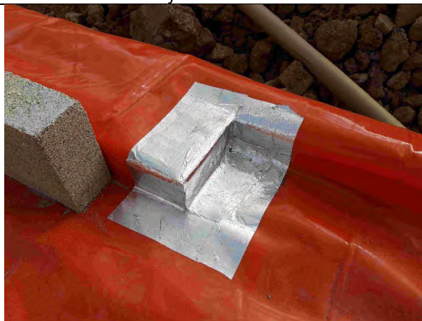
Plot 5: Good detail on cornering using proprietary detailing strip to reduce stress points.
