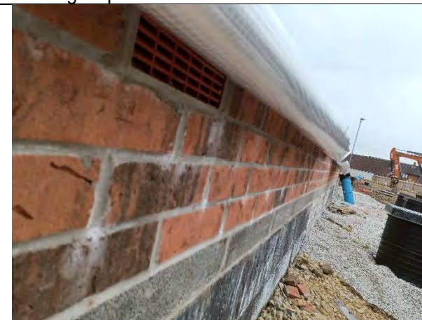
Plot 147: Membrane extends across outer cavity wall
