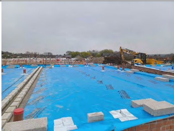
Plot 148: Membrane fully exposed and in good condition.
