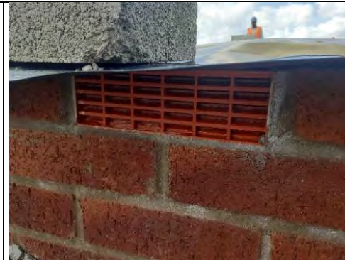
Plot 145: Airbricks installed were clear and free from any obstructions.
