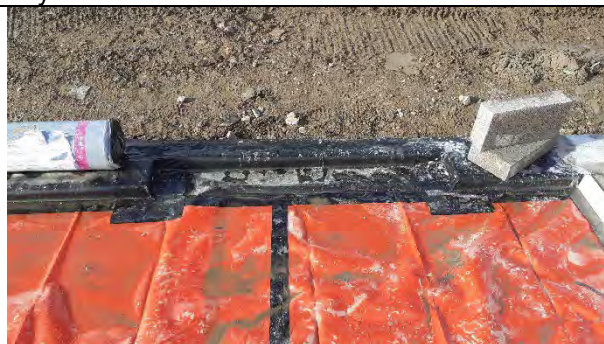
Plot 16: Good detail on cornering using proprietary detailing strip to reduce stress points; DPC taped to gas membrane extending to external wall.
