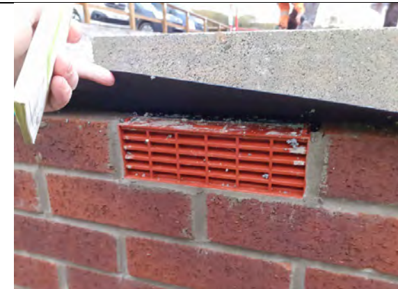
Plot 21: Airbricks installed were clear and free from any obstructions.
