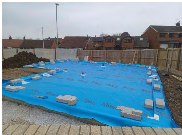
Plot 151: Membrane fully exposed and in good condition.
