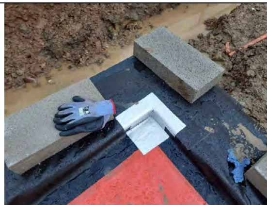
Plot 21: Good detail on cornering using proprietary detailing strip to reduce stress points; DPC taped to gas membrane extending to external wall
