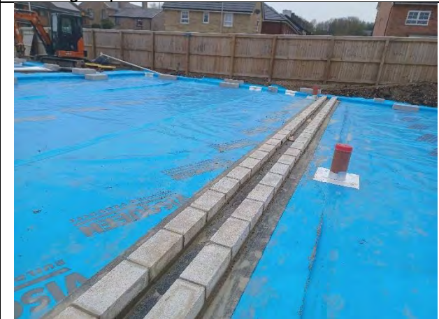
Plot 148: Membrane spans neatly under internal dividing wall between plots
