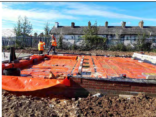
Plot 15: Membrane fully exposed and in good condition.
