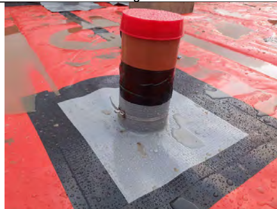
Plot 21: Service entry sealed with top hat, double and single sided tape and a jubilee clip
