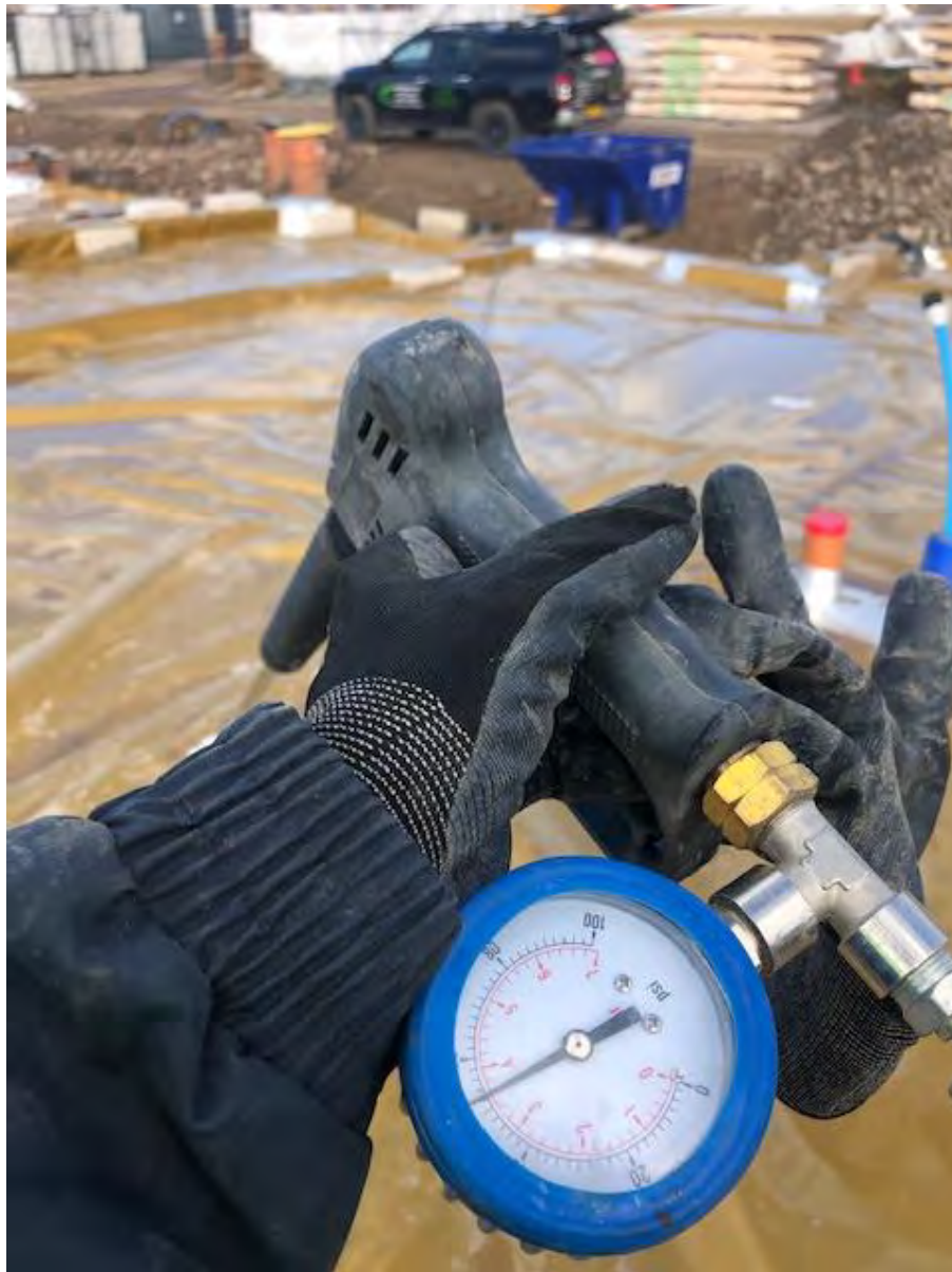
Barratt Bury Photograph 2: Air Lance Pressure Evidence: 31.1.22
