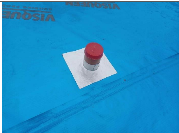
Plot 151: Service entry sealed with top hat, and adhesive membrane patches
