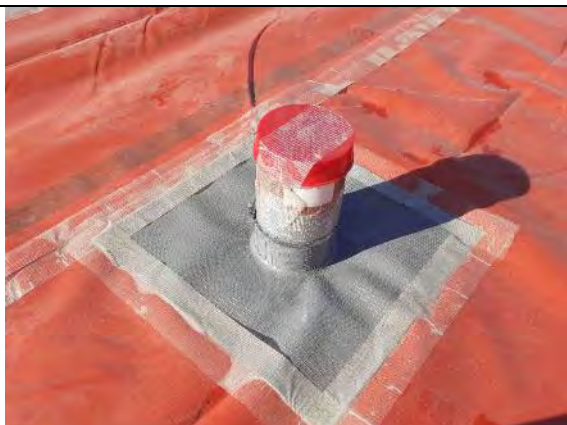
Plot 11: Overlap in membrane sheets >150mm and sealed with double and single sided tape. Service entry neatly sealed and tightened with jubilee clip.
