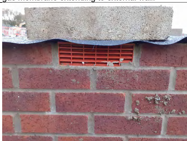
Plot 20: Airbricks installed were clear and free from any obstructions.
