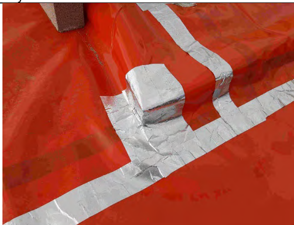
Plot 1: Good detail on cornering using proprietary detailing strip to reduce stress points.
