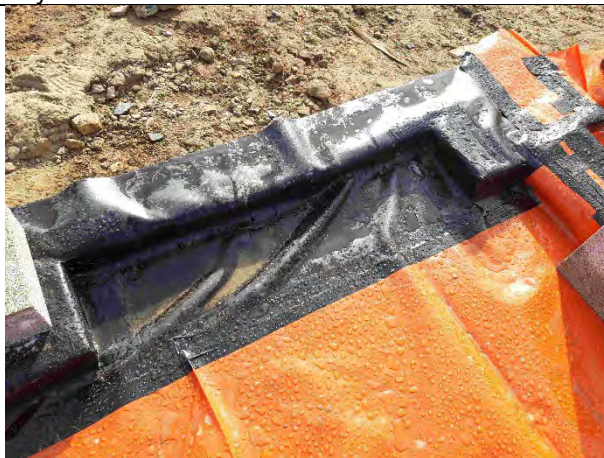
Plot 12: Good detail on cornering using proprietary detailing strip to reduce stress points.
