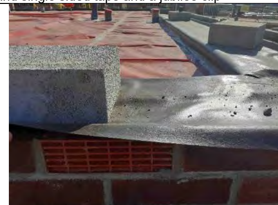
Plot 10: DPC taped to membrane and extends across outer cavity wall
