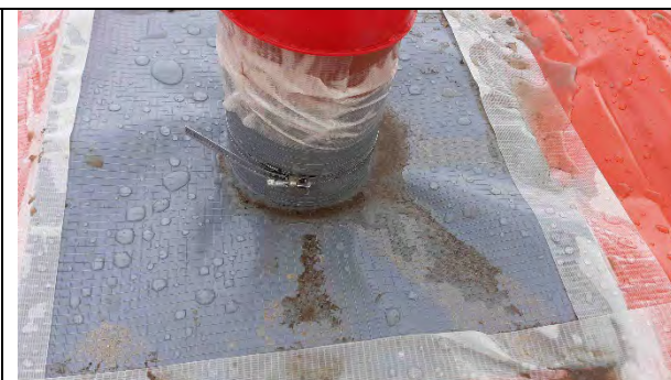
Plot 3 Service entry sealed with top hat, double and single sided tape and a jubilee clip.
