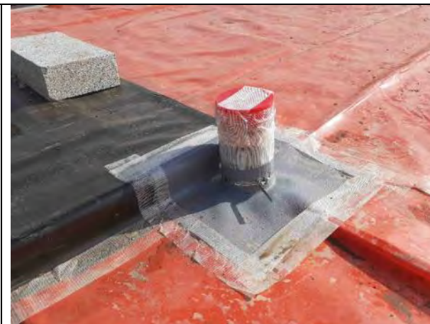
Plot 9: Service entry sealed with top hat, double and single sided tape and a jubilee clip
