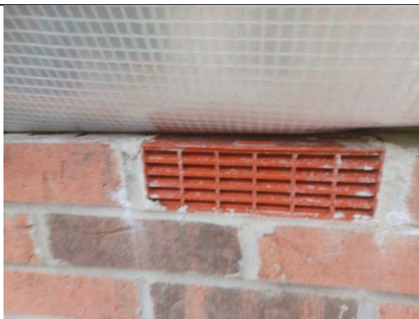
Plot 147: Airbricks installed were clear and free from any obstructions.
