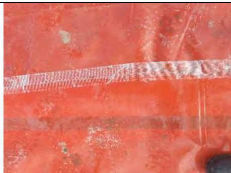
Plot 9: Overlap in membrane sheets >150mm and sealed with double and single sided tape
