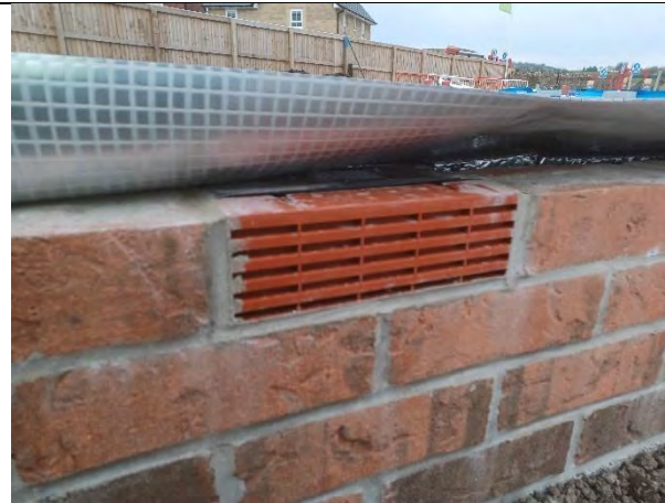
Plot 148: Airbricks installed were clear and free from any obstructions.
