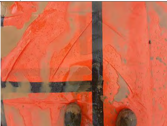
Plot 14: Overlap in membrane sheets >150mm and sealed with double and single sided tape. Service entry neatly sealed and tightened with jubilee clip.
