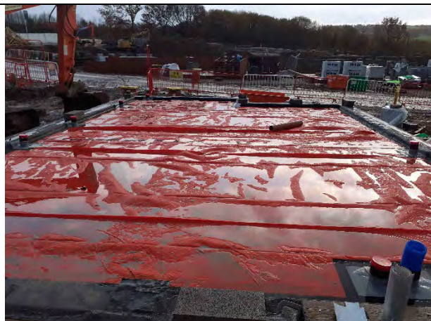
Plot 18: Membrane extends across plot footprint with all areas available for inspection. Standing water indicative of watertight seal achieved
