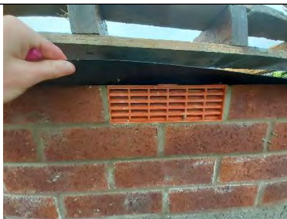
Plot 14: Airbricks installed were clear and free from any obstructions.
