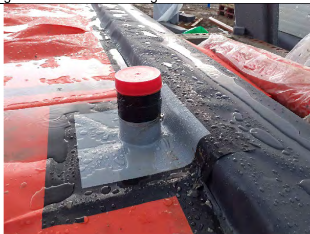
Plot 18: Service entry sealed with top hat, double and single sided tape and a jubilee clip
