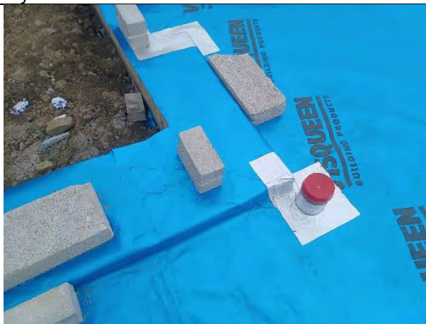
Plot 151: Good detail on cornering using proprietary detailing strip to reduce stress points.
