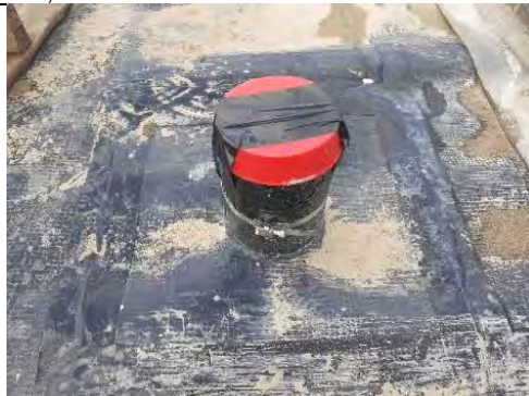
Plot 145: Service entry sealed with top hat, double and single sided tape and a jubilee clip.
