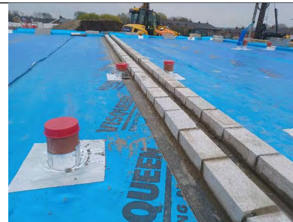
Plot 149: Membrane spans neatly under internal dividing wall between plots
