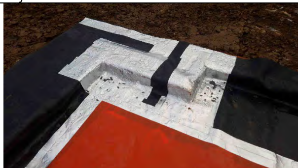
Plot 19: Good detail on cornering using proprietary detailing strip to reduce stress points; DPC taped to gas membrane extending to external wall.
