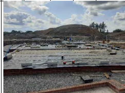
Plot 144: Membrane fully exposed and in good condition.
