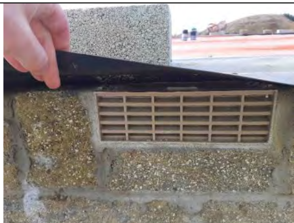
Plot 9: Airbricks installed were clear and free from any obstructions.
