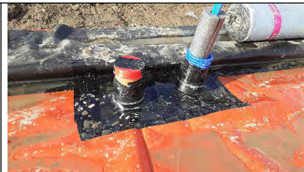
Plot 16: Service entries sealed with top hat, double and single sided tape and a jubilee clip
