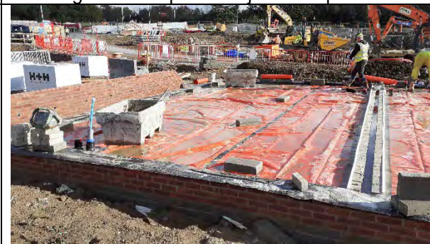
Plot 17: Membrane fully exposed and in good condition.
