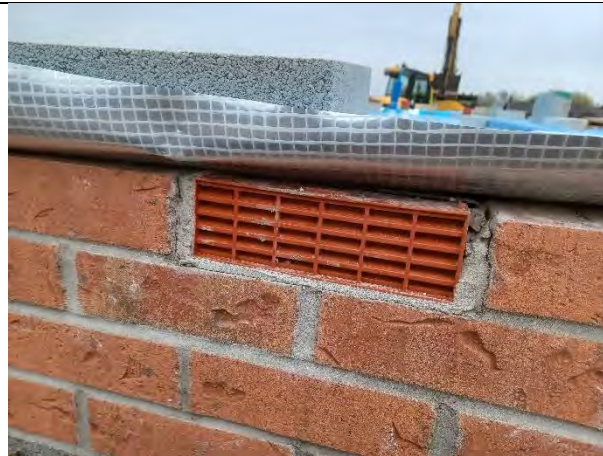
Plot 150: Airbricks installed were clear and free from any obstructions.
