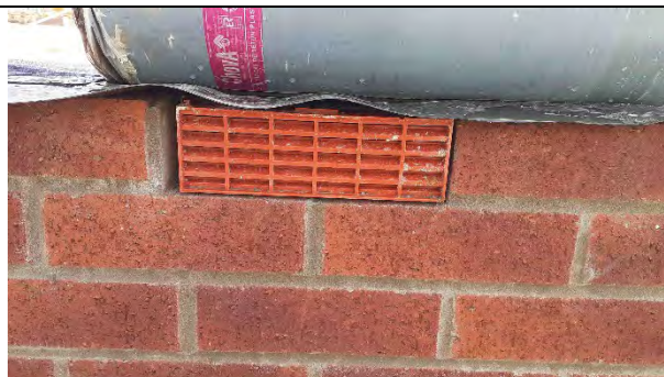
Plot 16: Airbricks installed were clear and free from any obstructions.
