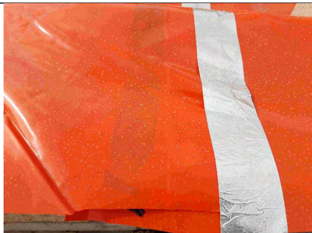
Plot 5: Overlap in membrane sheets >150mm and sealed with double and single sided tape.
