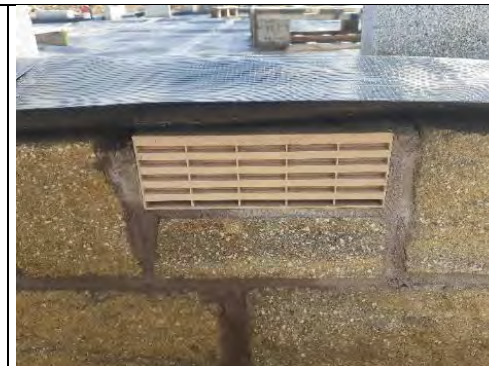
Plot 146: Airbricks installed were clear and free from any obstructions.
