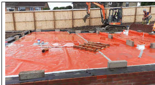
Plot 2: Membrane fully exposed and in good condition.
