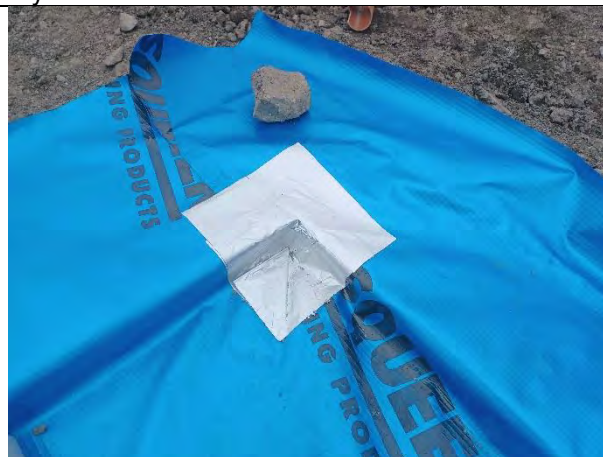
Plot 149: Good detail on cornering using proprietary detailing strip to reduce stress points.
