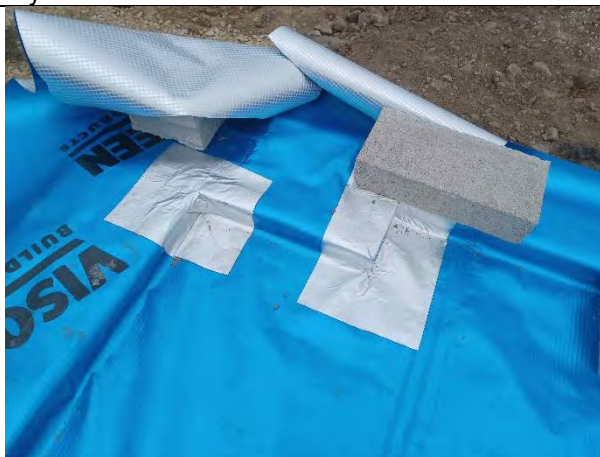
Plot 147: Good detail on cornering using proprietary detailing strip to reduce stress points.
