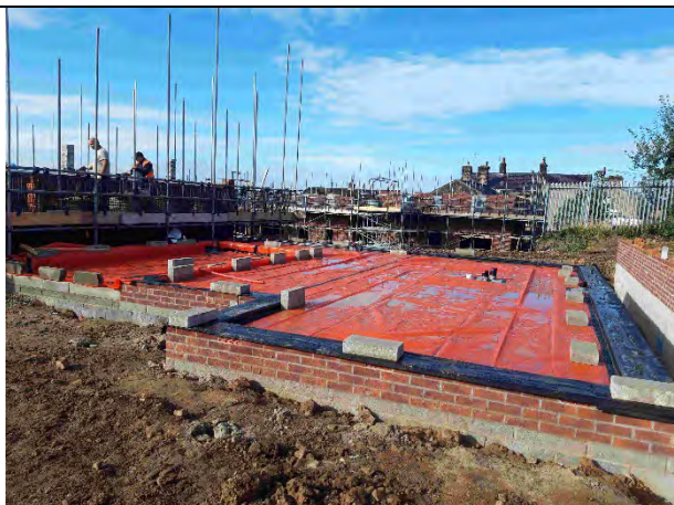
Plot 12: Membrane fully exposed and in good condition.
