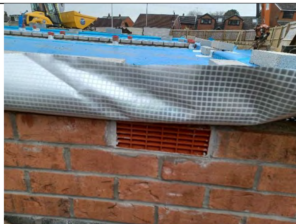
Plot 149: Airbricks installed were clear and free from any obstructions.
