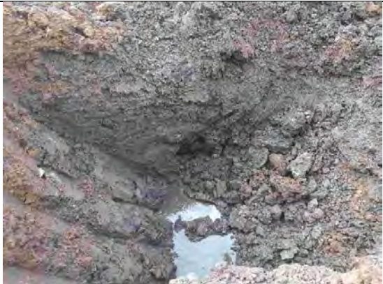
Base of excavation at 2.5-3.0m
