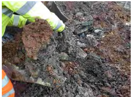
Boundary between natural clay (excavated) and underlying Rough Rock (excavated to competent rockhead)
