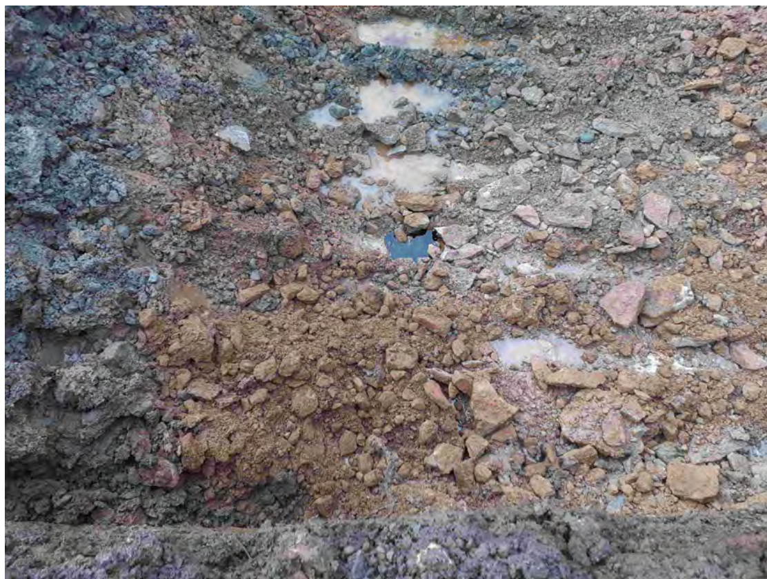
Figure 4.1: 'HS11' Photograph showing localised product with groundwater ingress
