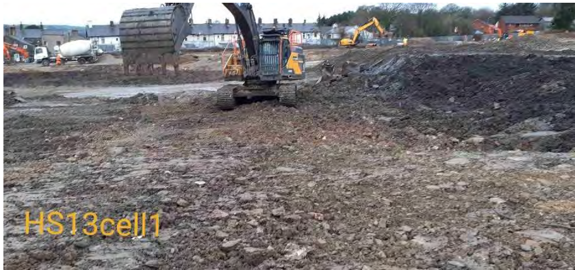
General view before excavation
