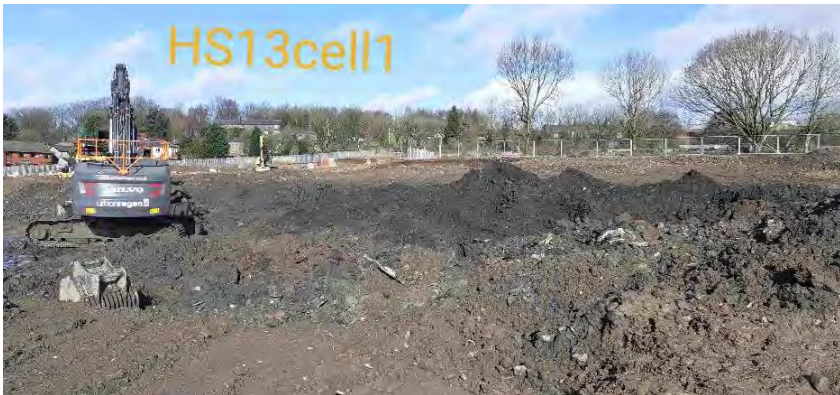
General view after excavation
