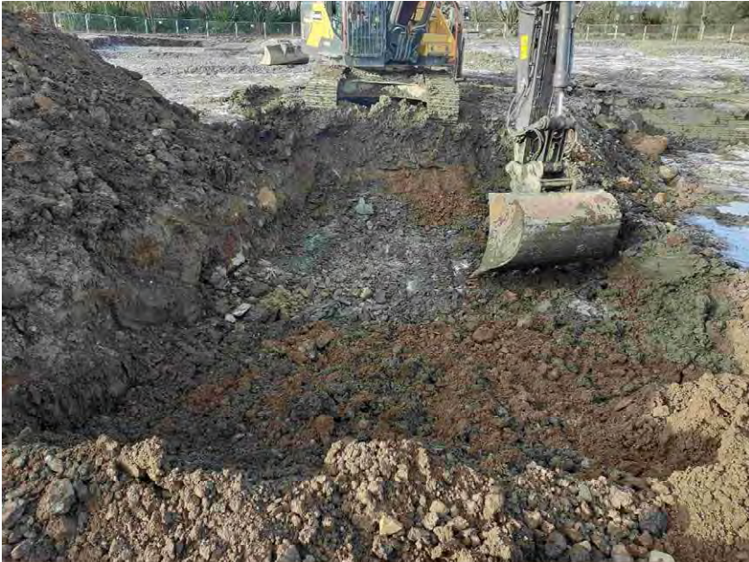
General view north over Cell
