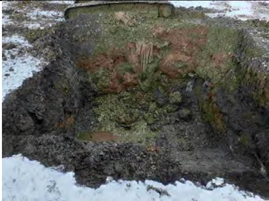
Initial dig in south side
