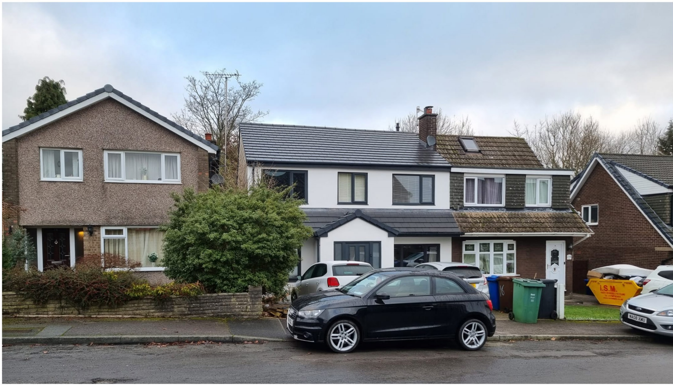
As-built Precedent Property #P2 - 16 Sheep Gate
