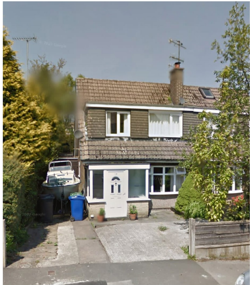
Original Precedent Property #P2 - 16 Sheep Gate Drive
