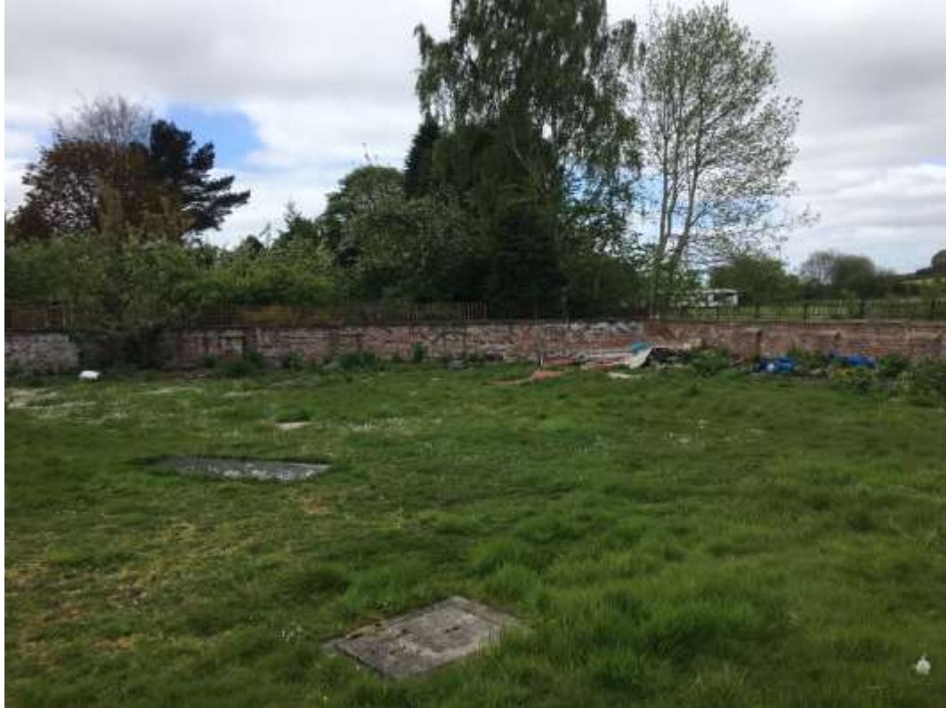
Photograph 5: View northwest across the garden area, note former demolished structure in the background and service cover in the foreground
