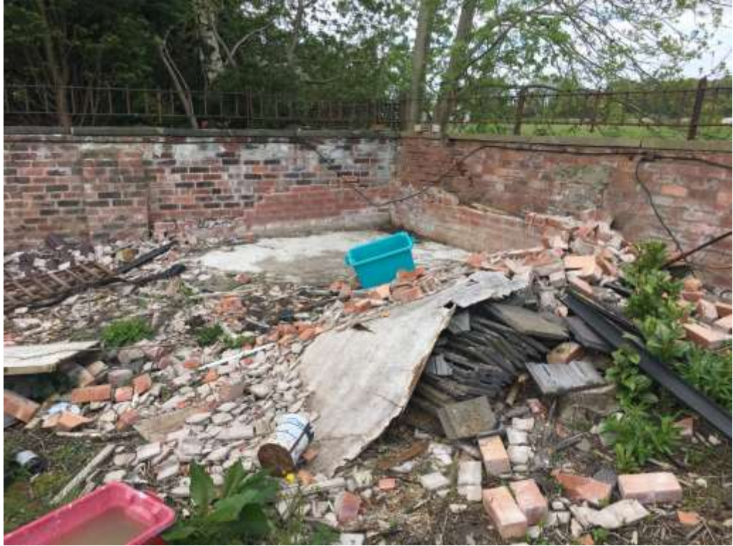
Photograph 6: Close up view of demolished structure in the northwest corner of the site
