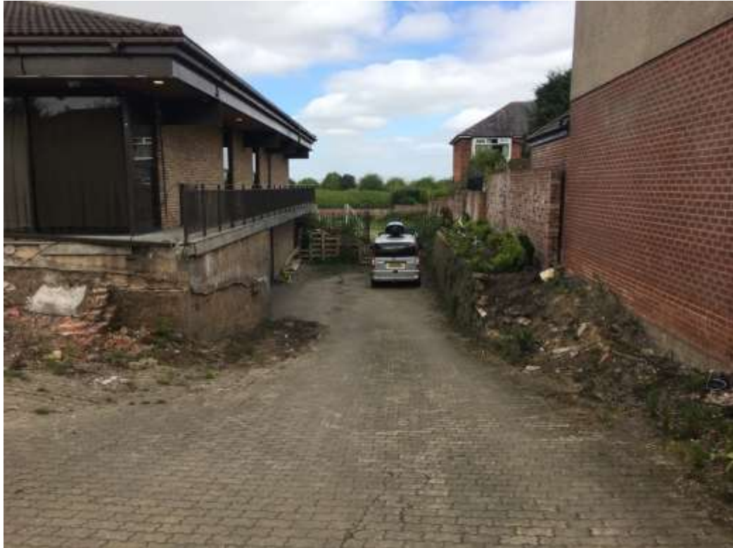
Photograph 1: View northwest – Along eastern side of the existing property
