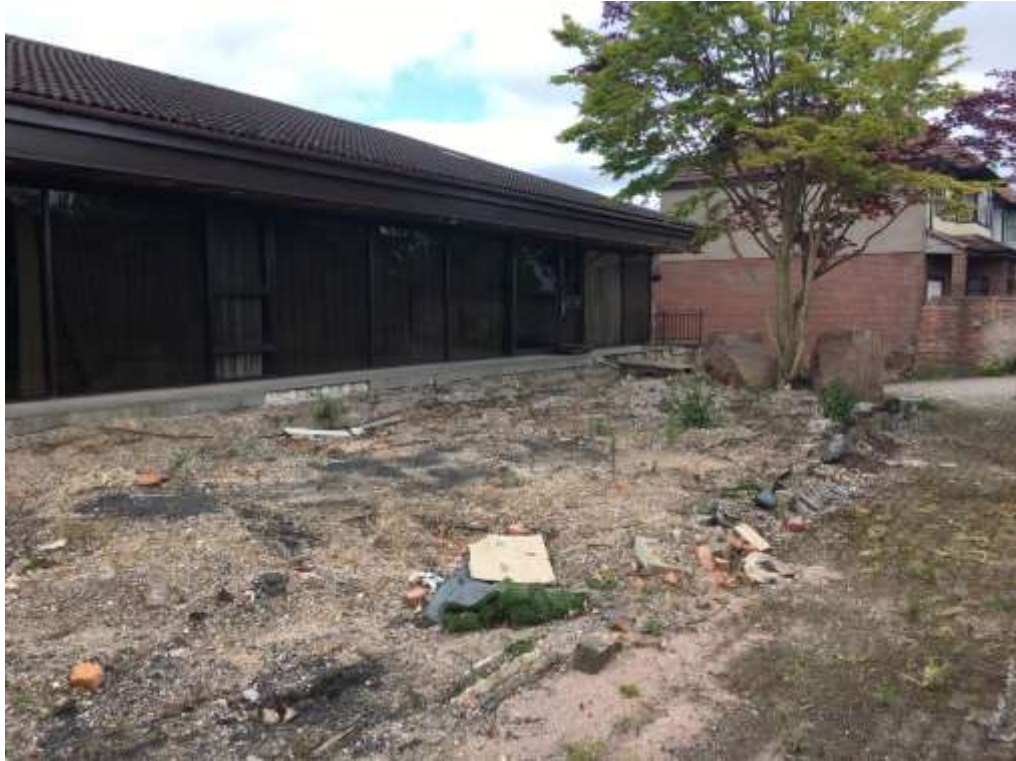
Photograph 3: View northeast along the front /southern side of the exiting property showing the area where the trees once were
