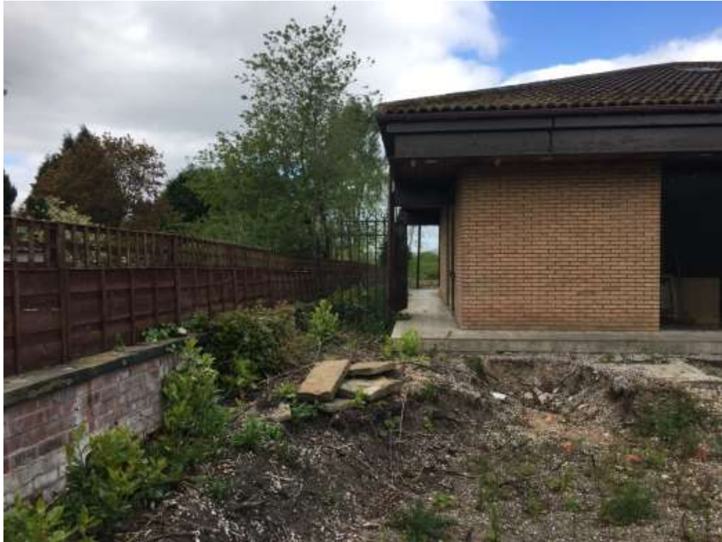
Photograph 2: View northwest – Along western side of the existing property
