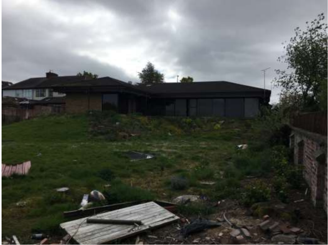
Photograph 8: General view south from northwest corner of the site showing existing property
