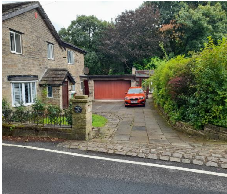
Existing site access from Bass Lane with Garage to rear
