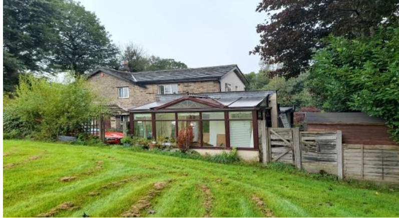
View from east of the to-be demolished conservatory
