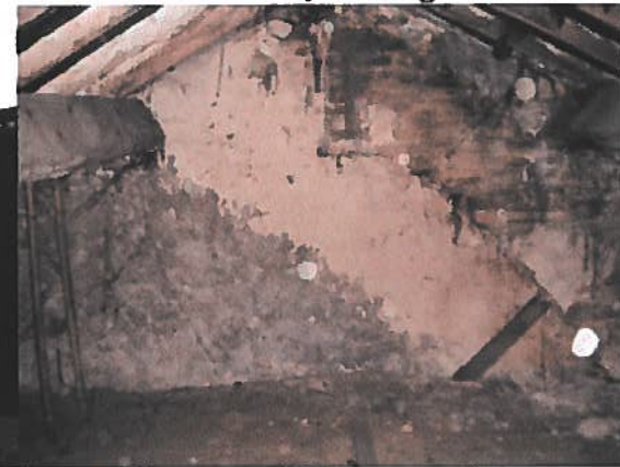
P8, House loft, building 2
