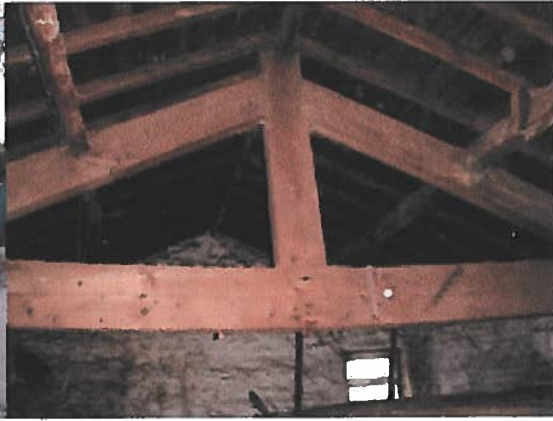
P6 Plank-lined roof, building 6
