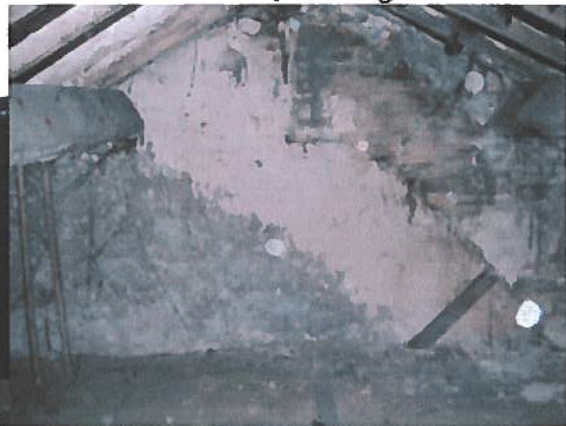
P8, House loft, building 2
