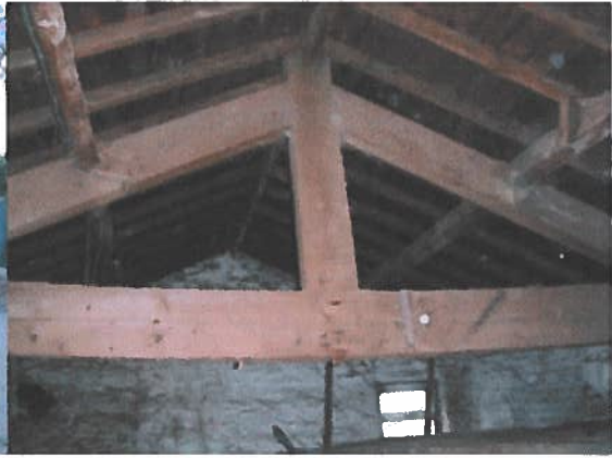
P6 Plank-lined roof, building 6
