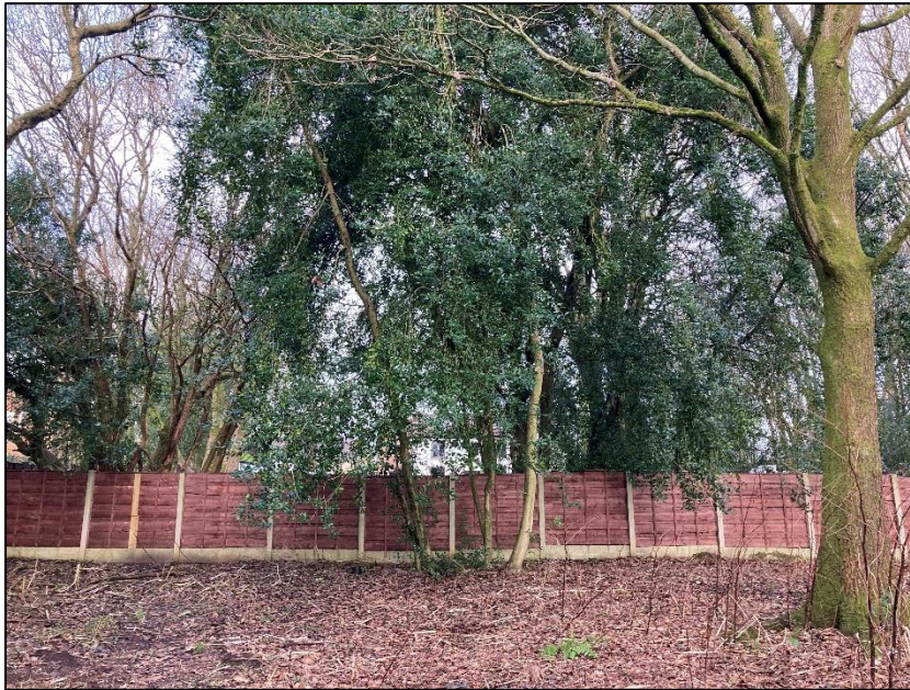
Photograph 8 showing the panel fencing
