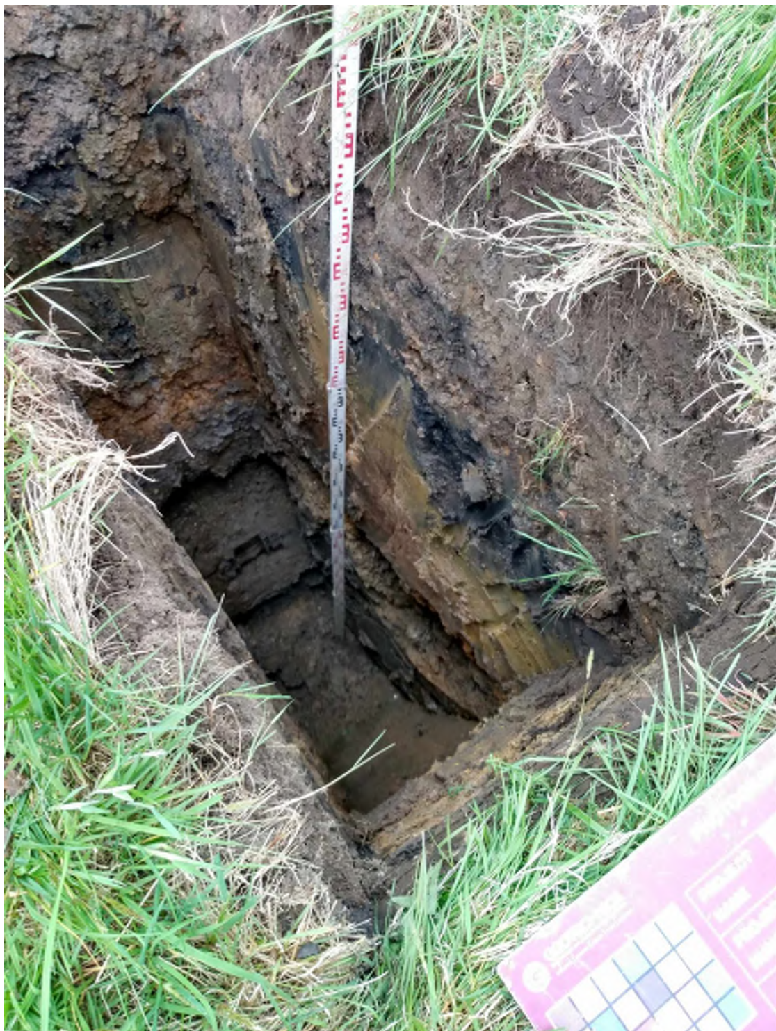
Machine-dug Trial Pit TP05 (2)
