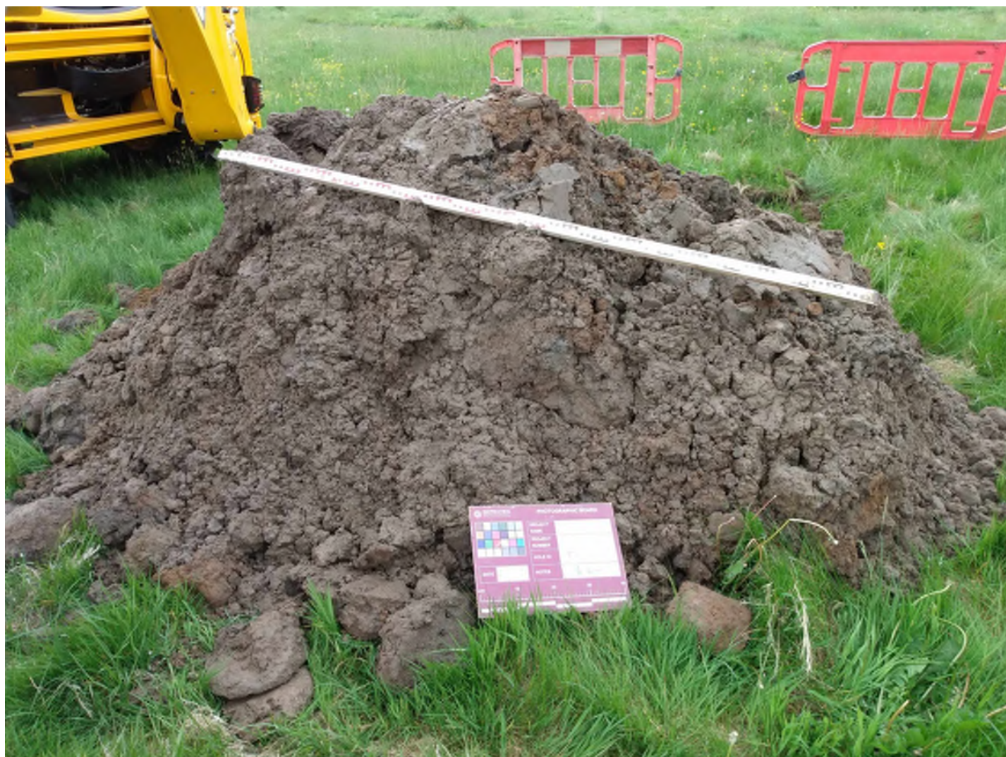
Machine-dug Trial Pit TP04 (3) Arisings
