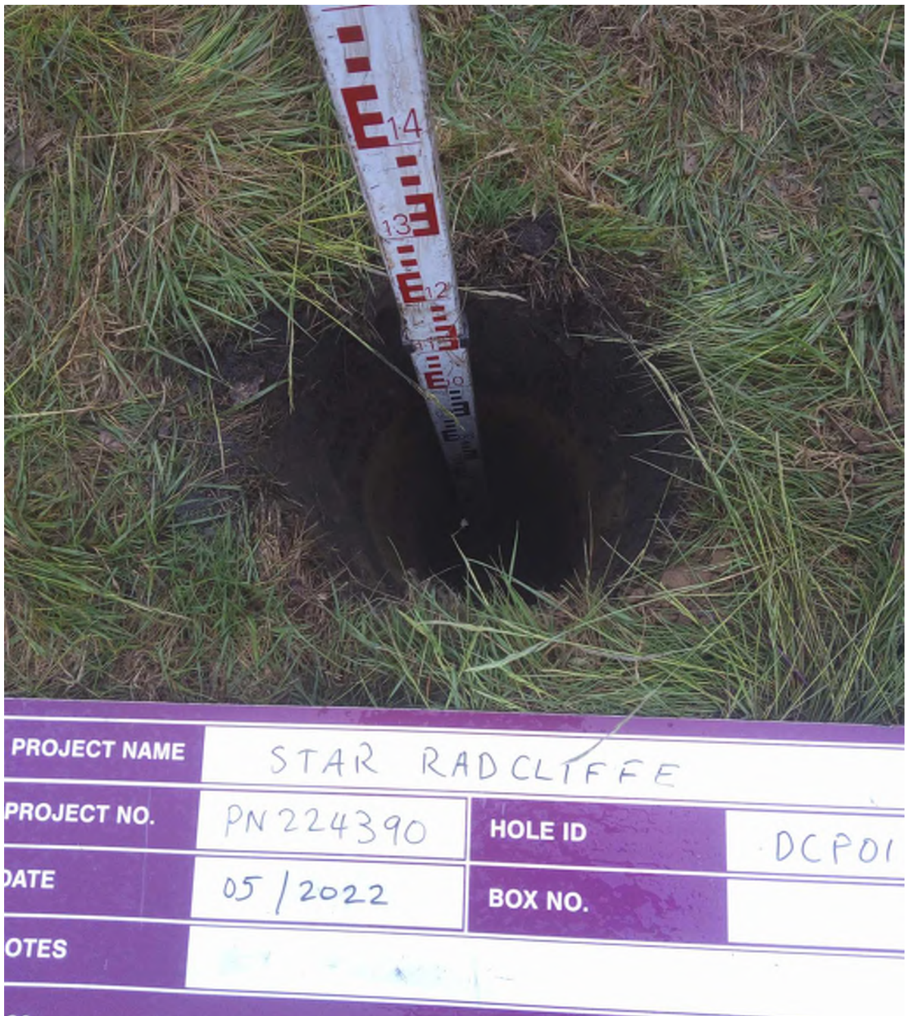
Hand-dug Trial Pit DCP01
