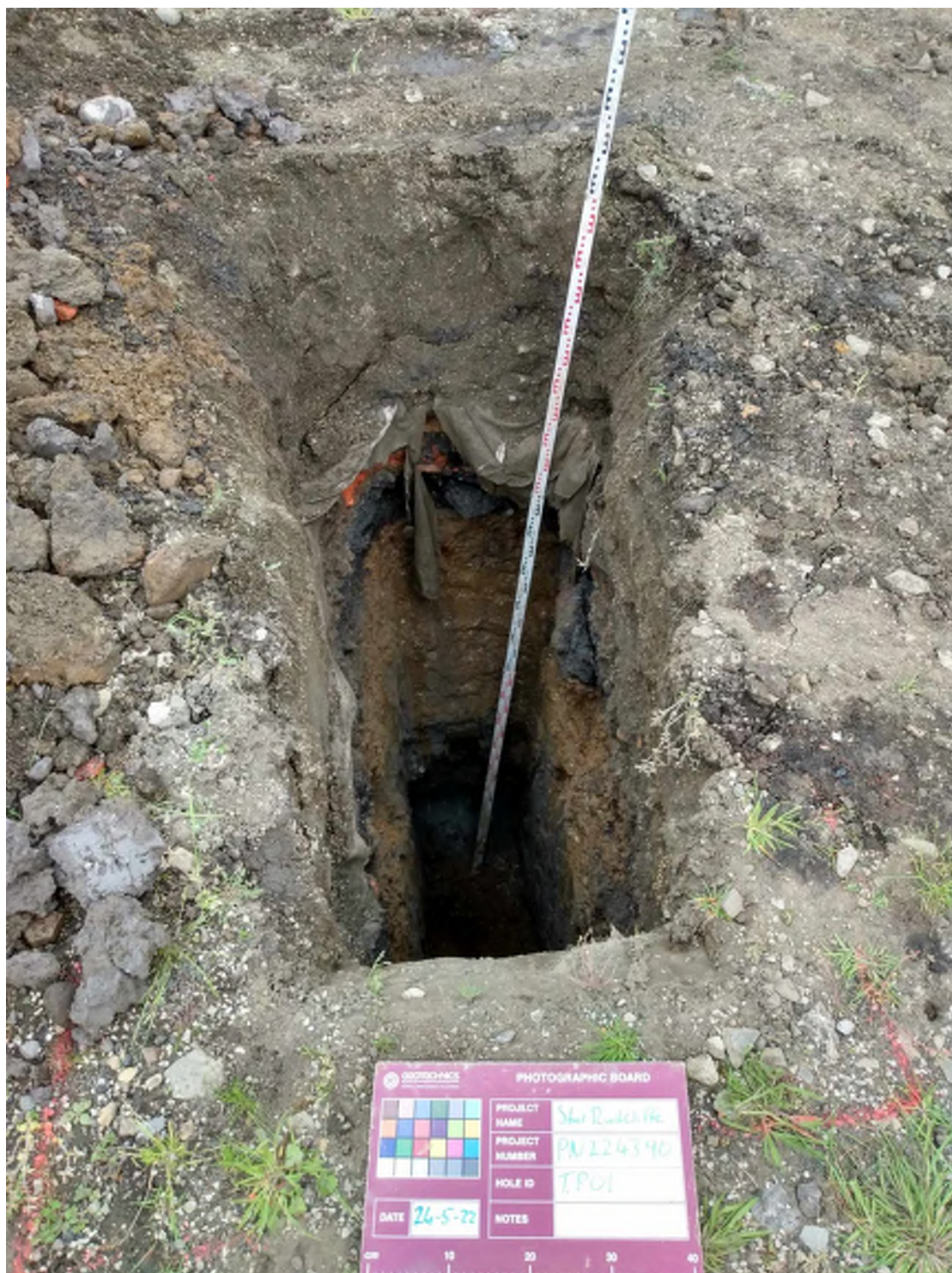
Machine-dug Trial Pit TP01 (4)
