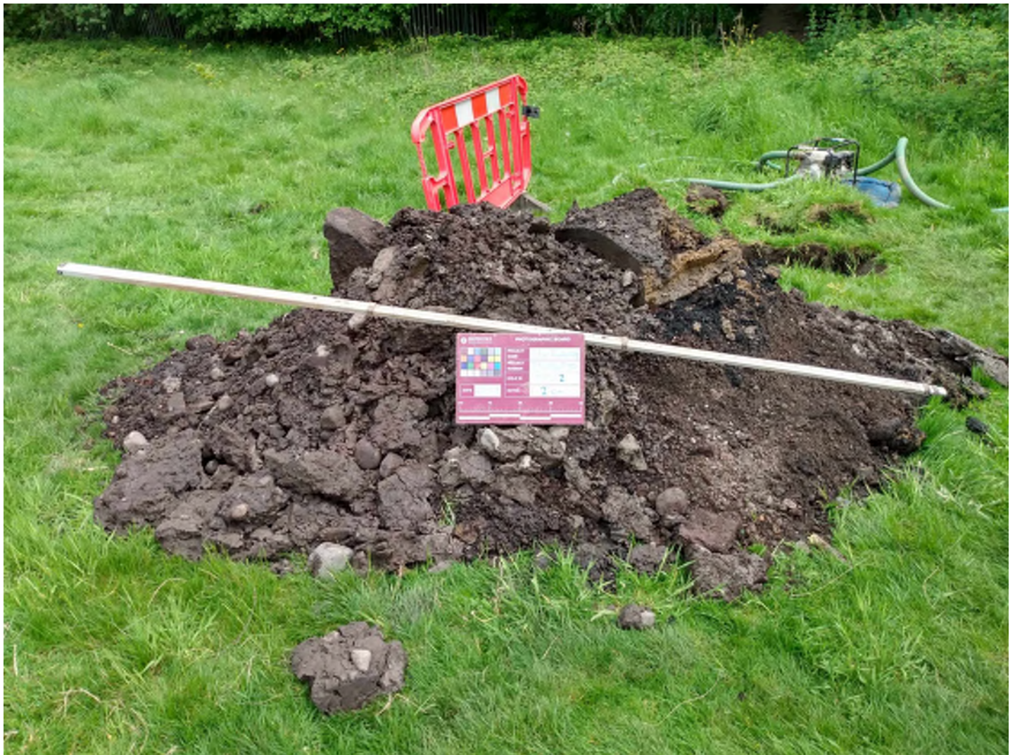
Machine-dug Trial Pit TP02 (2) Arisings
