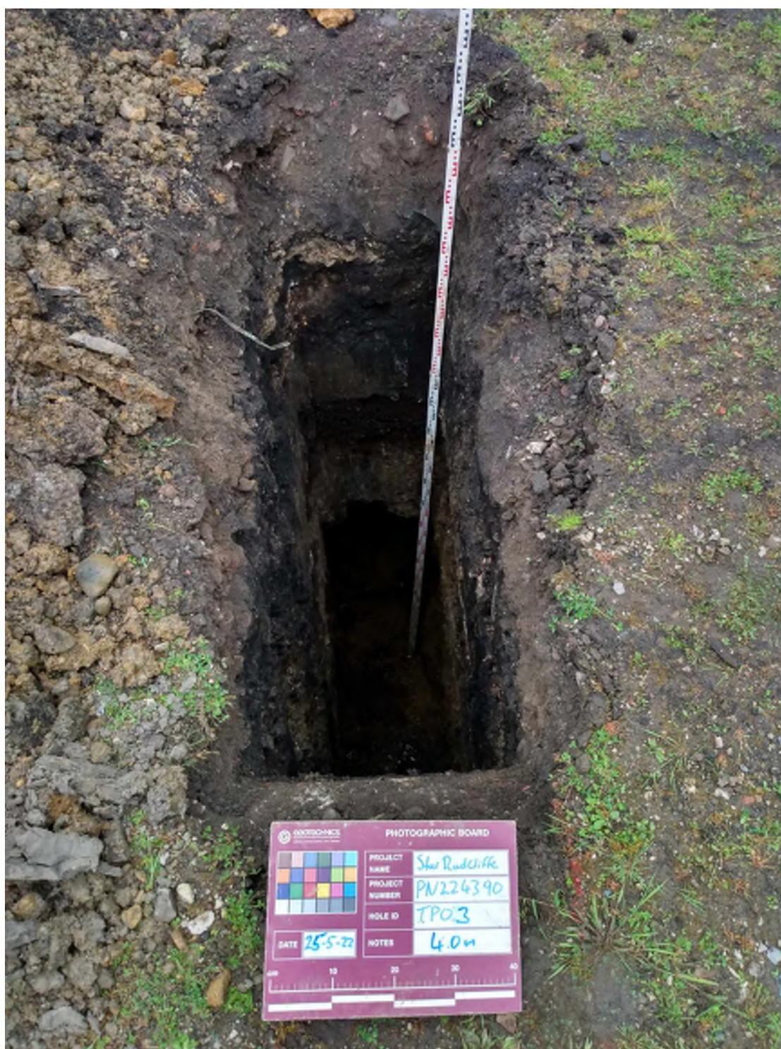
Machine-dug Trial Pit TP03 (I)
