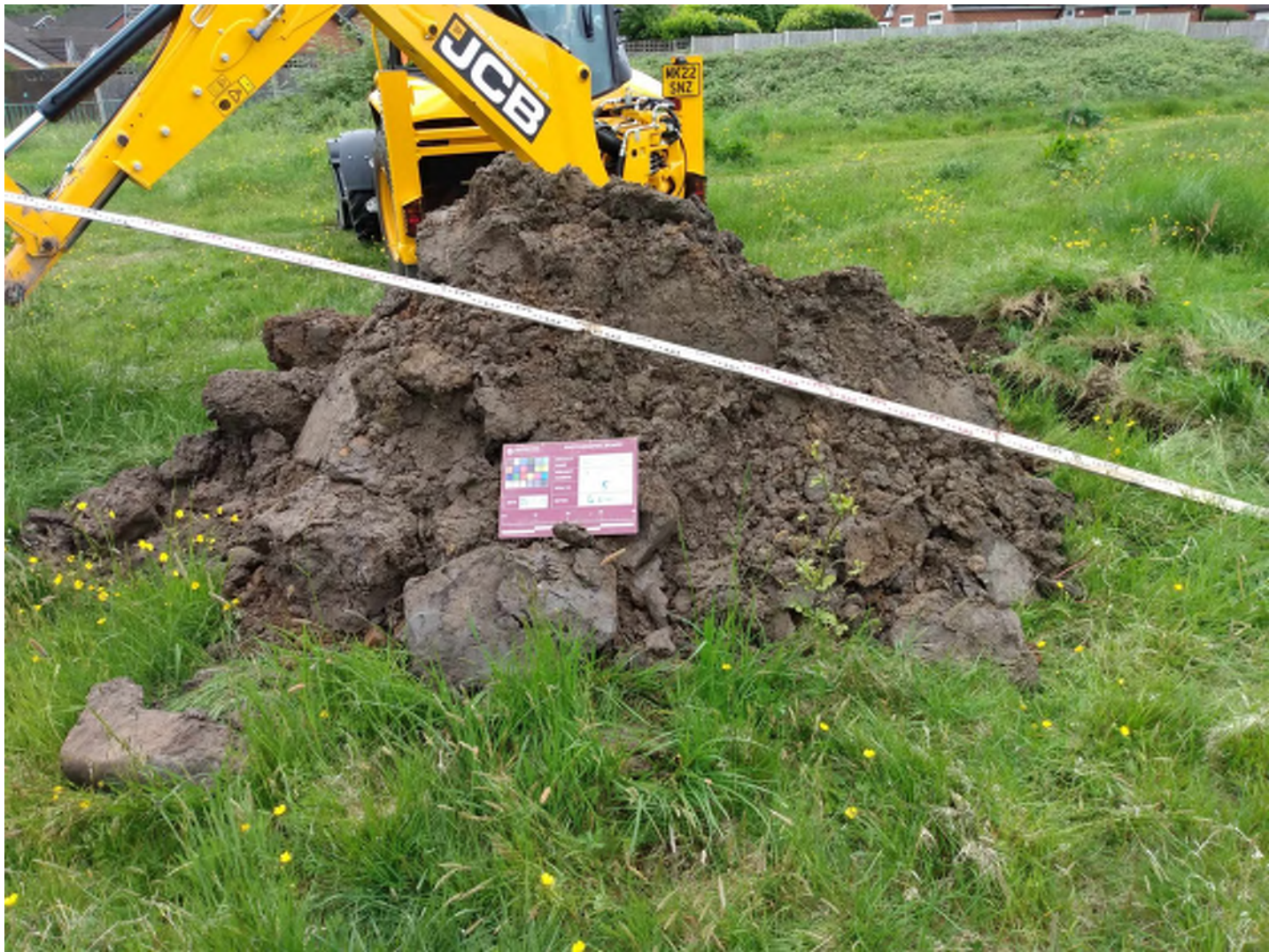
Machine-dug Trial Pit TP05 (3) Arisings
