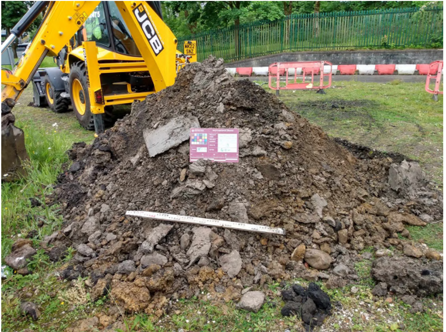
Machine-dug Trial Pit TP03 (3) Arisings
