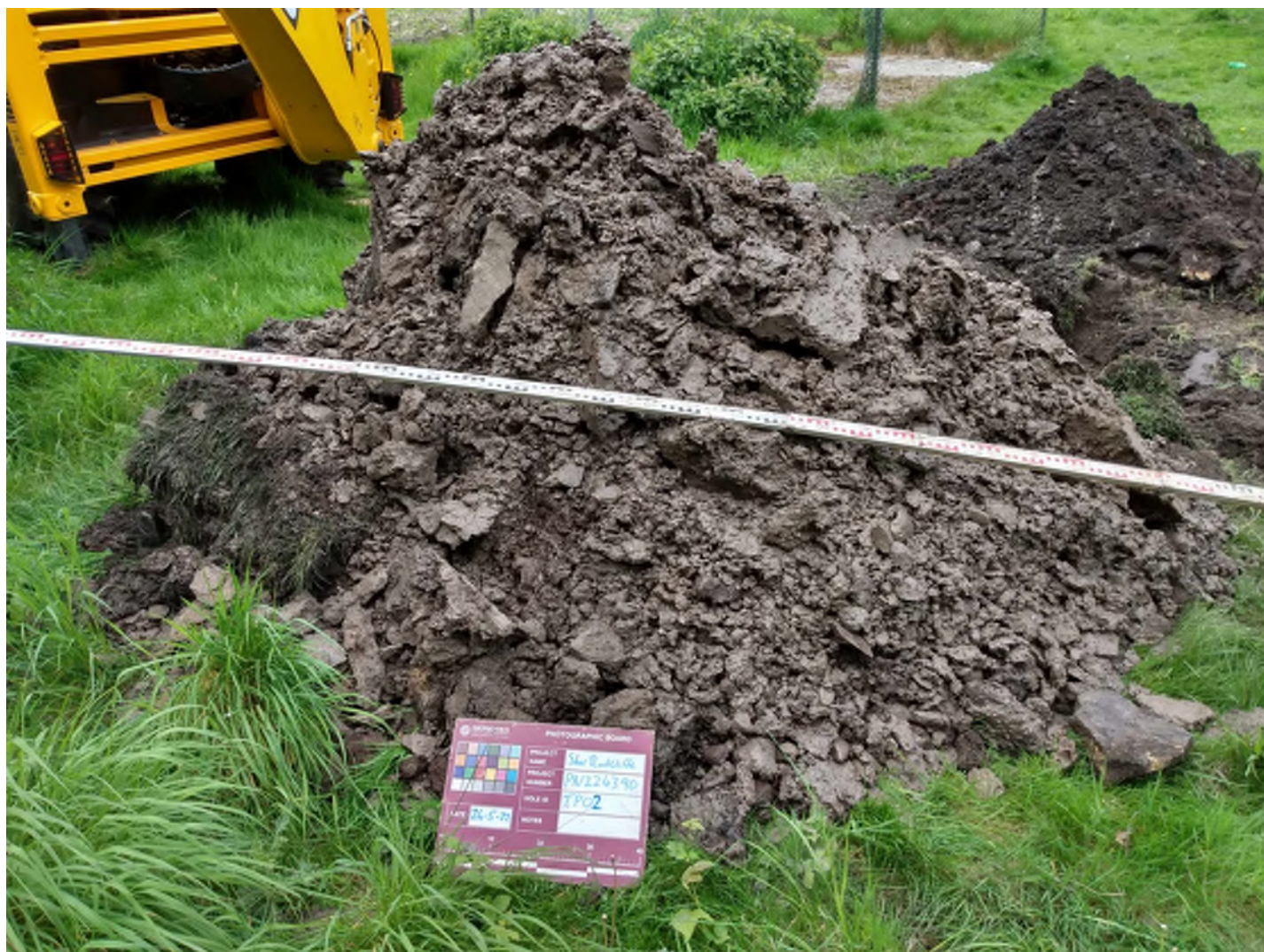
Machine-dug Trial Pit TP02 (5) Arisings
