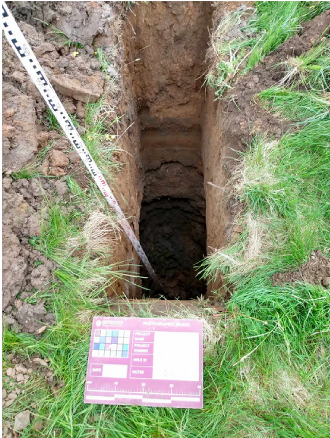
Machine-dug Trial Pit TP04 (I)
