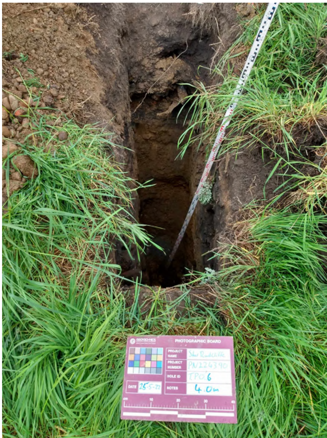
Machine-dug Trial Pit TP06 (I)
