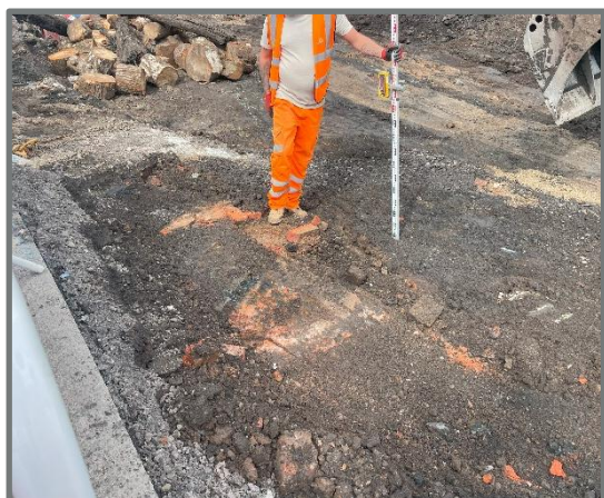
Check layer install using lazer level
