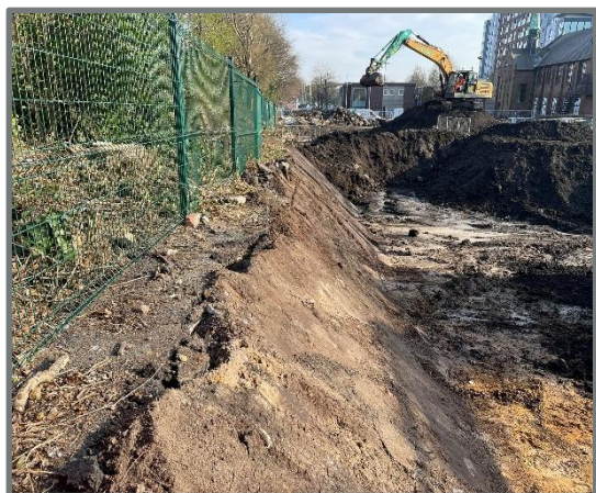
Battered sides of excavation
