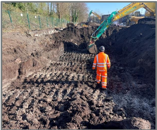
Base of excavation
