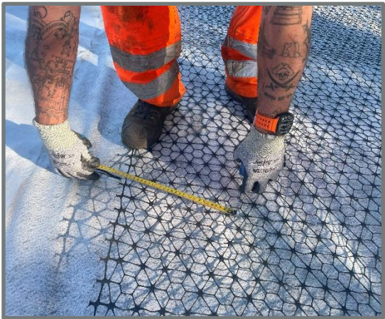
Geogrid and term install, 300mm overlay
