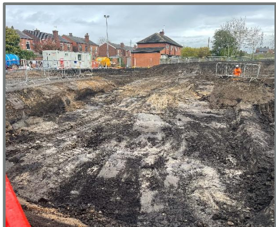
Base of excavation
