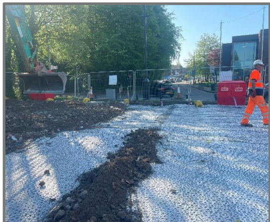
Geogrid and stone install
