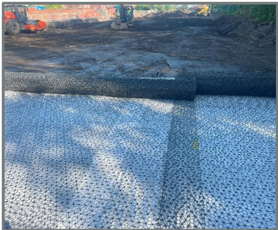
Geogrid and term install, 300mm
