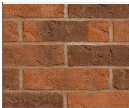
01. Brickwork (walls) Forterra 'Woodside Mixture' brick laid in stretcher bond with stone coloured mortar, bucket handle finish
