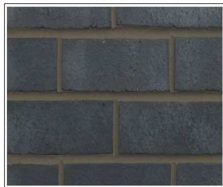
02. Brickwork (details) Forterra 'Blue Smooth' brick with stone coloured mortar, bucket handle finish
