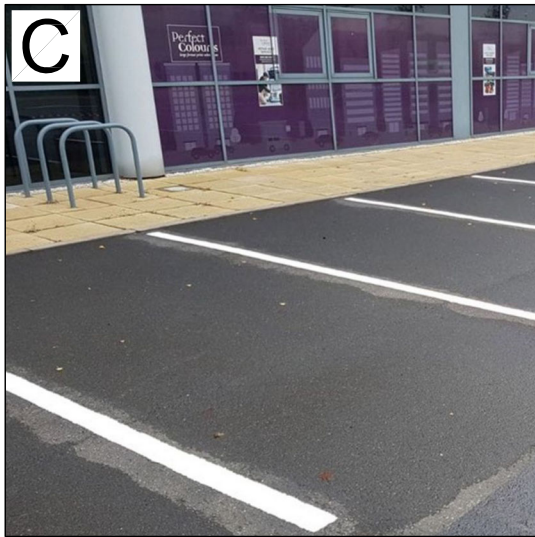
Tarmac with Resincoat car park line marking paint.
