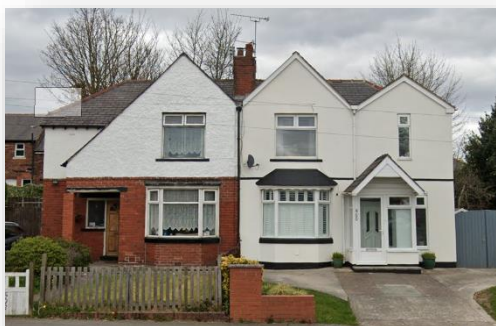
500 Bury Old Road Extension
