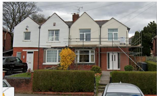
508 Bury Old Road Extension
