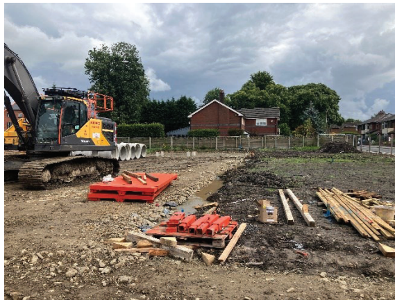
PLATE 2 GENERAL SITE OVERVIEW AND TEMPORARY WORKS PLATFORM
