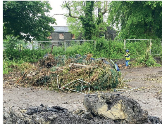
PLATE 10 SEGREGATED VEGETATION AND SCRAP MATERIALS
