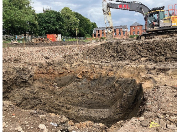
PLATE 8 SOFT CLAY ENCOUNTERED DURING DRAINAGE EXCAVATIONS
