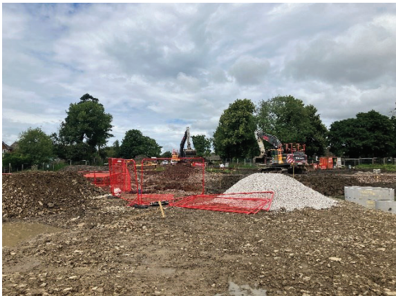
PLATE 3 GENERAL SITE OVERVIEW POST CLEARANCE
