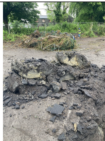
Trial Pit 203 Spoil
