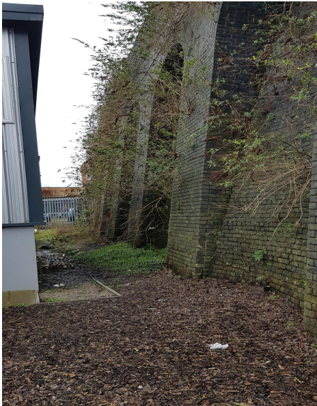
View of the current gap between the retail unit and the retaining wall. It is proposed that this will be enlarged to provide a drive-thru road.
