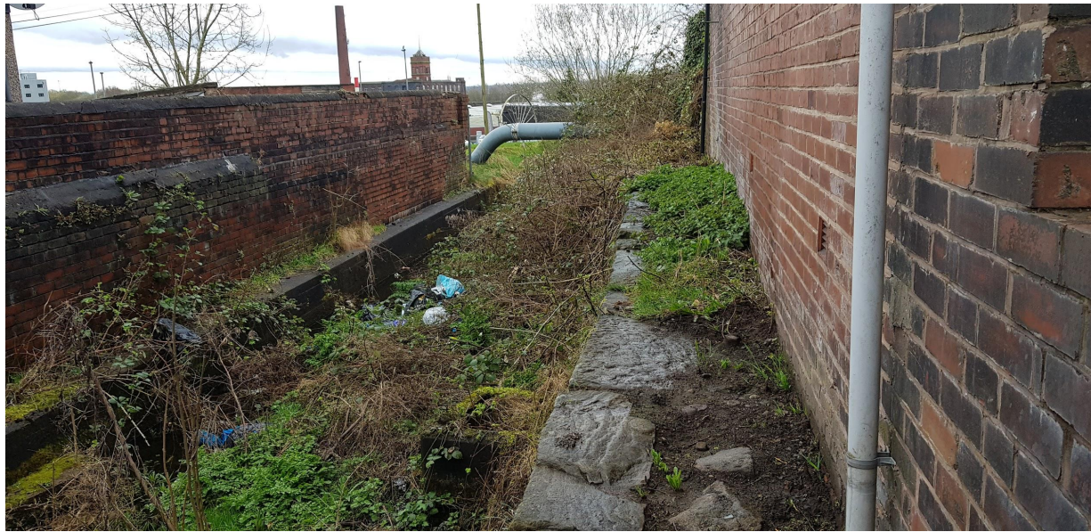
View of the feeder channel behind the top of the retaining wall.
