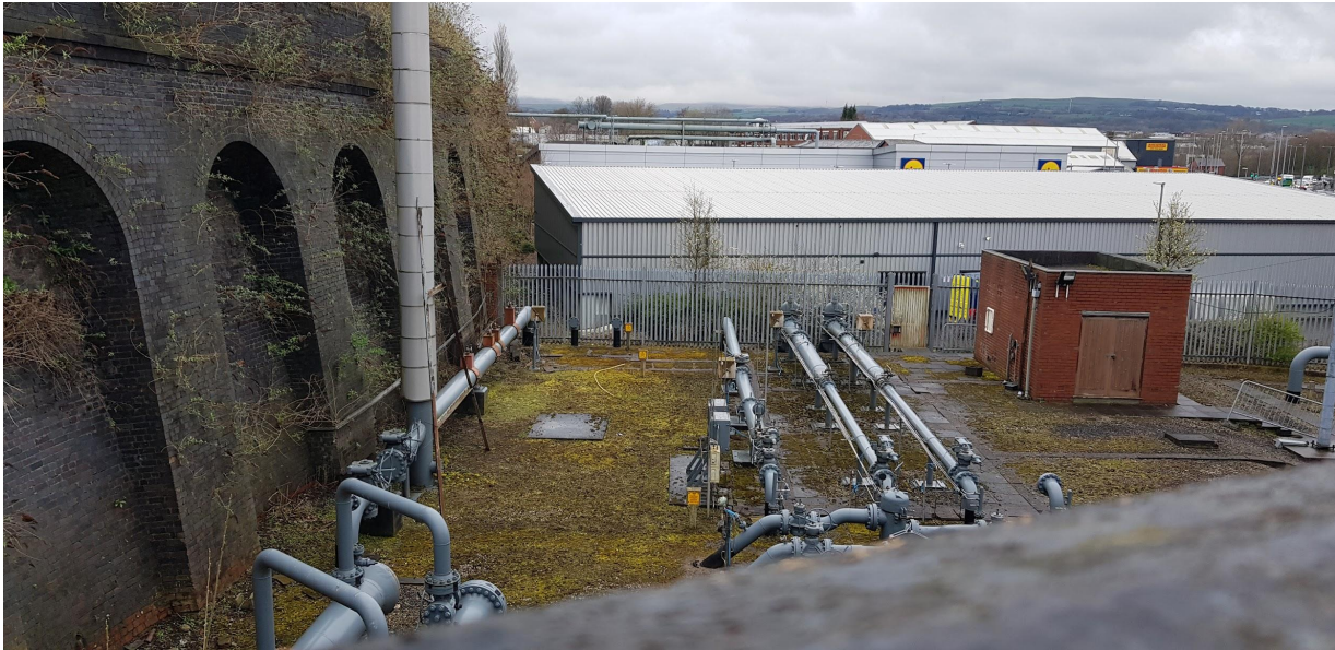
Rear view of the development location showing the gas infrastructure.
