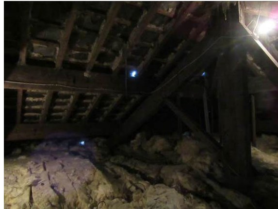
2016, prior to re-roofing
