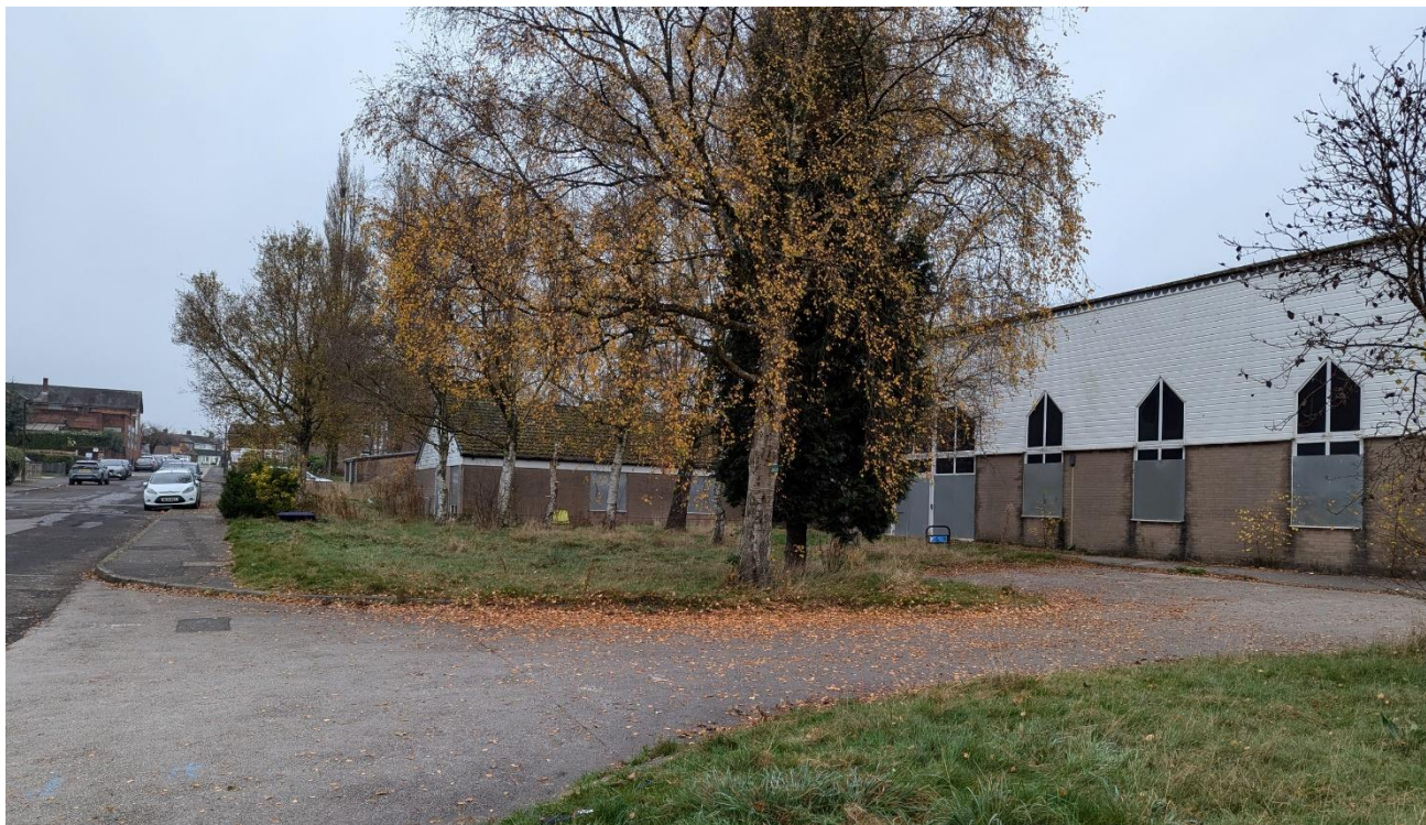
Figure 3 - Existing site access point and existing building on site
