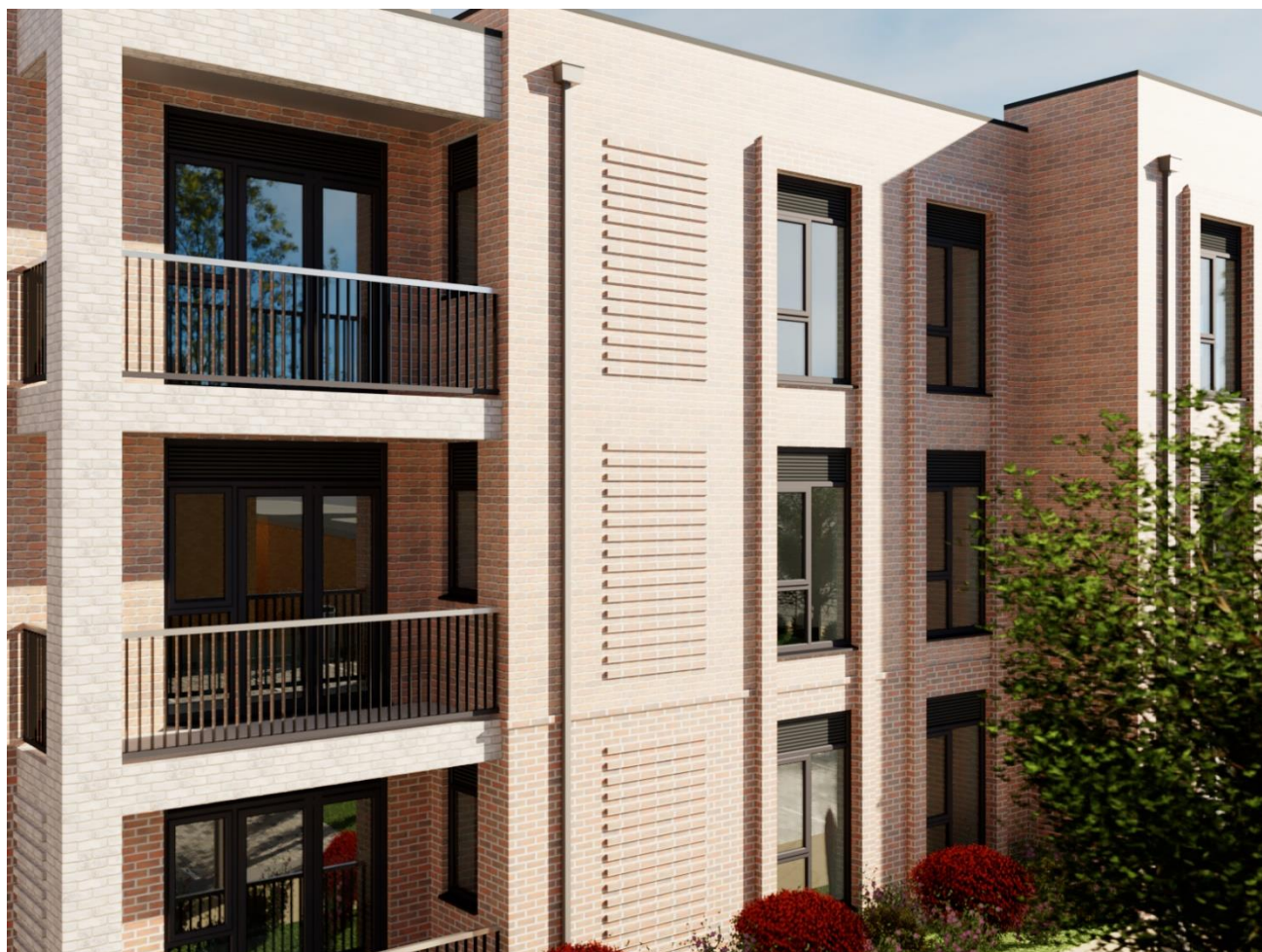
Figure 20 - CGI showing windows with integrated louvres
