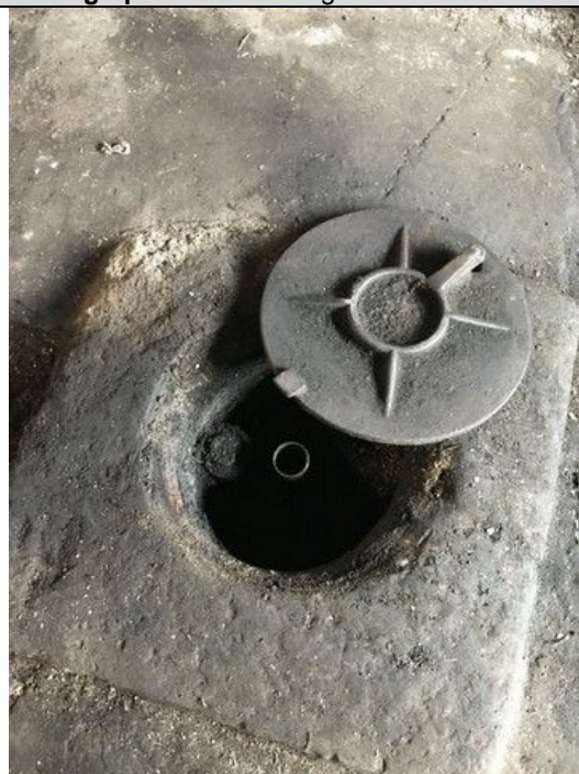
Photograph 5: Underground oil tank adjacent to inspection pit.
