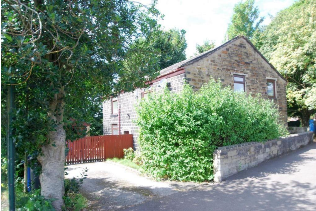
Figure 2: Photograph of existing property
