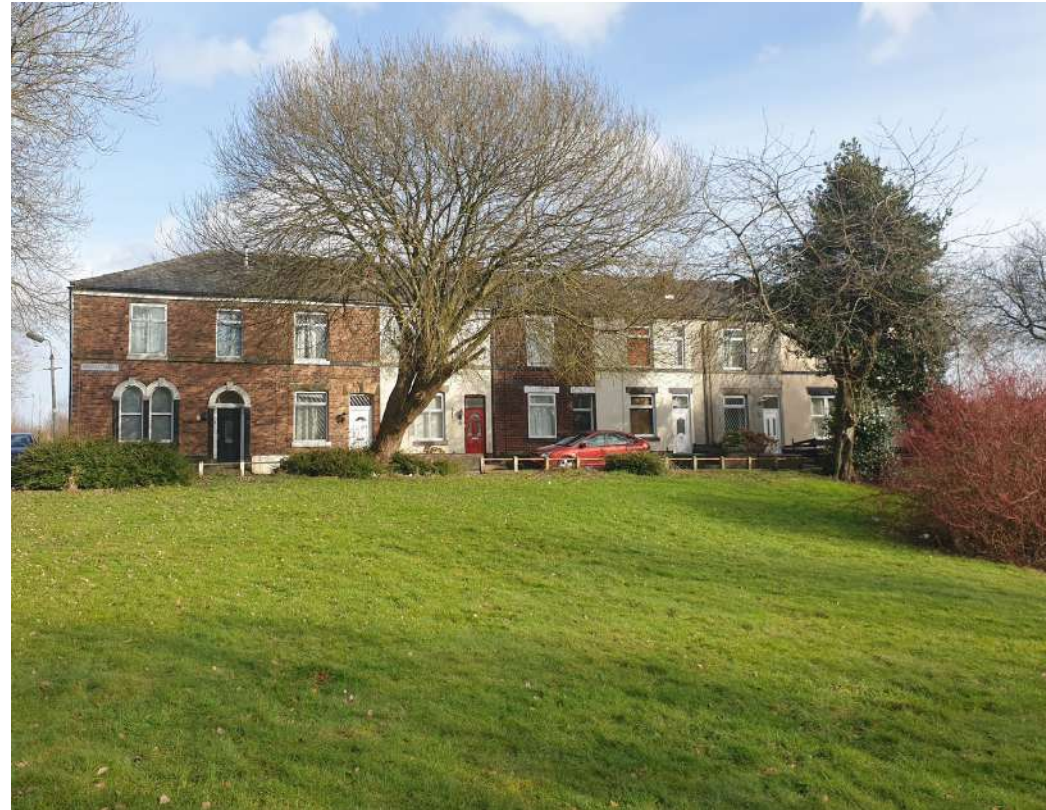
View looking North from grassed area
