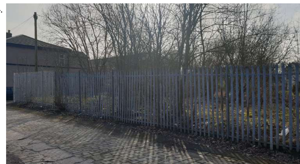
View Looking West into the site from Cock Clod Street
