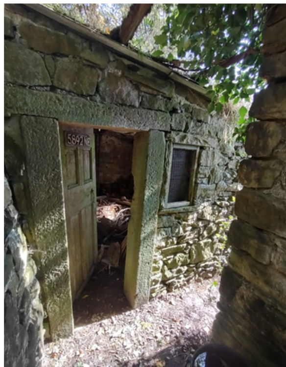
Existing outbuildings in elevated position adjacent to existing covered storage area
