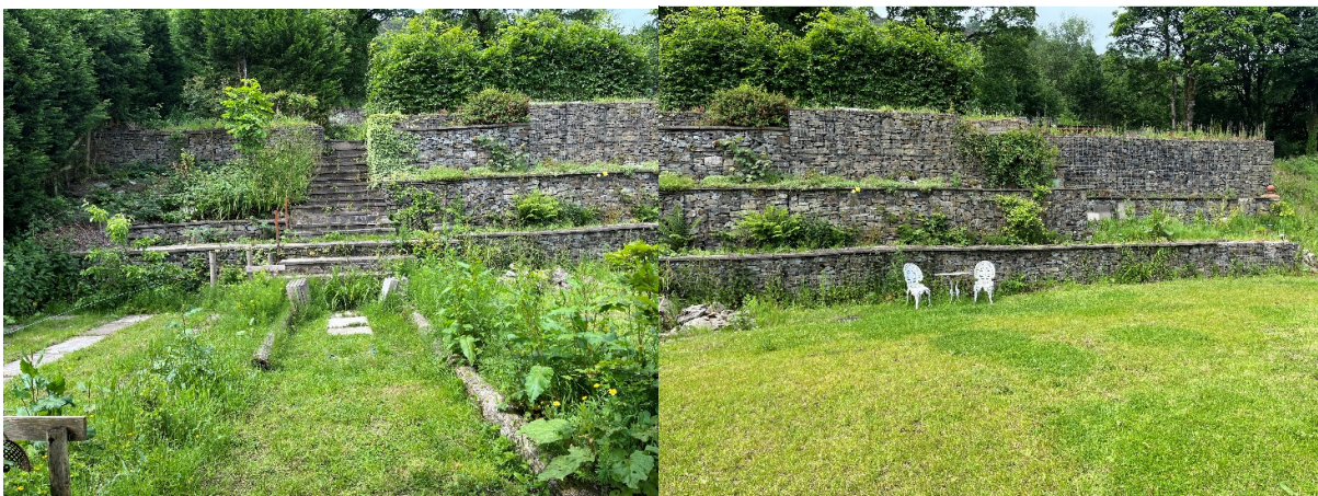
Random stones contained in gabion baskets form the retaining wall
