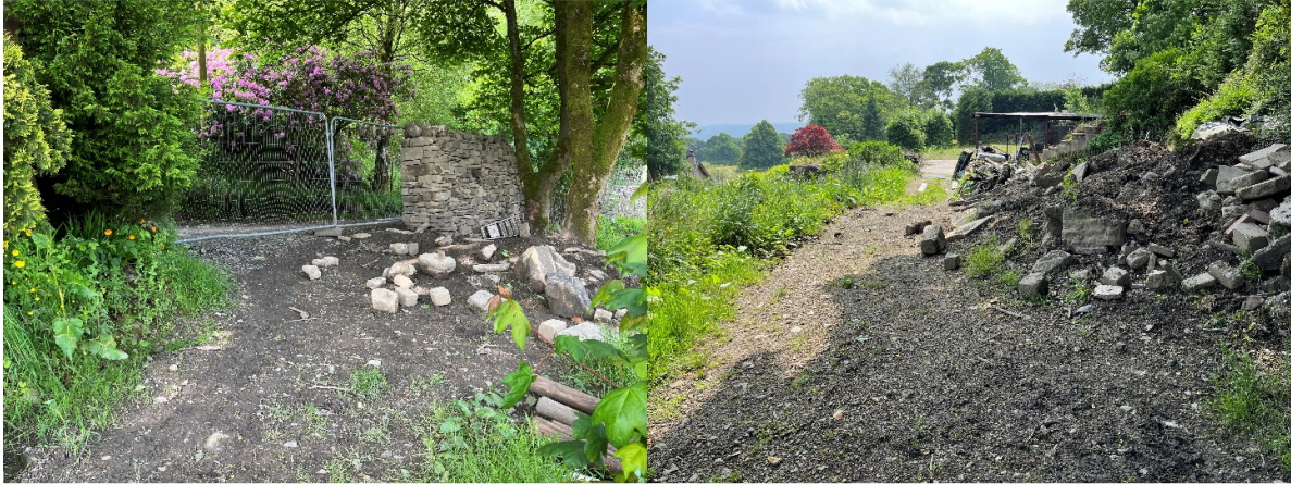
Entrance gate pillars leading from Moorbottom Road to the upper part of the site
