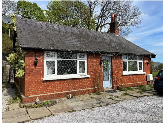
Front entrance elevation
