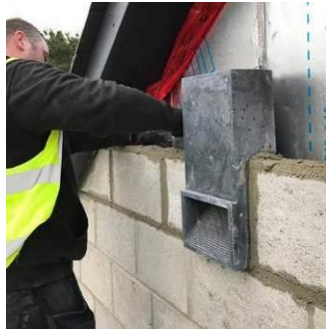
Green and Blue Bat Block/Brick in situ
