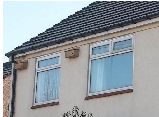
Wooden, wall-mounted swift nest boxes in situ
