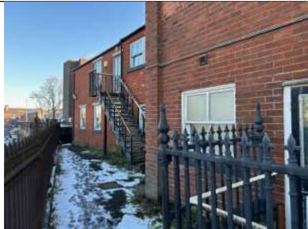
Image 02 – Gable elevation (apartment 1) Existing brick facings
