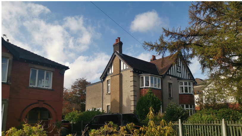
View of flat roof from road outside 22 Longsight Road
