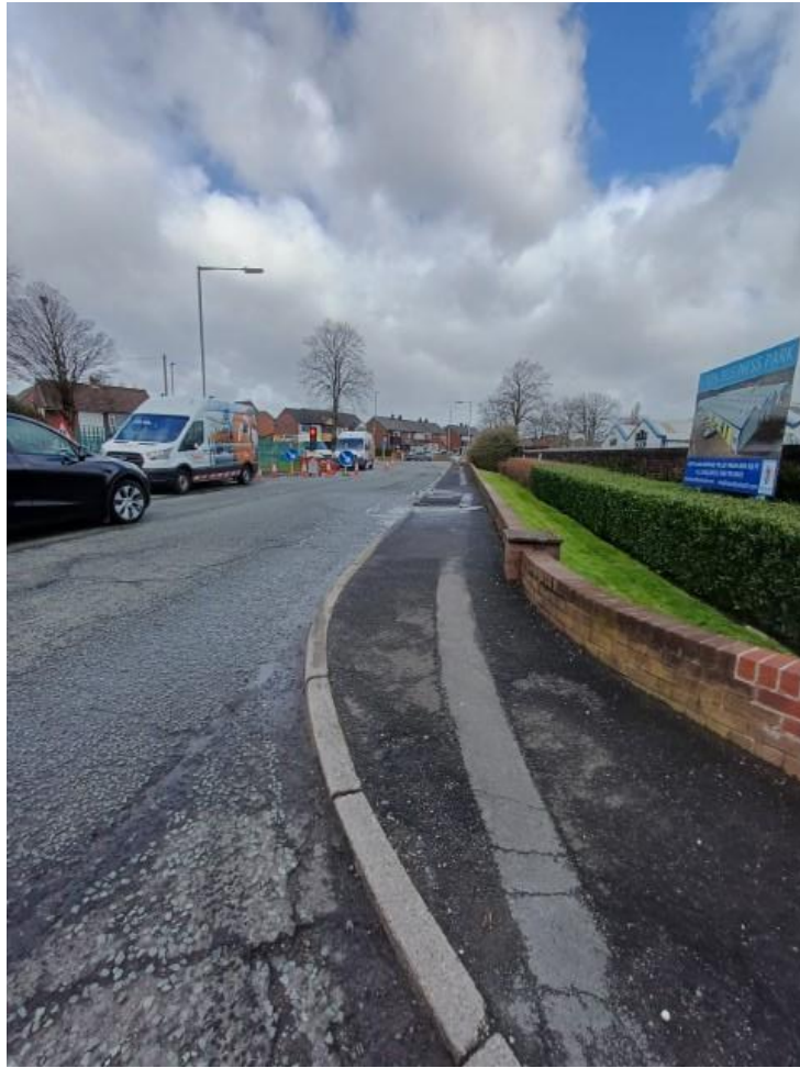
Entrance right (Cadent working on Eton Hill Road)
