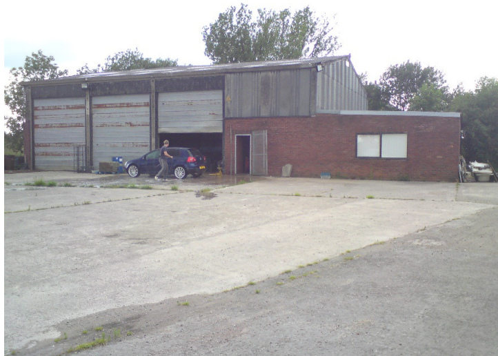
Existing office block and workshop currently standing between the proposed location of our static caravans and the listed Brick House Farm
