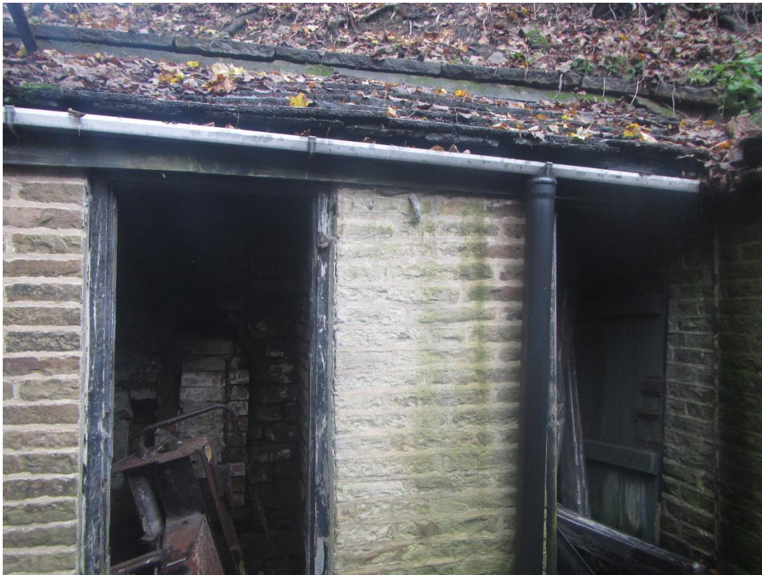
Photograph 15 – Eastern aspect of Building 4.
