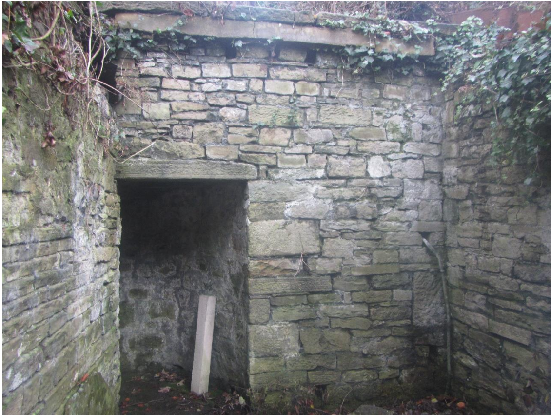
Photograph 13 – Eastern aspect of Building 3.
