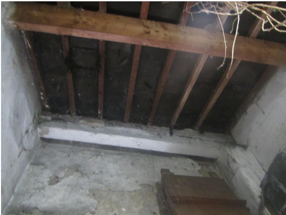
Photograph 24 – Internal view of roof within Section B of Building 2.
