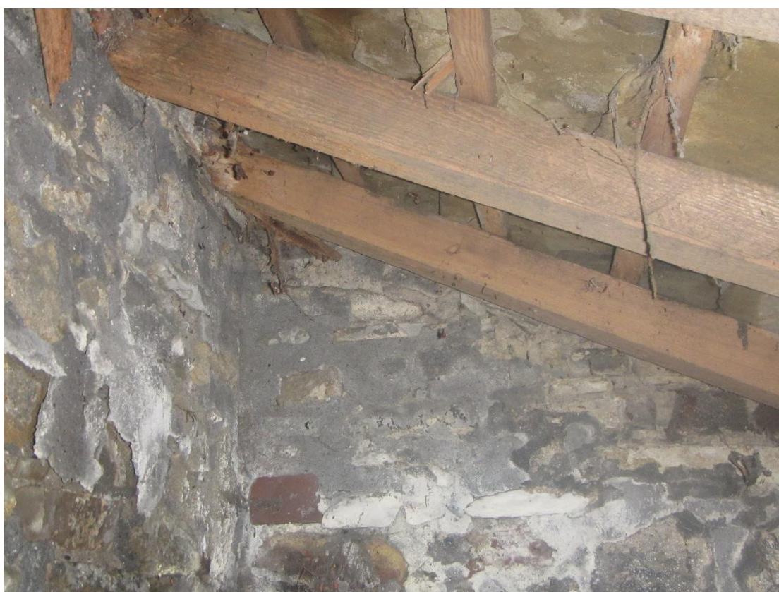
Photograph 18 – Internal view of Building 1.
