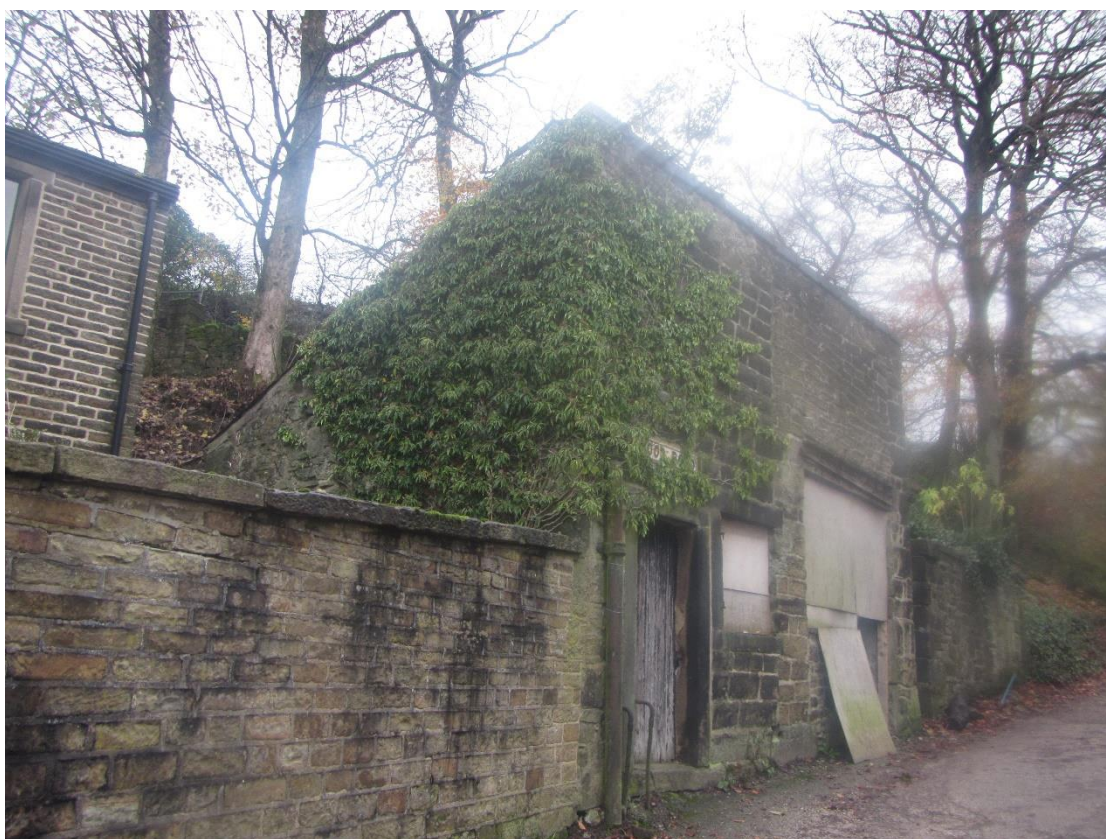
Photograph 4 – South-eastern aspect of Building 2.
