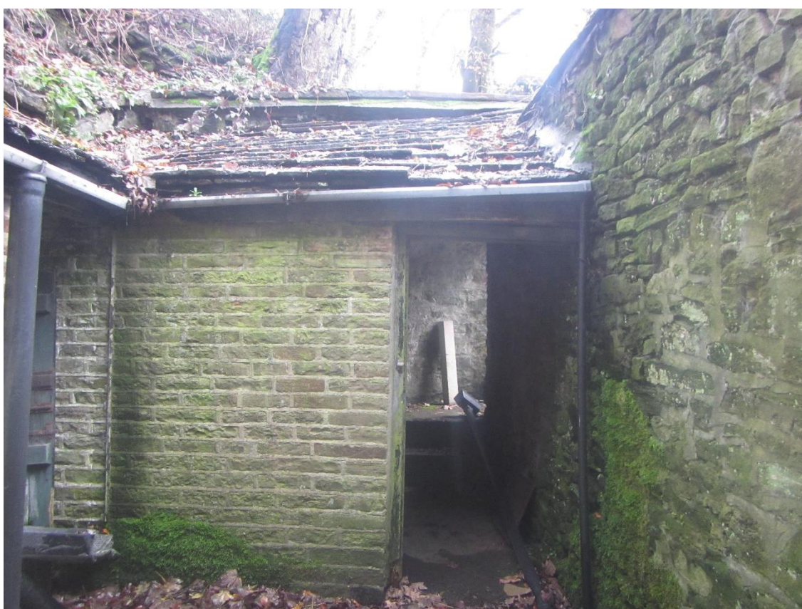
Photograph 12 – Southern aspect of Building 3.
