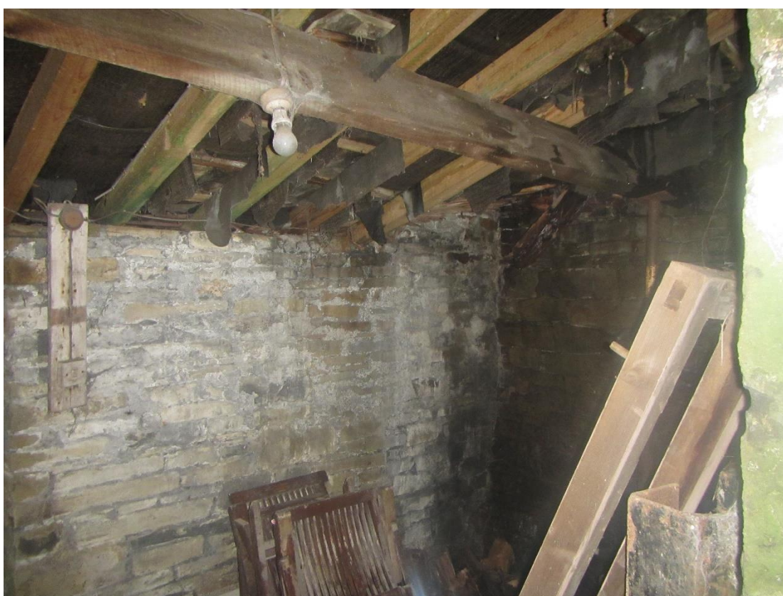
Photograph 28 – Internal view within Building 3.
