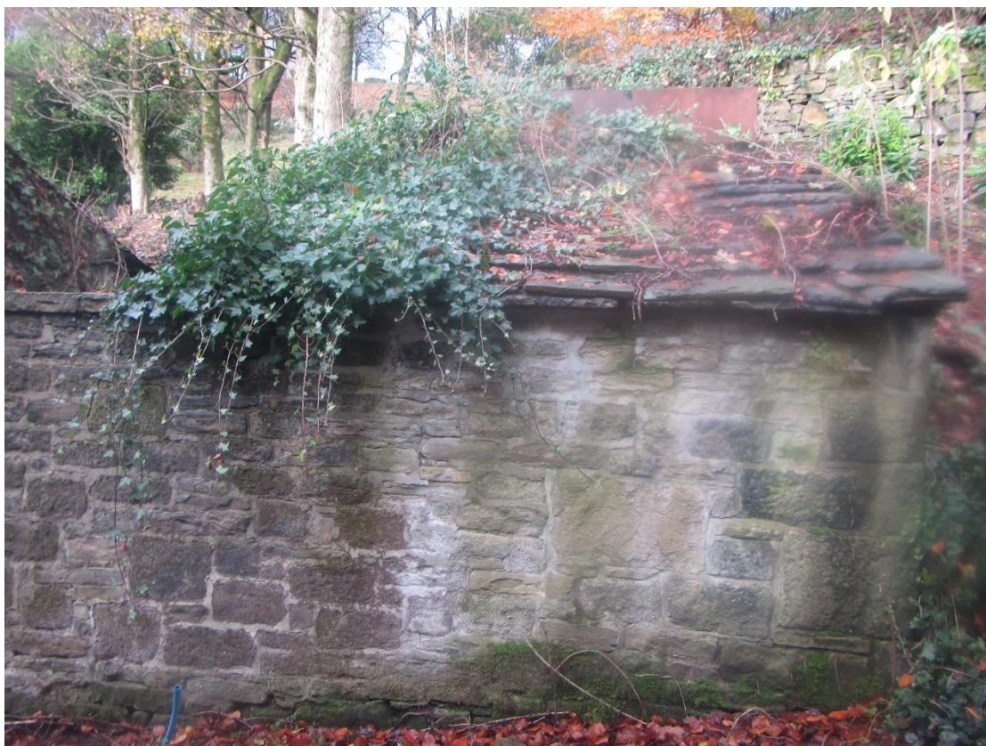
Photograph 2 – The eastern aspect of Building 1.
