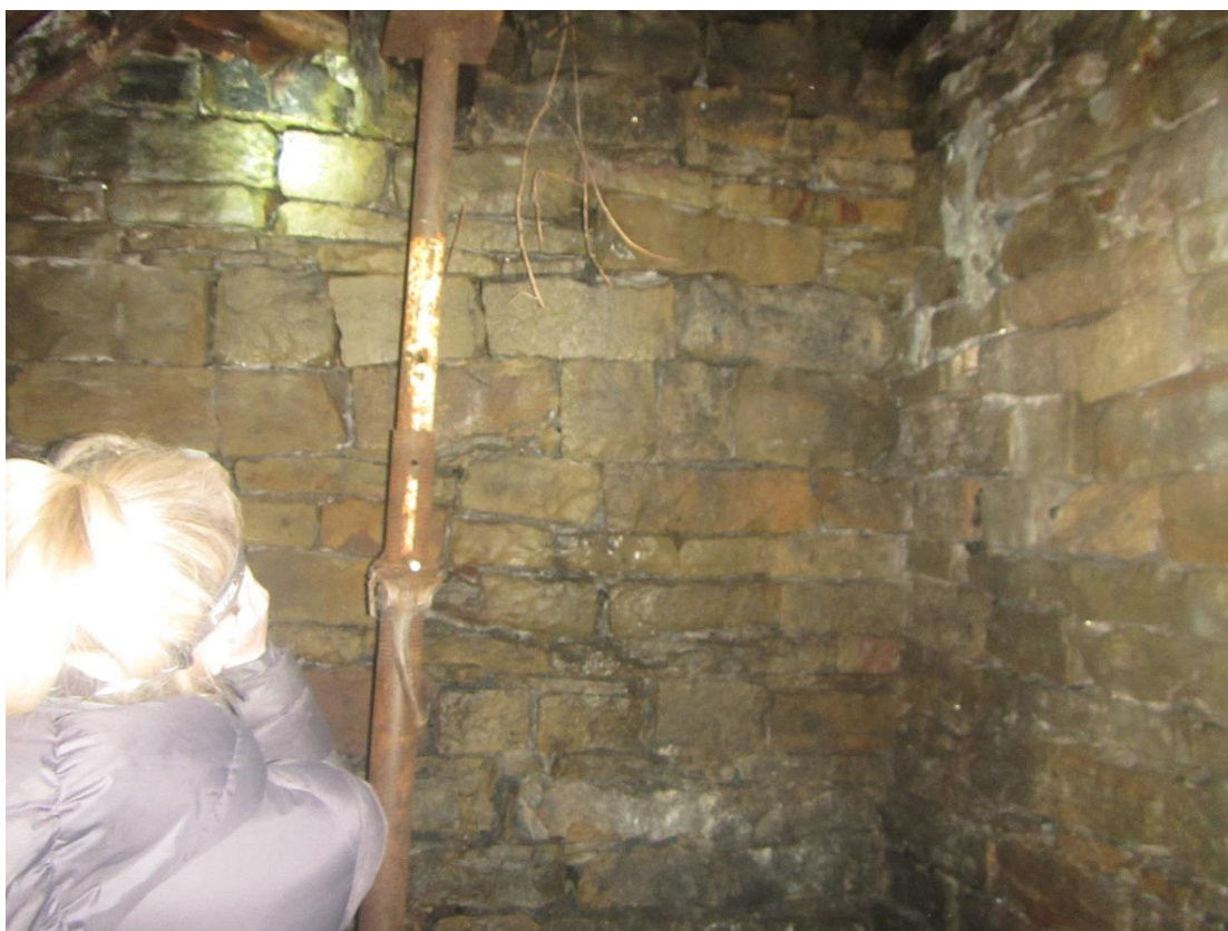
Photograph 27 – View of steel support within Building 3.
