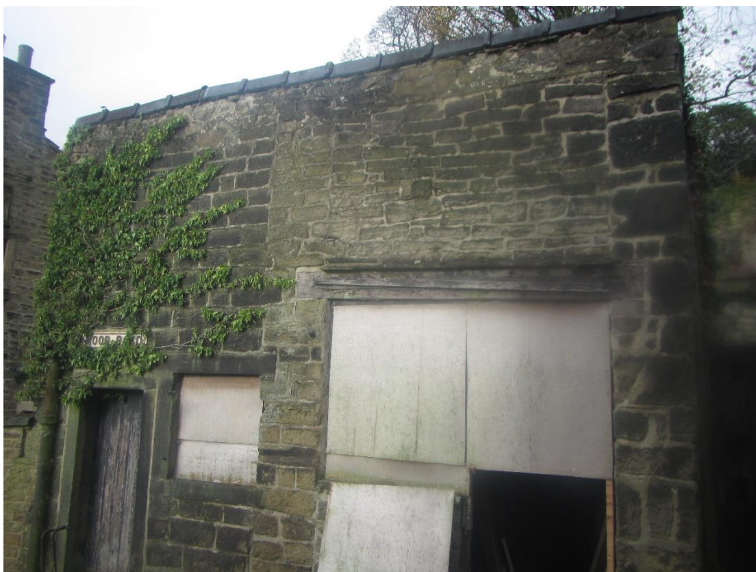
Photograph 5 – Eastern aspect of Building 2.
