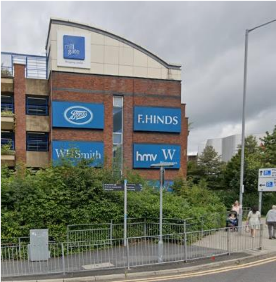
Prominent advertisement display at the multi-storey car park to the north
