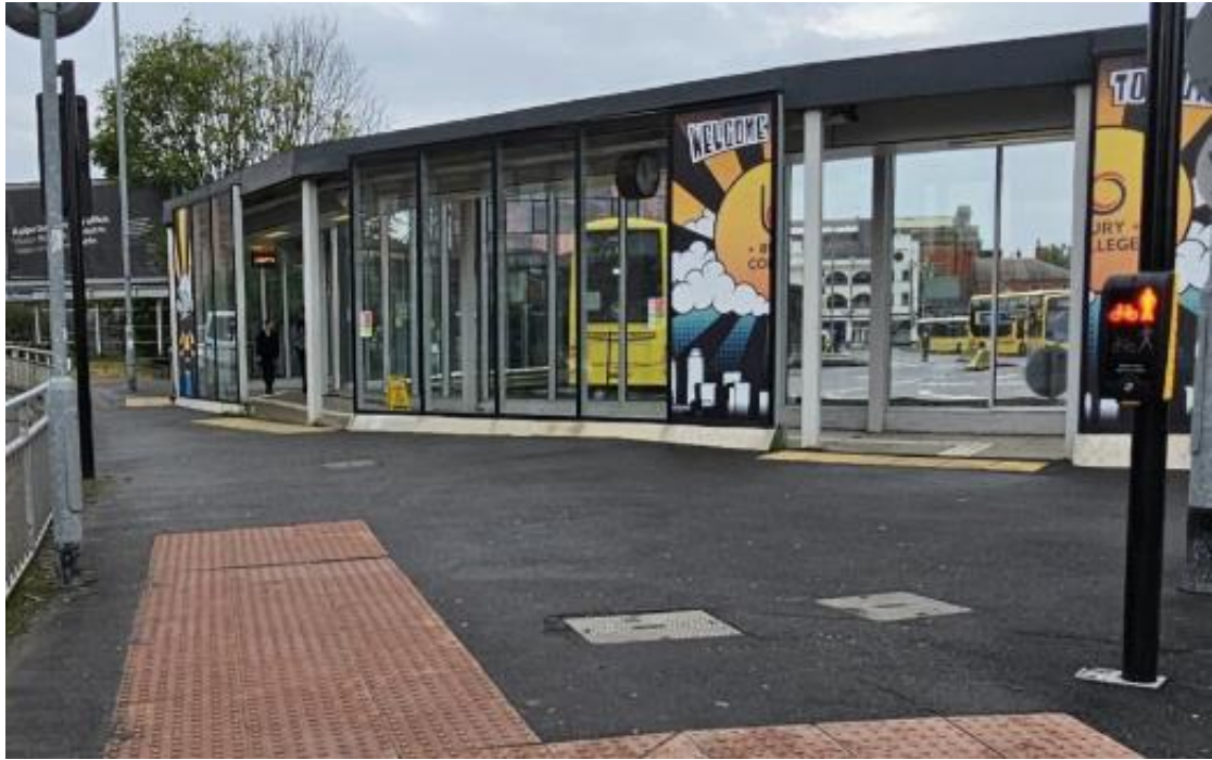
Street view of site
