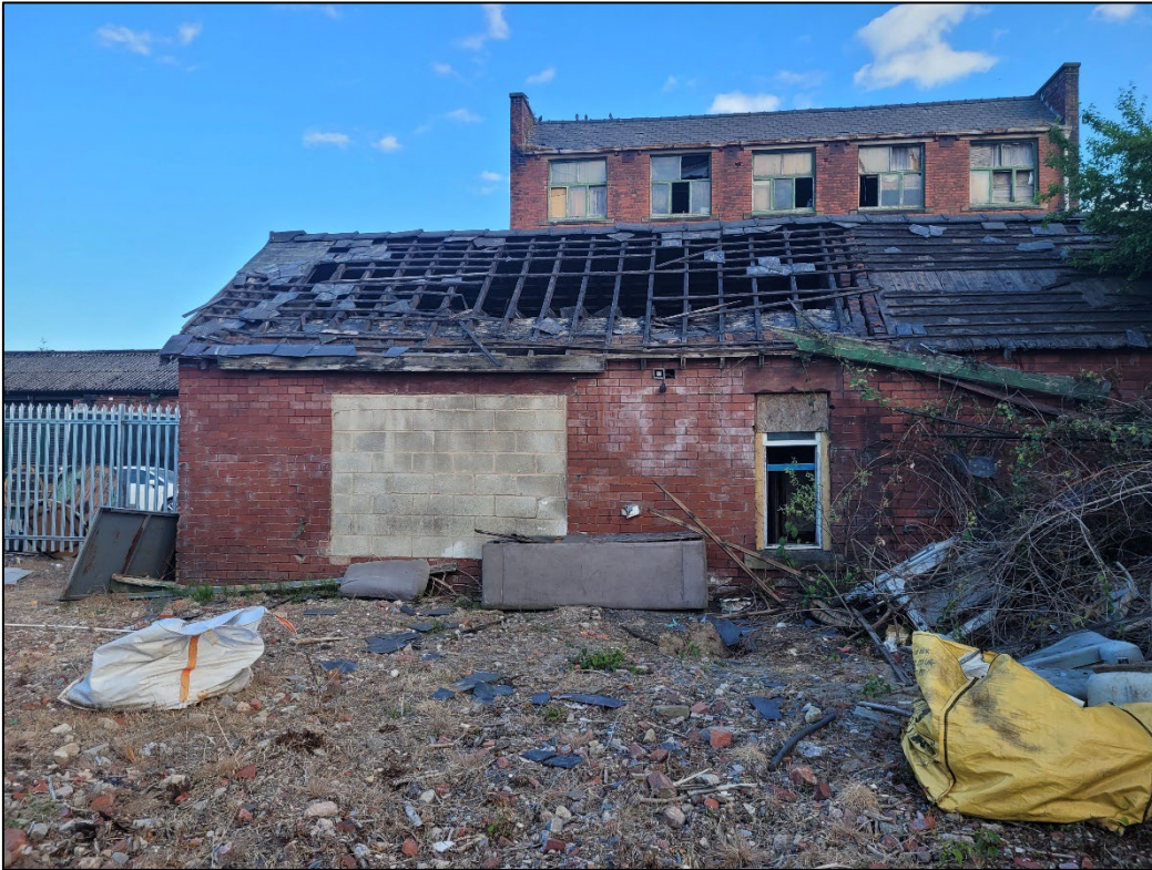
Photograph 1 Single-storey red brick-built outbuilding
