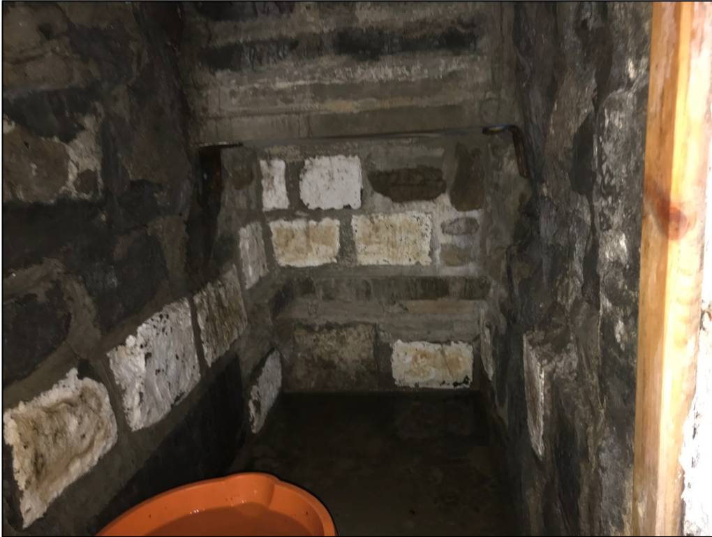
4.3 Modern niche within cellar. This would be concealed on completion of the tanking scheme.
