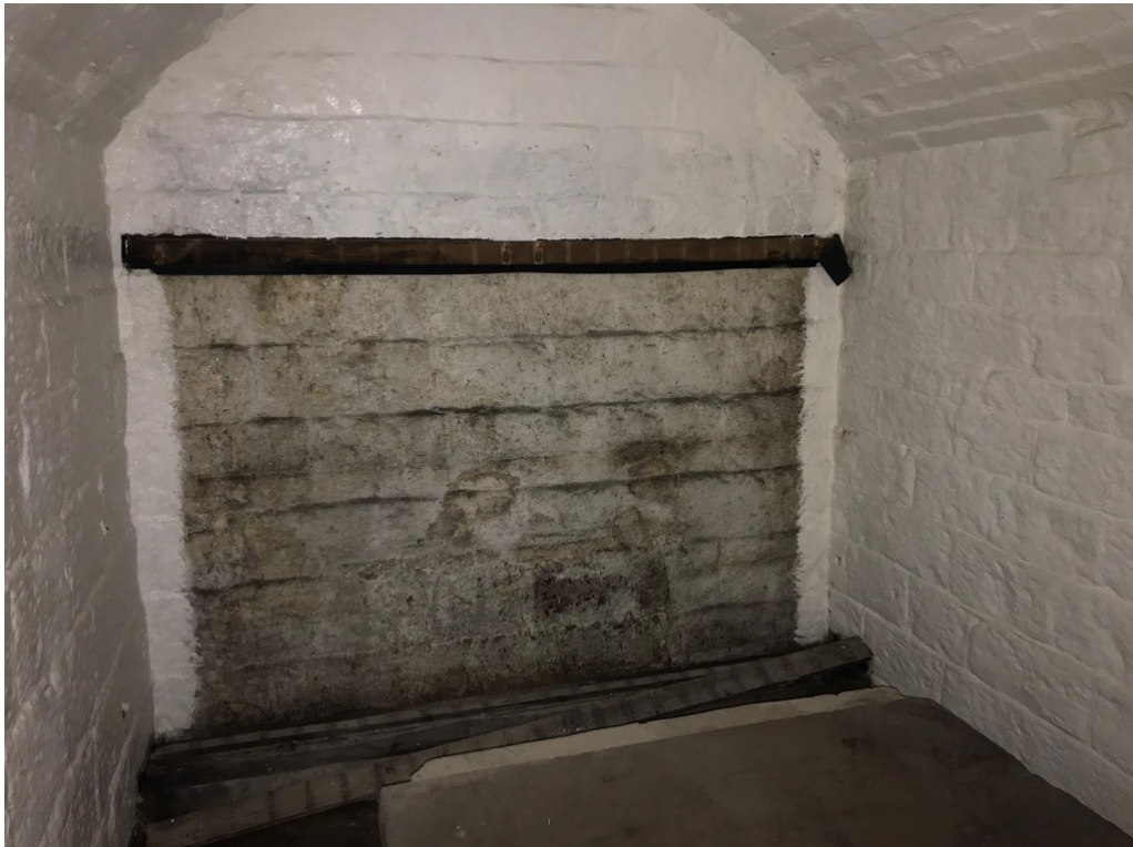
4.2 Partially historic stonework within cellar walls proposed for tanking system.
