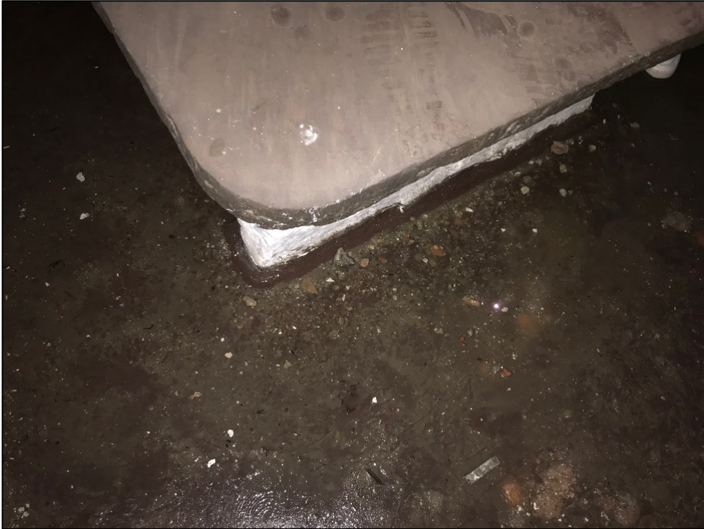
4.1 Stone table within cellar, proposed for removal under a scheme of membrane tanking.
