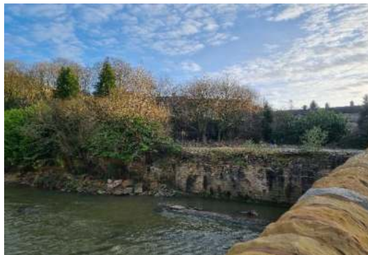
View of Site from bridge over River Irwell
