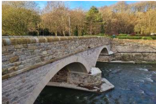
View of bridge over River Irwell
