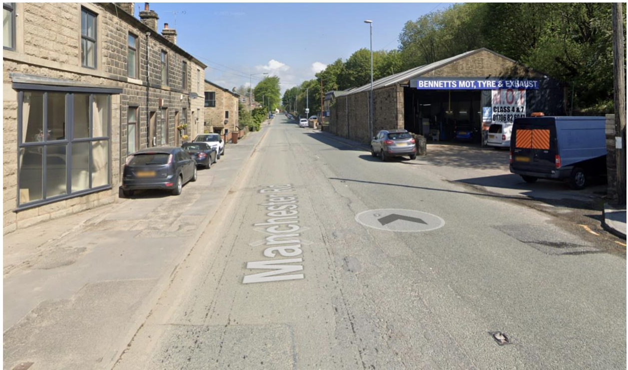
A view looking north along Manchester Road.
