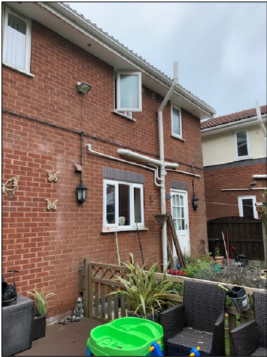
04 EXISTING REAR ELEVATION 001 photo
