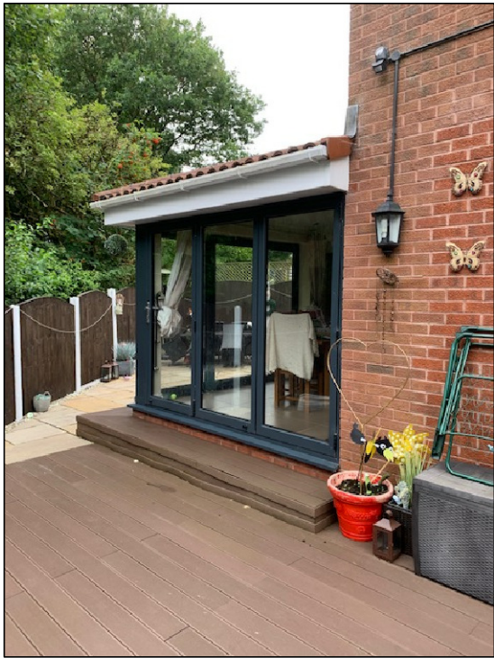
03 EXISTING REAR EXTENSION 001 photo
