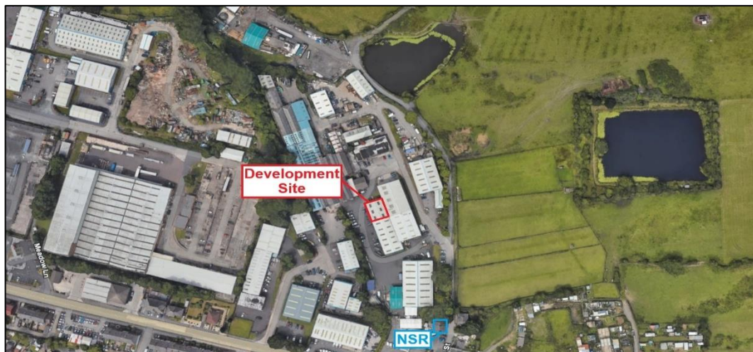
Figure 1: Development site aerial photograph.
