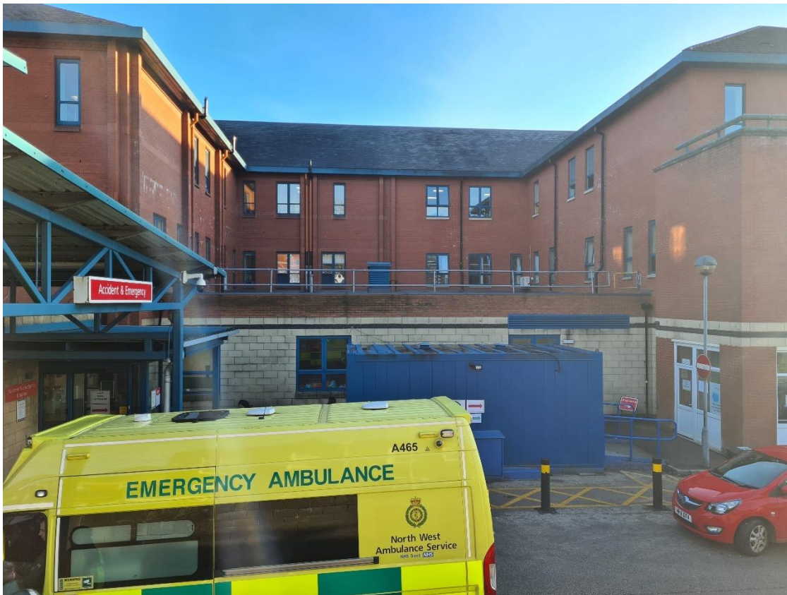
Figure 1 showing the front of the existing site area.
