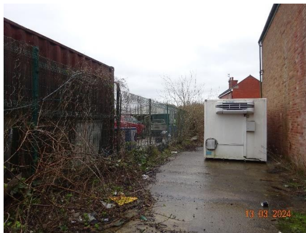
Pic 11 shows the view looking east along the northern perimeter of the proposed development site. The proposal is to demolish the brick building adjacent to the white container on the right of the picture.
